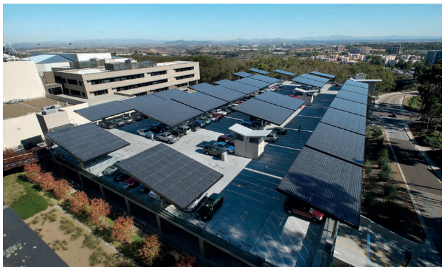
9.8 Solar Tree® array by Envision Solar
