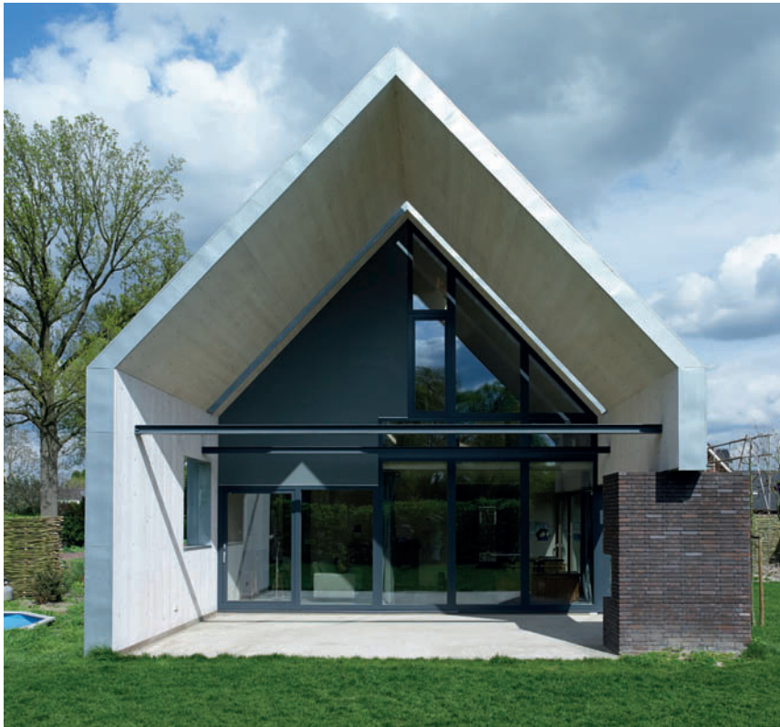
4.1 Direct daylight reflected indoors via the ground, walls, and roof Source: Passivhaus Witven © Architect: Thomas Kemme Architekten; Photography Ruud Peijnenburg
