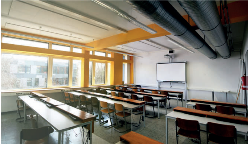
12.11 Computer room after the refurbishment
