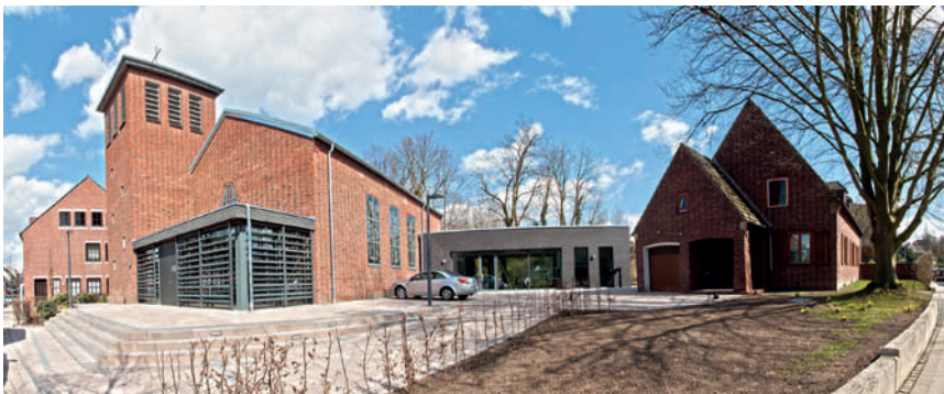
12.2 View (front) of the church after the refurbishment
