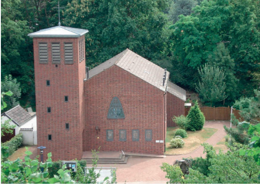
12.1 Church (Christuskirche) in Heinsberg, Germany before the refurbishment took place
