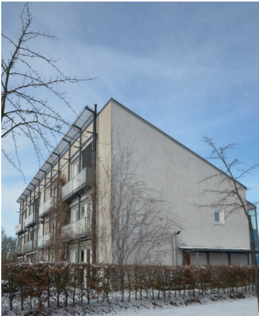
1.3 First Passivhaus in Kranichstein close to Darmstadt, Germany
