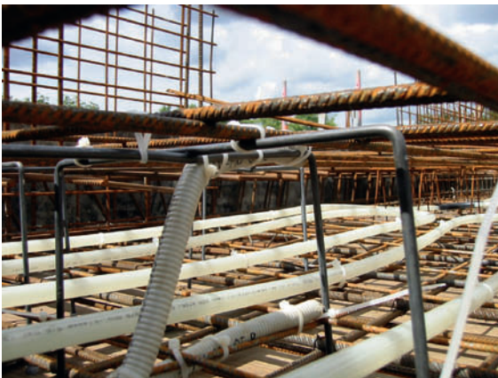
76 Thermo-active building systems: (left) pipe circuit between upper and lower reinforcement, (right) floor area with pipe circuits, and connection at ceiling for TABS Source: Fraunhofer ISE
