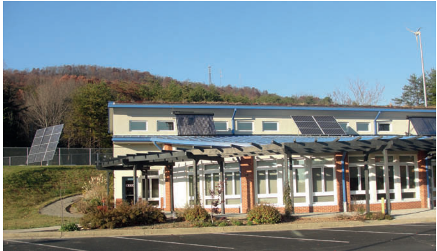
9.17 The Centre for Energy Efficient Design Source: © James Madison University
