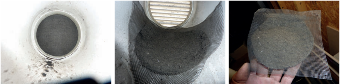
Fly screen installed on supply air terminal totally blocked with fibrous material.
