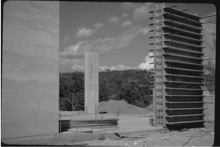
14.6 Concrete posts and bond beam yet to be poured.
