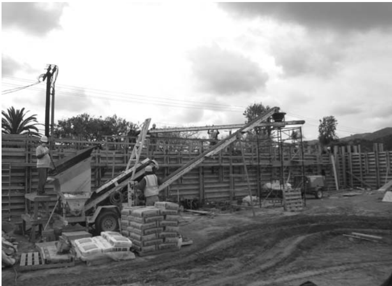
14.4 Installation using conveyor delivery.
