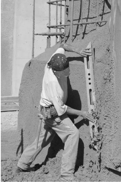
15.6 PISE being rodded (finished).
