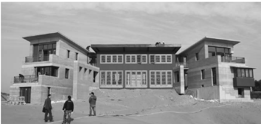
24.5 River house – main house: multi-storey stabilized insulated rammed earth.
