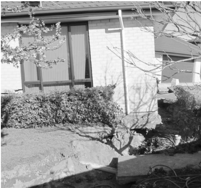
19.34 Major ground disruption around a house due to lateral spreading initiated by liquefaction. Not an earth house – timber frame with fired brick masonry veneer (photo: M. Pender).
