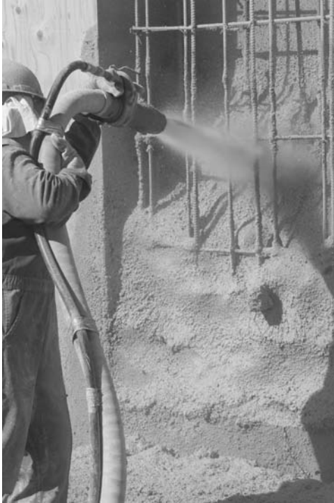
15.1 PISE being installed.
