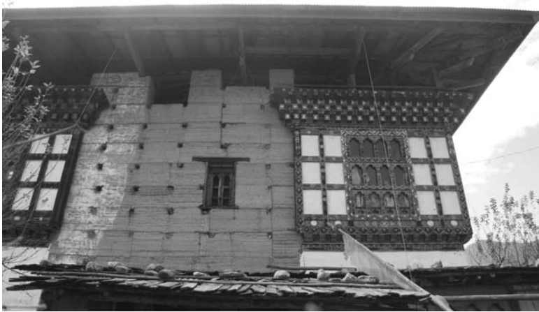
12.1 Rammed earth section of Kyichu Lhakhang Monastery, Bhutan.
