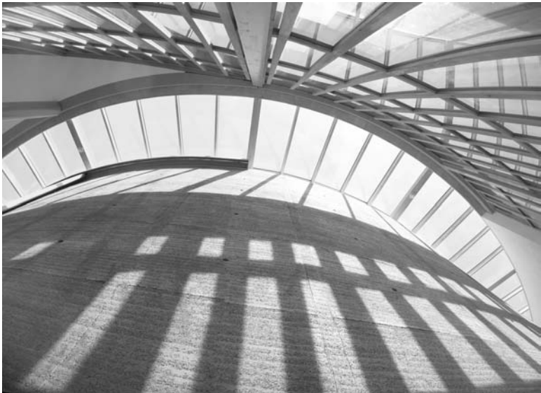
23.29 Load-bearing, curved unstabilised rammed earth walls forming the structure of the WISE Lecture Theatre, Centre for Alternative Technology (CAT), Wales (© Pat Borer, 2011).
