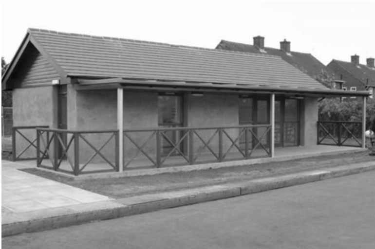
23.25 Brimington bowls pavilion, built in just 21.5 hours including the 17.5 m 3 of load-bearing stabilised rammed earth walls and the timber truss roof structure plus roof covering (© M R Hall, 2003).
