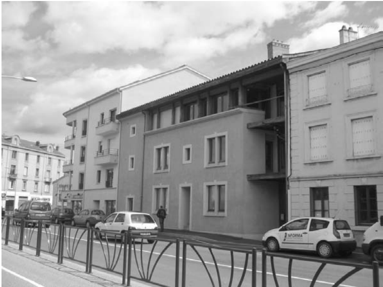
23.19 Completed 9.4-m-high unstabilised earth wall building at Montbrison, Loire with external render and traditional appearance (© Nicolas Meunier, 2011).
