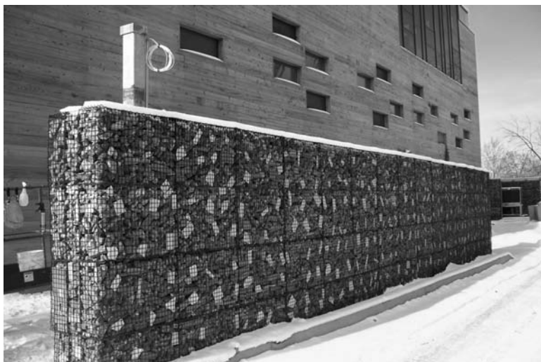
7.3 Wall made of coarse compacted demolition waste in gabions (photo reproduced by kind permission of www.gabionbaskets.net ).
