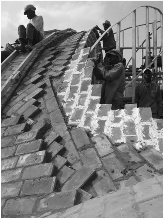
17.13 Mapungubwe Interpretation Center under construction (photo: James Bellamy).
