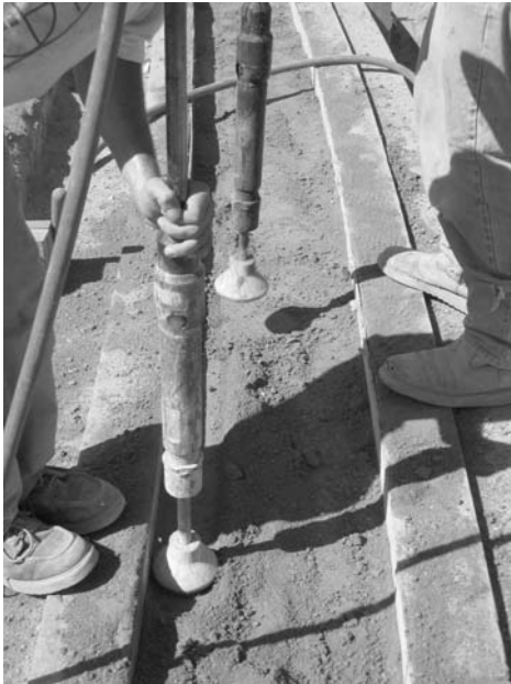
14.7 Pneumatic compaction at the top of a rammed earth wall.
