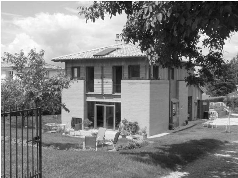
23.21 Completed house at Chasselay with rammed earth corner walls to provide thermal buffering, and lightweight timber frame upper floor construction with increased glazing area to allow direct solar gain (© Nicolas Meunier, 2011).
