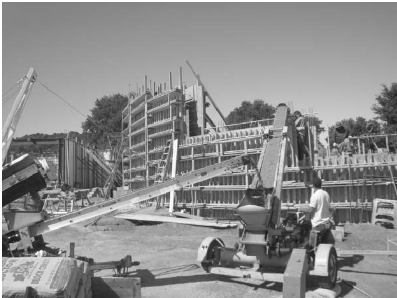
14.5 Installation using conveyor delivery.
