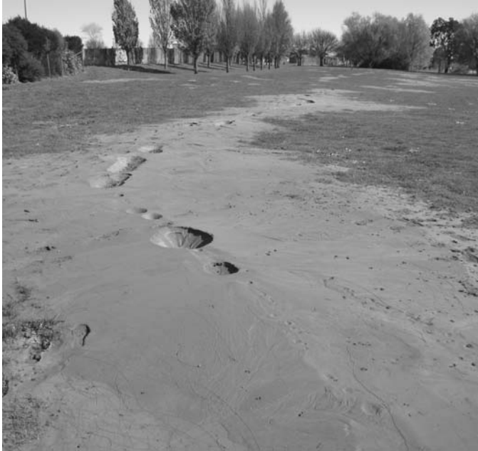
19.33 Sandboils due to ground liquefaction in New Zealand (photo: M. Pender).
