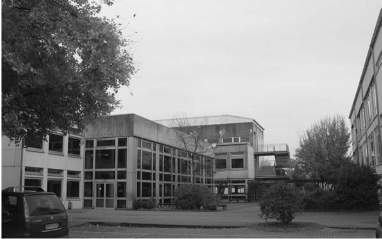
5.32 Construction phases 3 and 4 of the school buildings before refurbishment. Photo courtesy of Rongen Architects GmbH.
