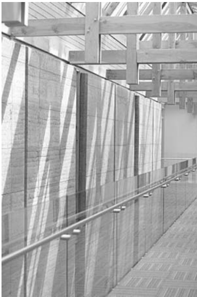
23.14 Timber wall plate and roof truss connection on the 6-m unstabilised rammed earth wall at the Rivergreen centre, Aykley Heads, UK (© Rivergreen Developments Plc – Developer/Contractor, photograph by Allan Mushen, 2006).
