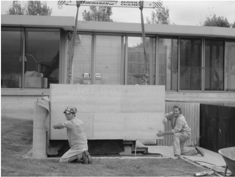
22.19 Placing an elevated SRE panel. Flinders, Victoria.
