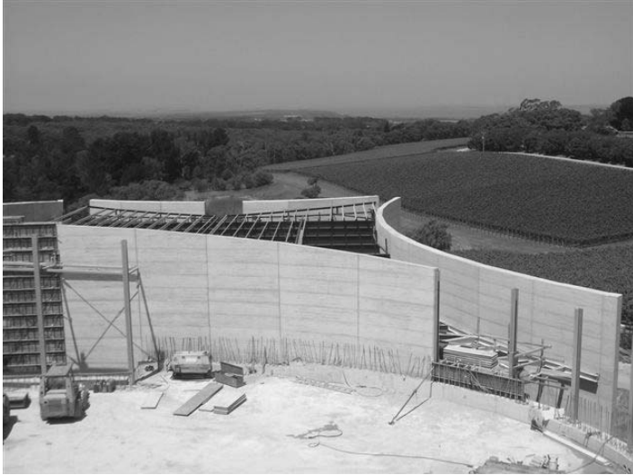
A1.2 Port Phillip Estate under construction.
