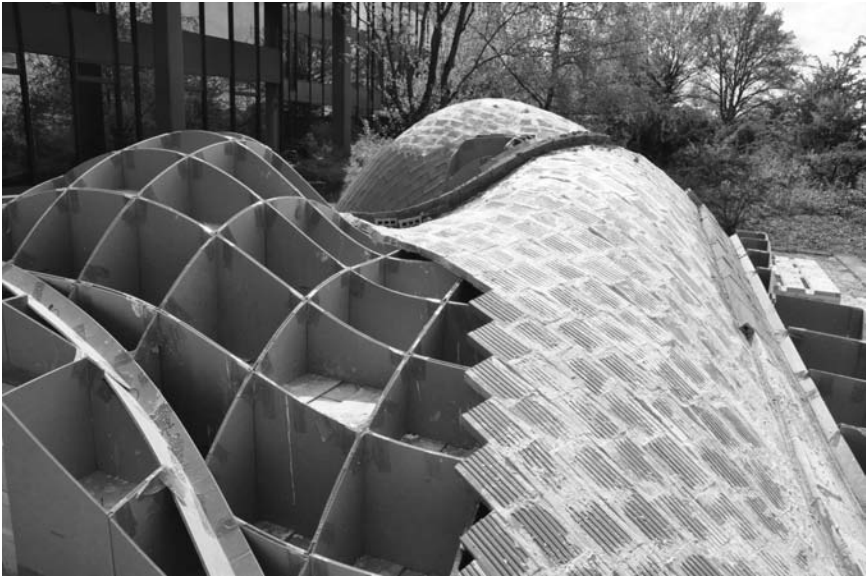
17.16 Continuous expandable cardboard guidework system during construction (photo: Lara Davis).
