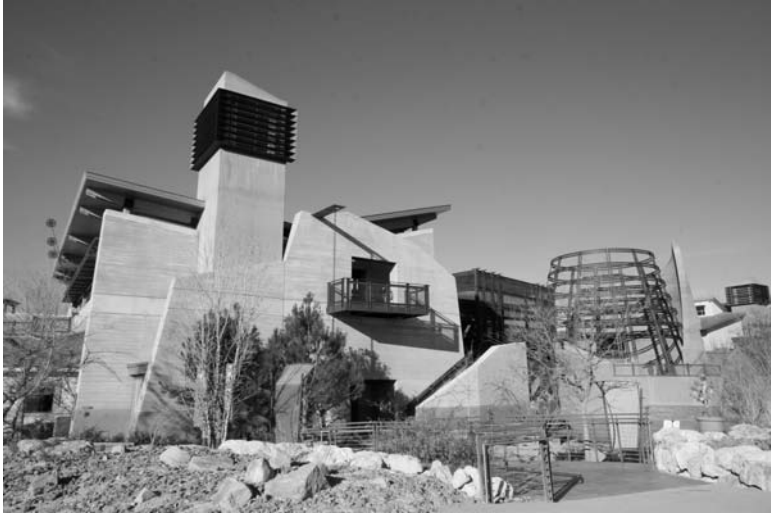
14.1 Rammed earth with modern aesthetic, Las Vegas, NV.
