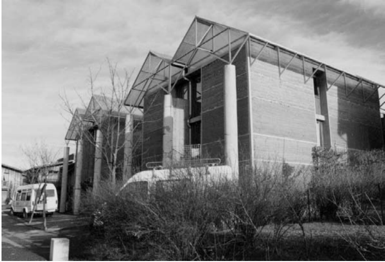
23.17 Stabilised compressed earth block apartment block at Domaine de la Terre, l'Isle d'Abeau (© Teresa Kelm, 2011).
