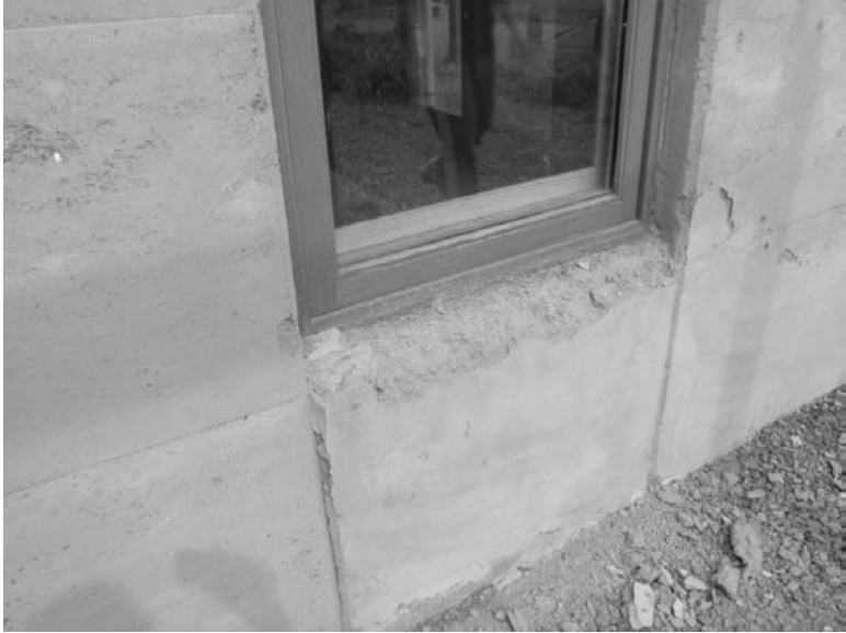
A1.4 Unstabilised earth walls, Omeo, Victoria.
