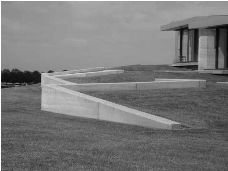
22.17 Landscape SRE walls used to structure a lawn area. Flinders, Victoria.
