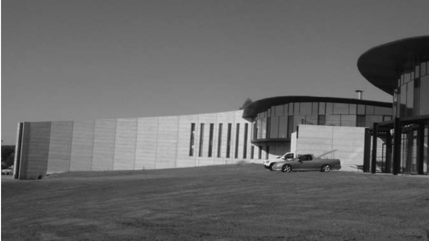
1.3 Port Phillip Estate, Red Hill, Australia. Facet SRE panels to 12.6 m height (© Earth Structures Pty Ltd, 2011).
