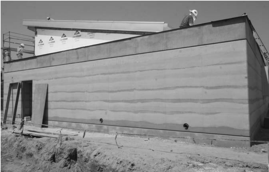
14.8 Rammed earth wall with color changes.
