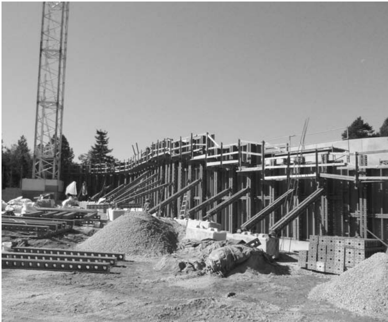
21.16 Concrete formwork used for curving rammed earth walls.
