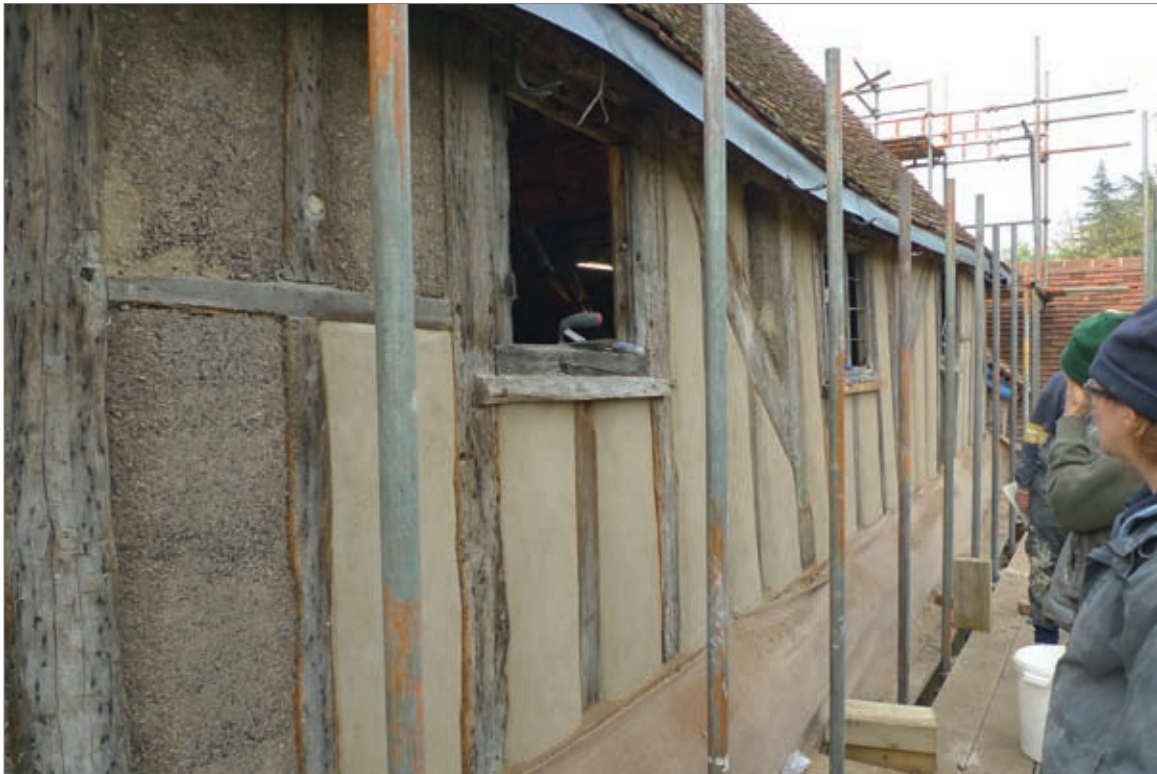
When the surface has dried sufficiently, finishes can be applied.
