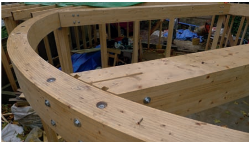
Glulam provides a more sustainable alternative to massive hardwood beams or steel joists.
