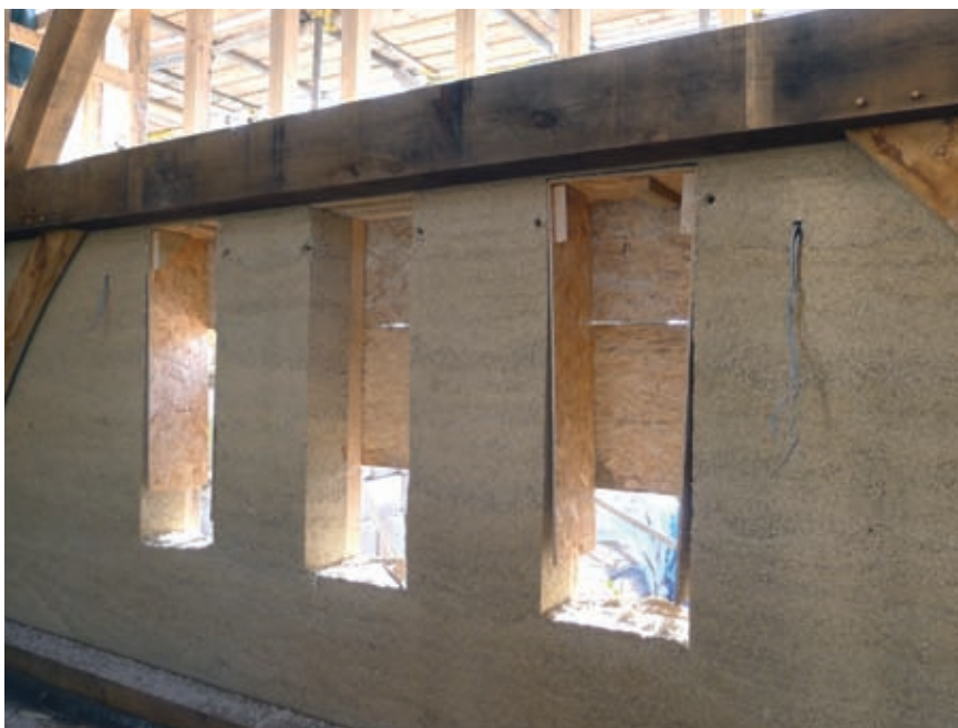
Window openings with shuttering partially removed.
