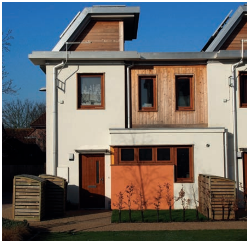
A variety of breathable finishes can be used on hempcrete buildings, such as the mixture of timber cladding and lime-based render at the Tomorrow's Garden City development in Letchworth.
