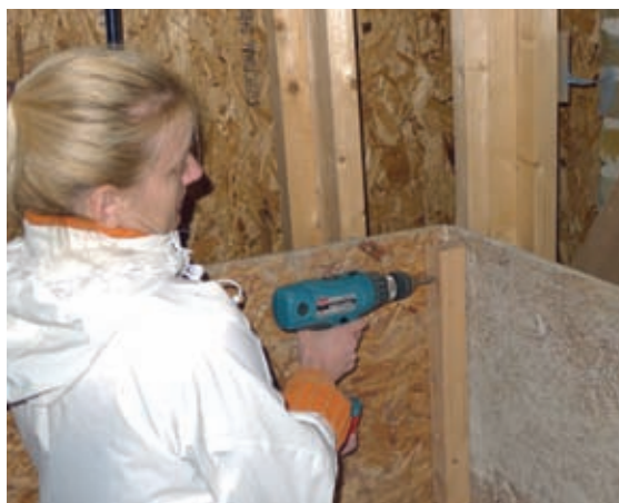
Fixing shuttering for an internal corner.
