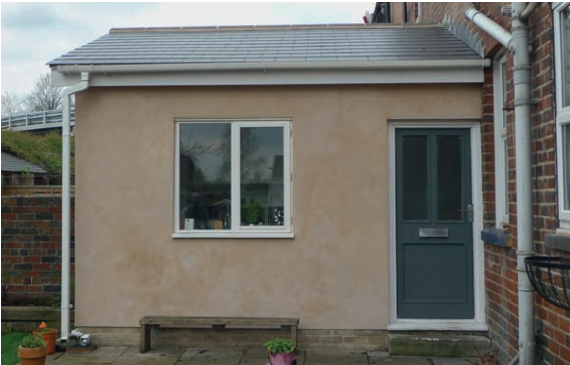
This hempcrete extension was built on a raft foundation (see step-by-step photos on page 150).
