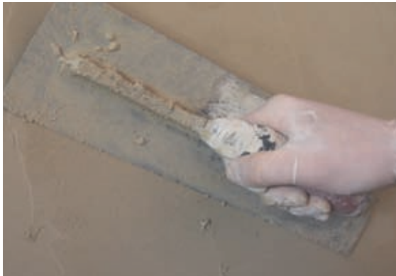
Gradually angle the trowel towards the wall to apply all of the plaster.
