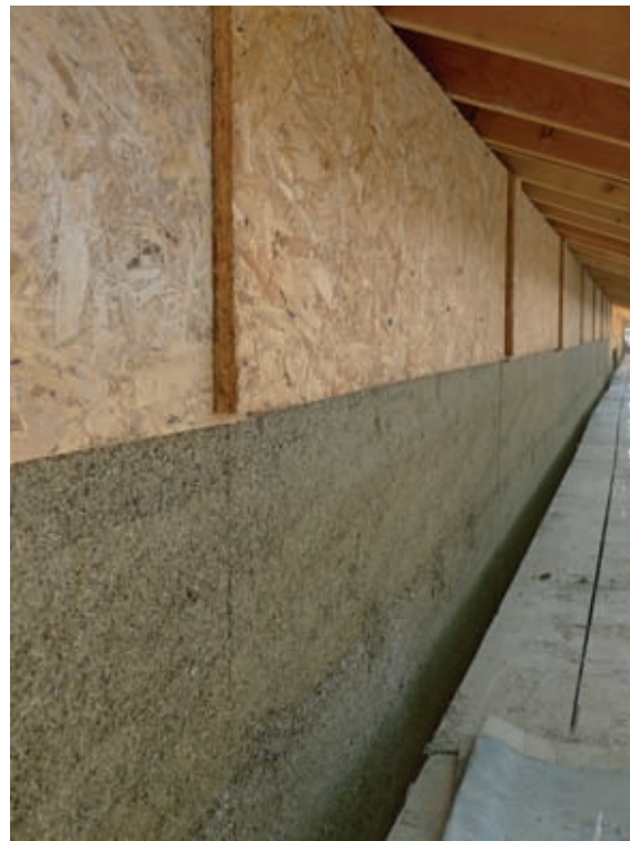
Shuttering partially removed from a hempcrete wall.
