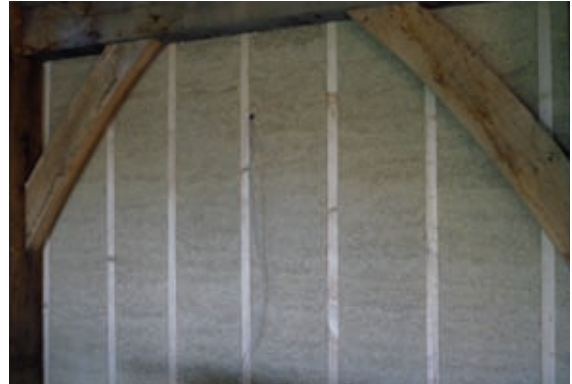
Exposed frame on the internal face of the wall.
