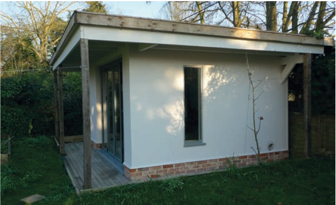
Accuracy at the framing stage makes applying render and plaster finishes easier, and allows the formation of very straight walls, as demonstrated in the clean lines of this garden office building.
