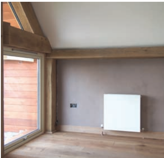
Lime plaster in a new-build hempcrete house.
