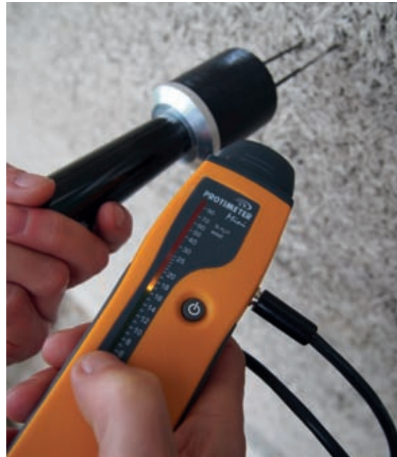
100mm probes allow testing at depth within the wall.
