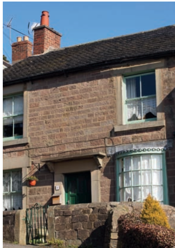
Vernacular buildings, such as this Derbyshire miner's cottage built about 1840, can provide lessons in how to site and orientate a new building, and how to make the best use of local materials.
