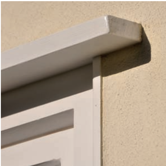
Oak drip details on a hempcrete house, above the window and at the sill.
