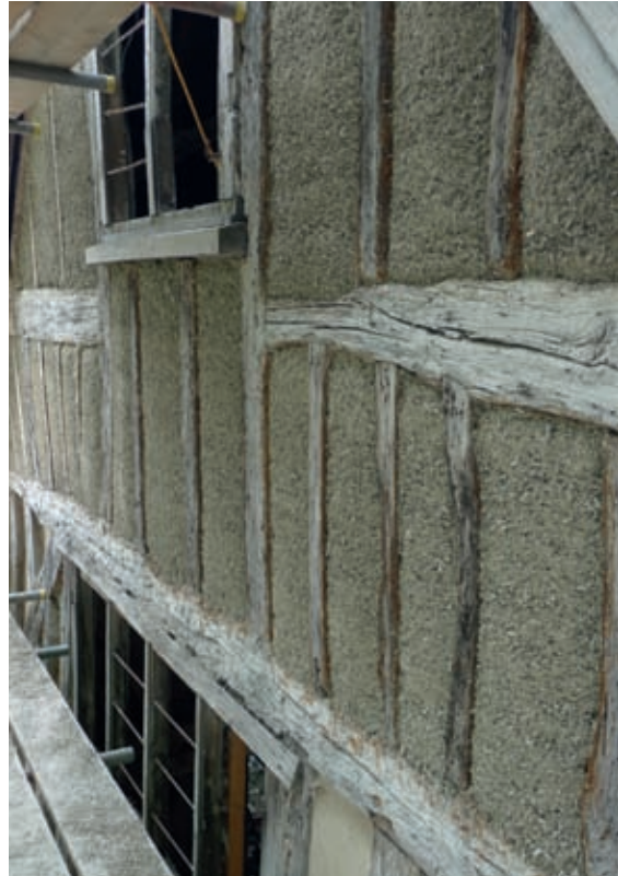
The same wall with hempcrete cast and shaped.
