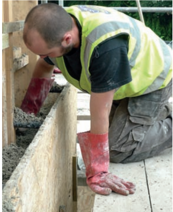
The loose hempcrete is spread around evenly, and patted down.
