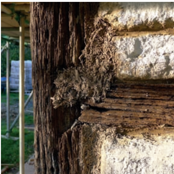
Hempcrete can be used to fill small spaces and voids in old buildings, like a natural building equivalent of expanding foam.
