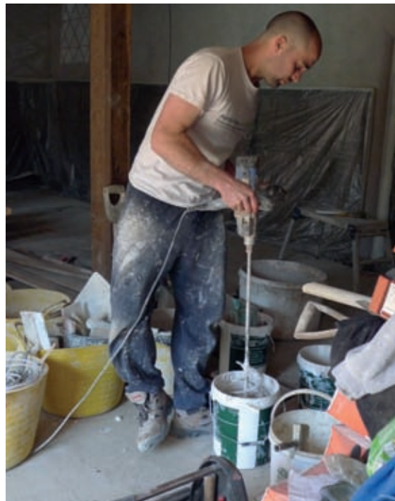
‘Knocking up’ a pre-mixed lime putty plaster to a workable consistency before use.
