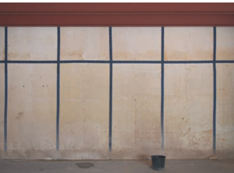
Magnesium silicate permanent shuttering, from inside the building.
