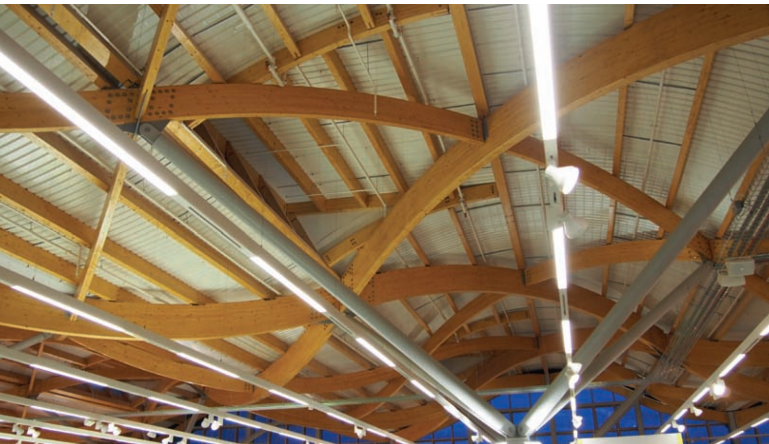
Glulam roof structure in a large hempcrete building.
