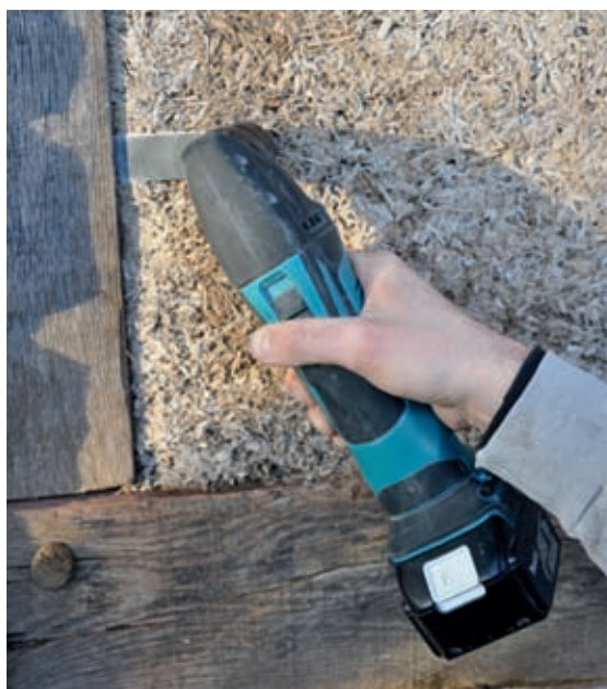
A multi-tool is useful for carving and shaping hempcrete.
