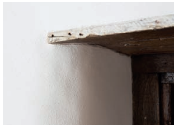
Curved corners and window reveals eliminate the need for corner beads in the plaster.
