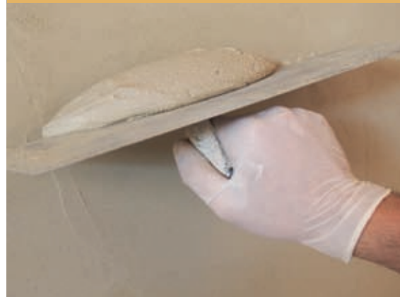
Using a laying-on trowel to apply the plaster.
