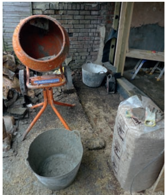
Mixing and placing hempcrete is a low-tech process.
