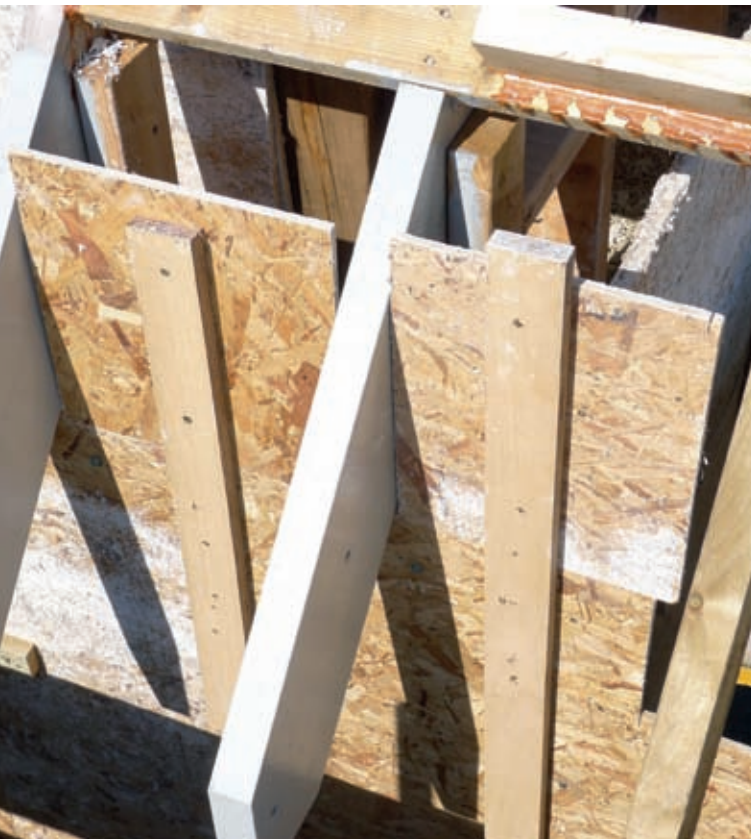
'Lollipops' extend the shuttering into the eaves.
