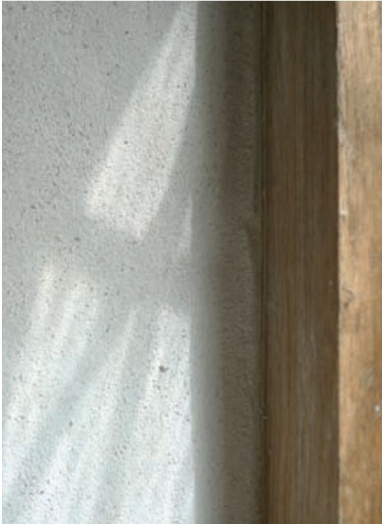
Traditional lime plasters, such as this lime putty plaster, form vapour-permeable finishes. The surface is rubbed back to 'open it up' and improve breathability (see page 240).
