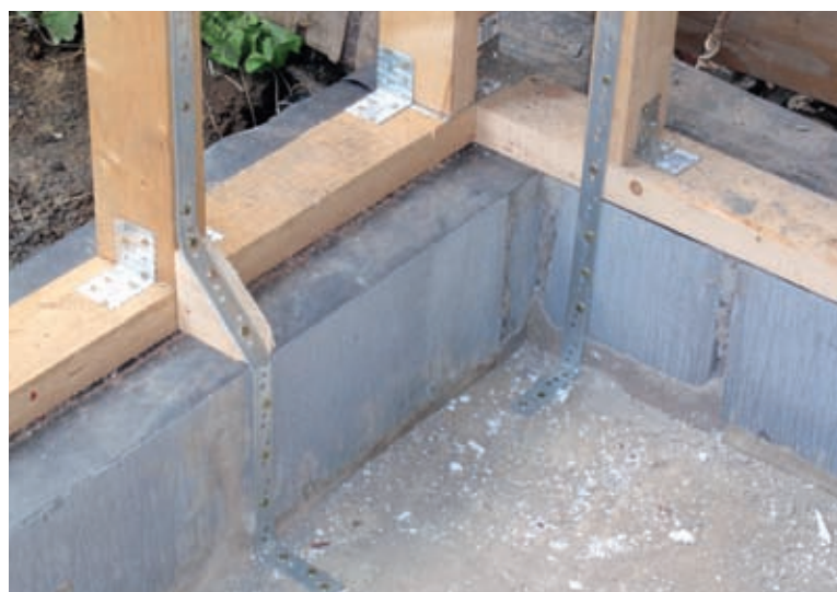
Metal straps are used to secure the sole plate.
