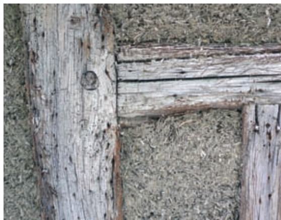
Hempcrete also fits against old timber frames much more snugly than board insulation does.
