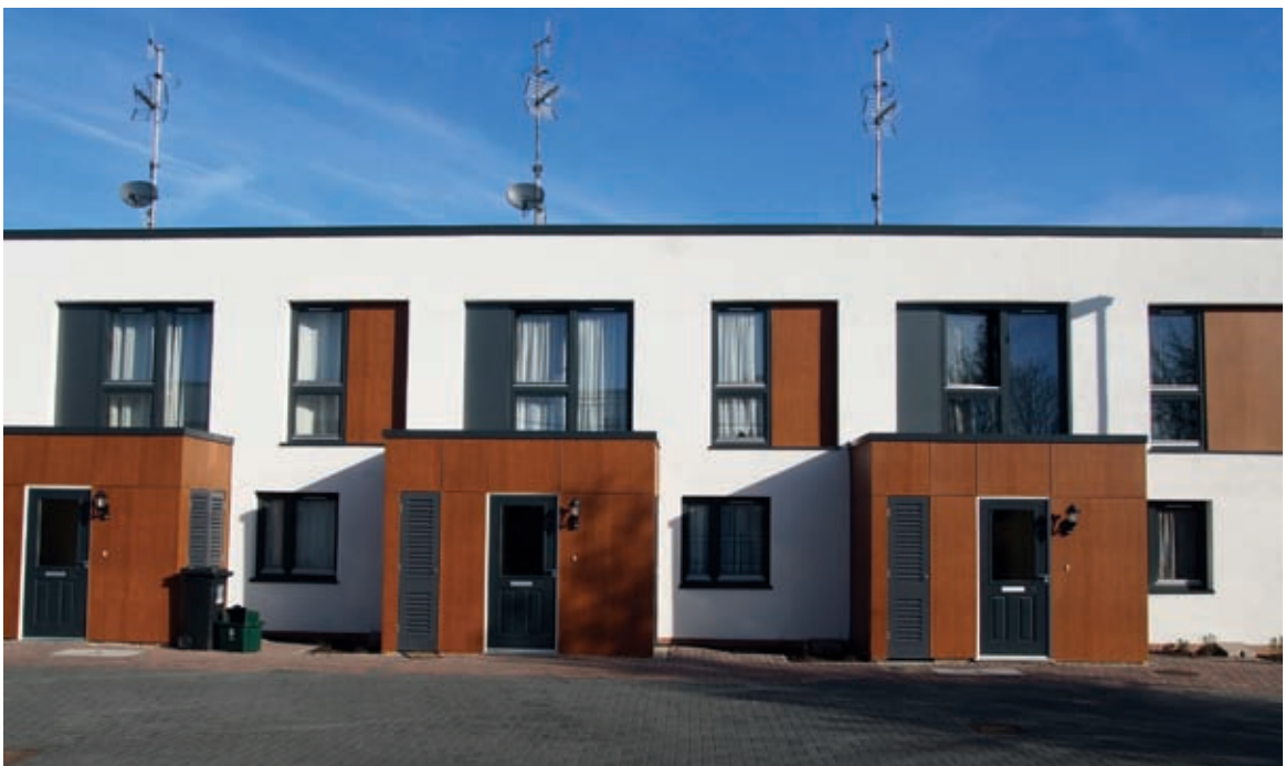
Social housing at Callowlands in Watford, built using a timber frame and cast-in-situ hempcrete.
