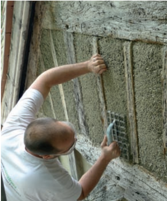
Hempcrete can be shaped with a nail or grid float after casting.
