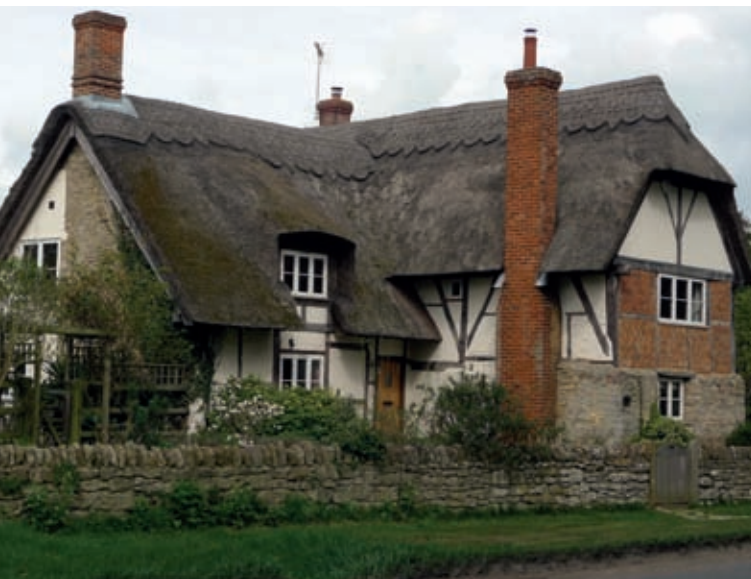
Traditional building materials allow moisture to pass through, keeping the structure in good 'health'.
