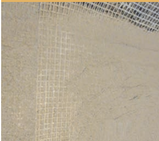
Mesh sunk into basecoat plaster.
