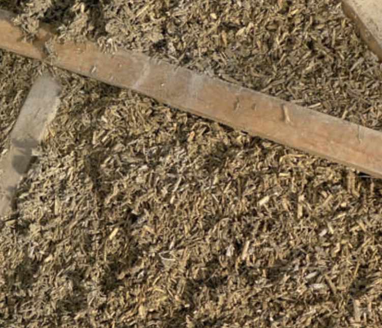
Low-density hempcrete used as roof insulation.
