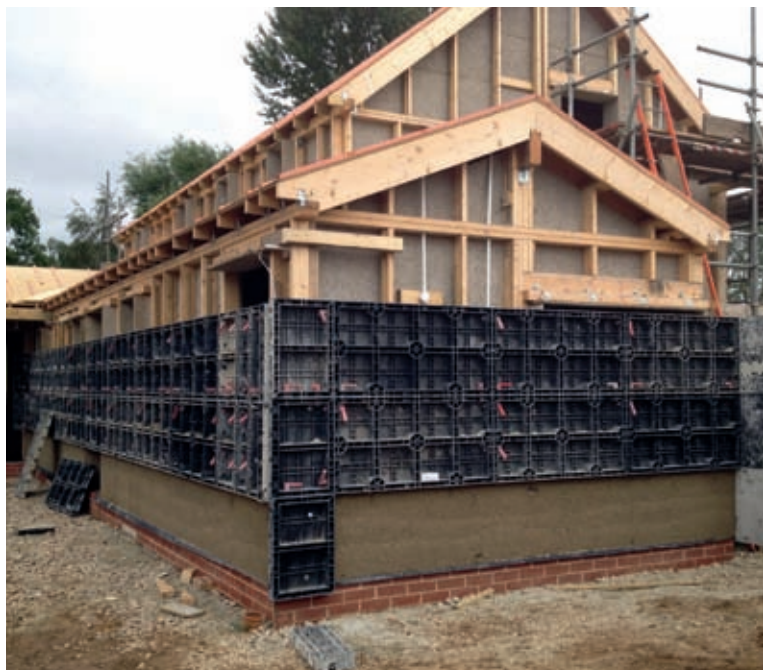
Plastic reusable shuttering. Image: The Limecrete Company
