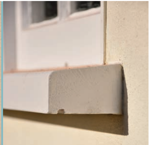
Oak drip details on a hempcrete house, above the window and at the sill.
