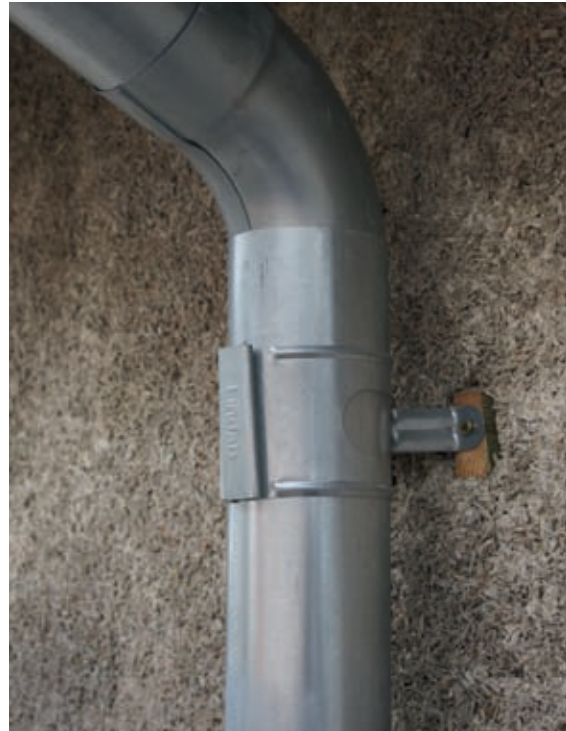
Downpipe fixed into hempcrete with wooden wedges.
