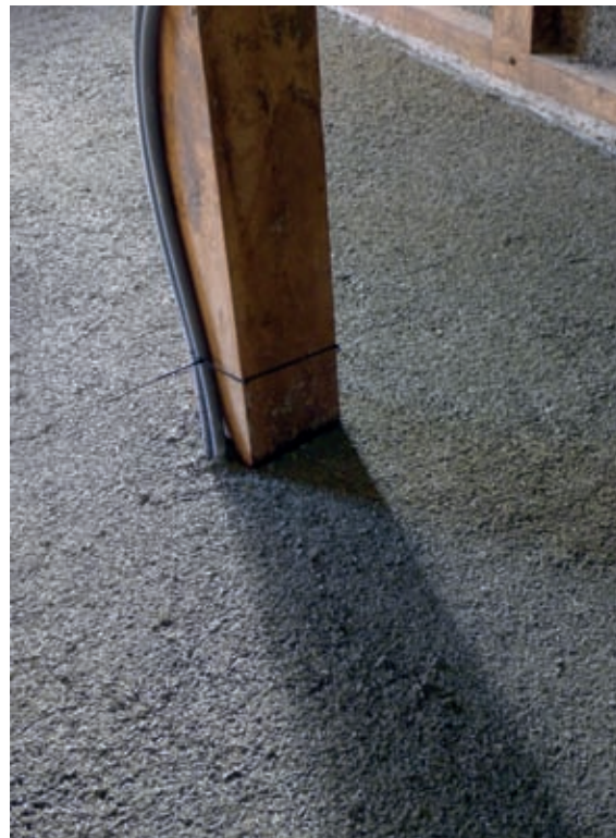
A freshly cast hempcrete floor.
