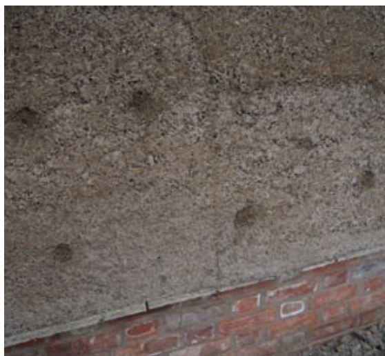
Spacer holes are filled in later with a little hempcrete mix.
