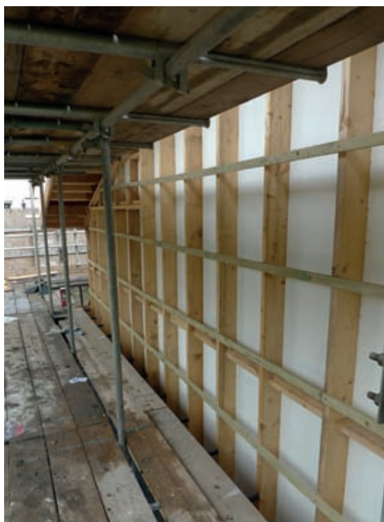
Permanent shuttering using magnesium silicate board, viewed from outside the building.
