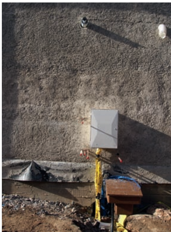
Services can easily be brought through a hempcrete wall.
