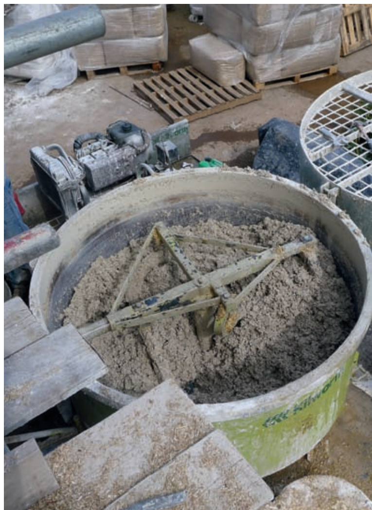
Pan mixer opened to show paddles and hempcrete mix. (Note: never use a pan mixer with the lid open!)
