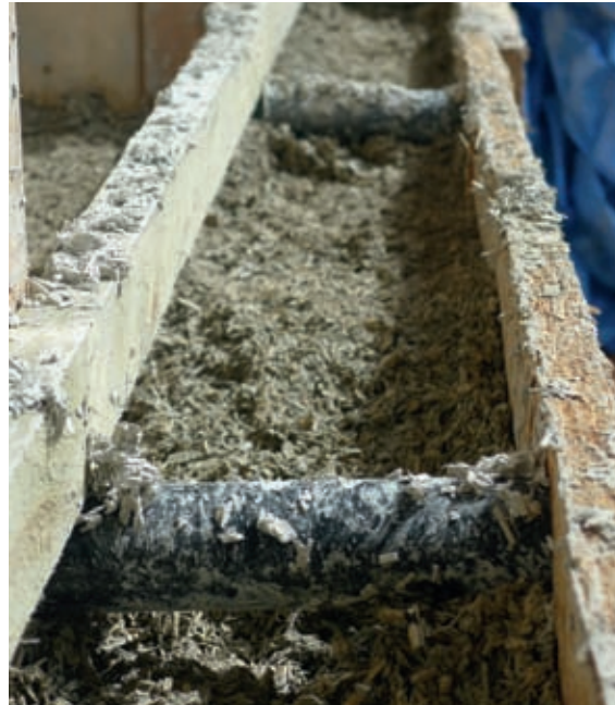
A section of shuttering filled with hempcrete.
