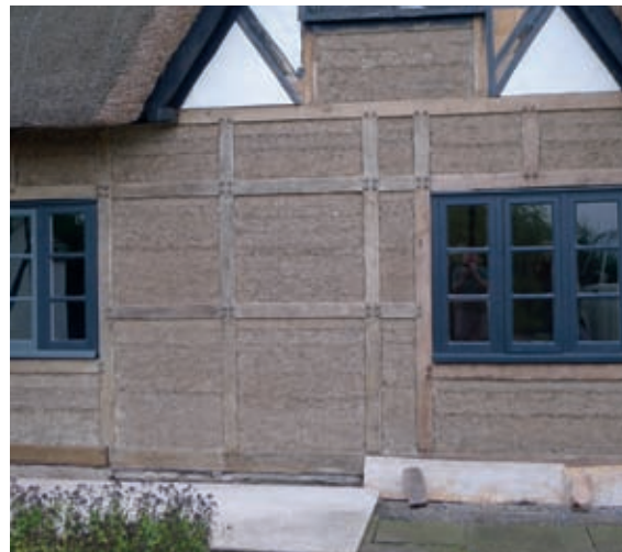
Completed hempcrete infill panels before plastering.
