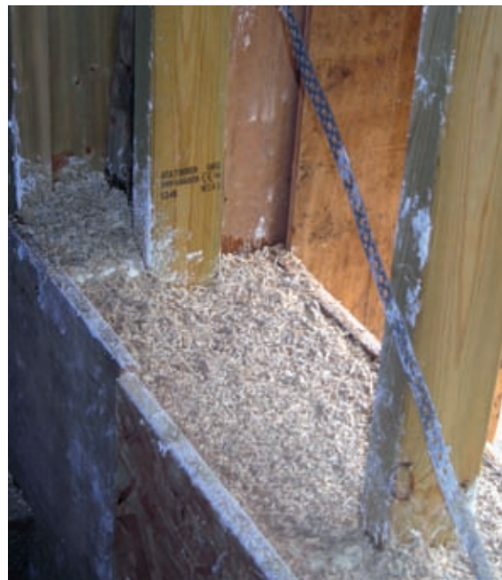
Diagonal stainless-steel strapping used as a brace. Image: Peter King
