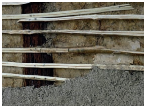
Daubed hempcrete over a wattle-and-daub panel, using split hazel poles to provide a key.
