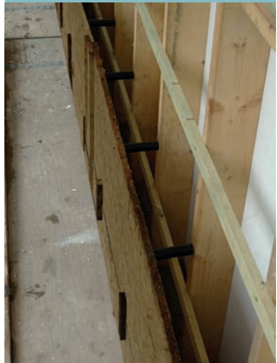
Exposed frame internally for permanent shuttering, showing horizontal rails.
