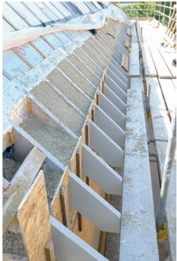
Hempcrete placed between rafters using 'lollipops'.
