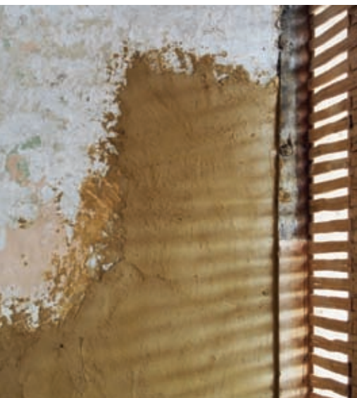
Clay plasters used in the repair of a historic timber-frame property.
