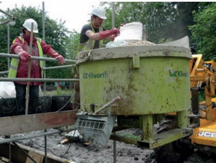
Mixing hempcrete for hand-placing.
