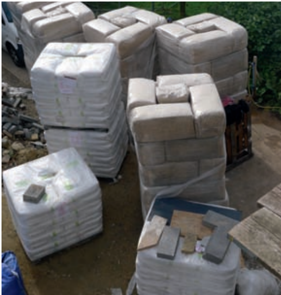
Hemp shiv and binder waiting to be mixed.
