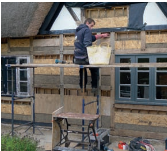
Casting hempcrete as timber-frame infill panels.
