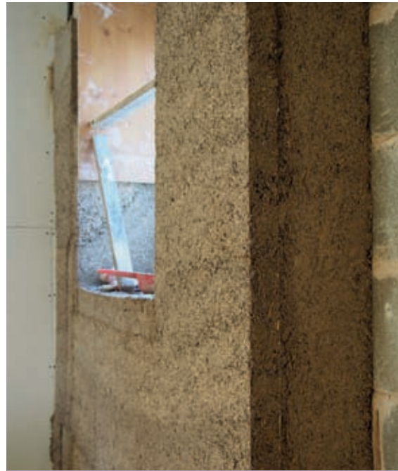
A completed wall of hempcrete solid-wall internal insulation.
