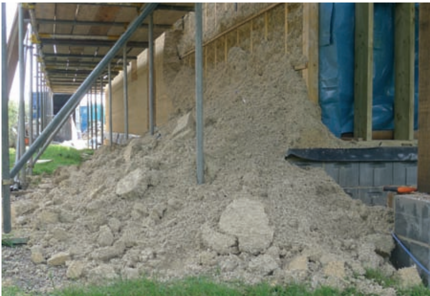
The catastrophic effects of excessive dust in hemp shiv.
