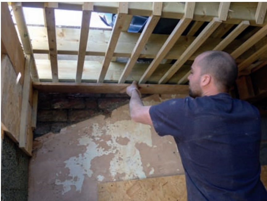
Erecting shuttering for a hempcrete ceiling.
