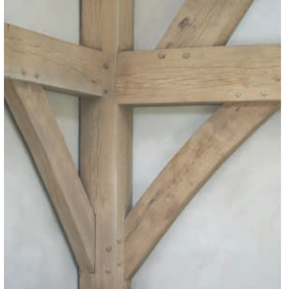
Lime plaster and an oak frame in a new-build hempcrete house.
