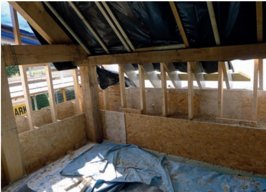
Hempcrete is always cast around a structural frame.
