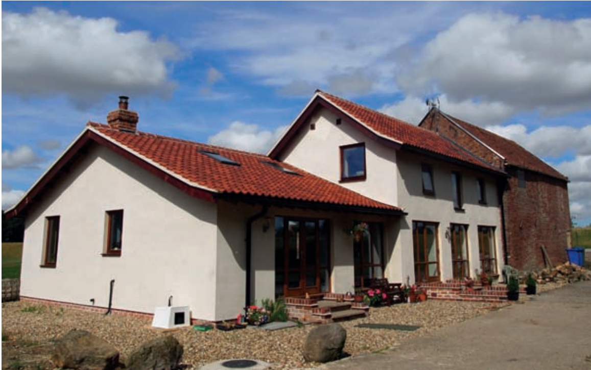
A self-build barn conversion using hempcrete for external insulation and internal walls.
