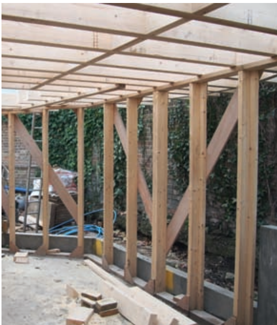
Timber frame with diagonal plywood braces and timber gussets.
