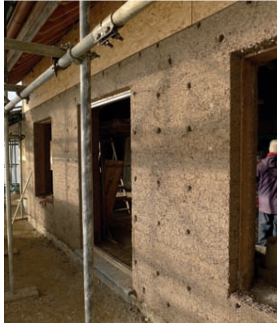
Hempcrete is used for walls . . .
