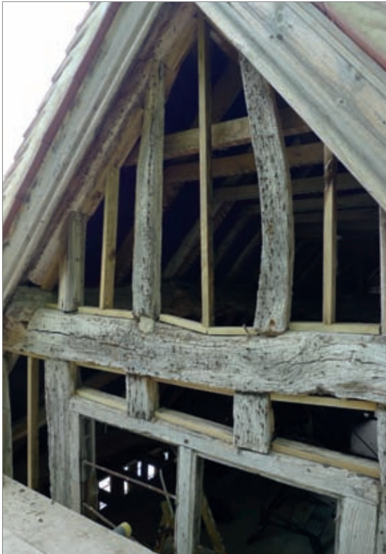
Reinforcing structure within a timber-frame panel.
