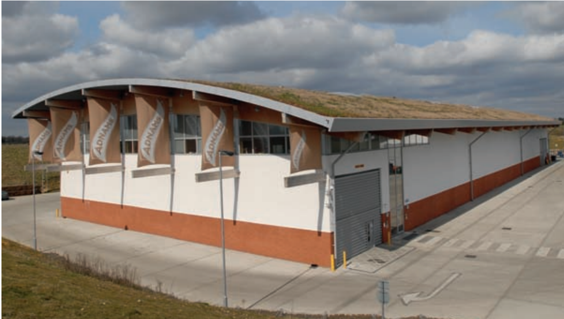
Adnams' distribution warehouse was constructed from a mixture of hempcrete blocks and cast-in-situ hempcrete. Image: Adnams
