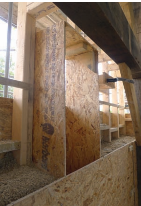
Shuttering for openings in the wall.
