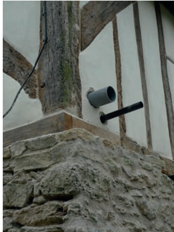
Waste pipes fitted by drilling through the hempcrete.
