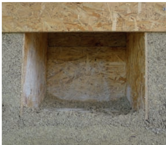
Hempcrete freshly cast around a window opening.
