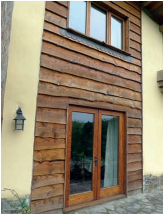
Timber cladding over a hempcrete section in a cob wall.
