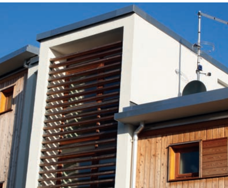
Timber cladding and render are the two most frequently used finishes for hempcrete.
