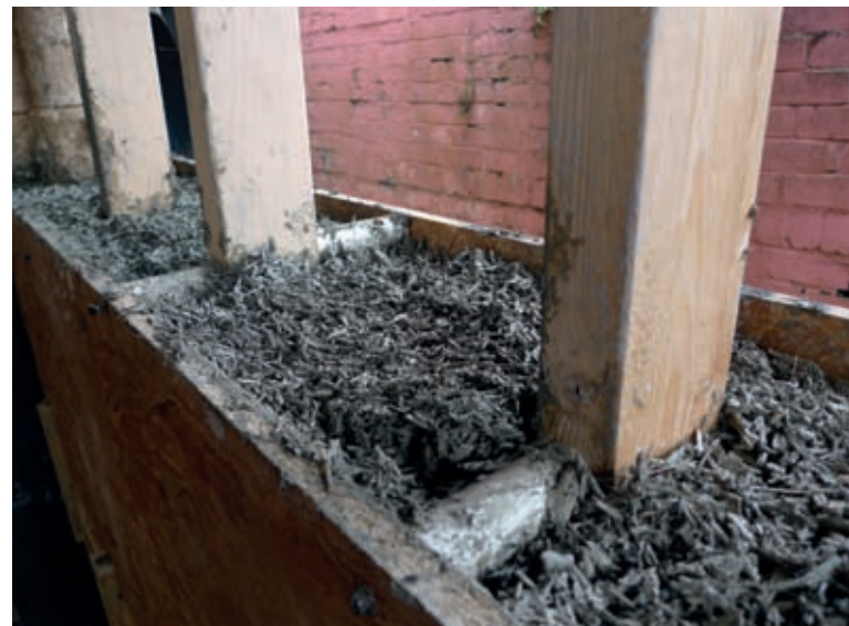
Cast-in-situ hand-placed hempcrete around a softwood timber structural frame.
