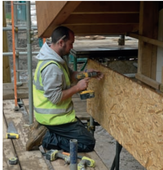
Waterproofs or knee pads help to minimize lime burns in wet weather.
