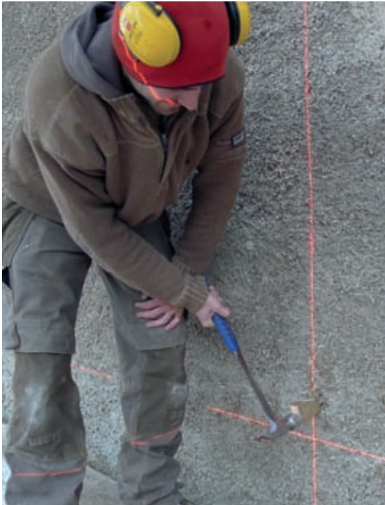
Hammering a wooden wedge into a hempcrete wall.
