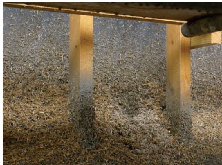
Sprayed hemp is projected against a permanent shuttering board.
