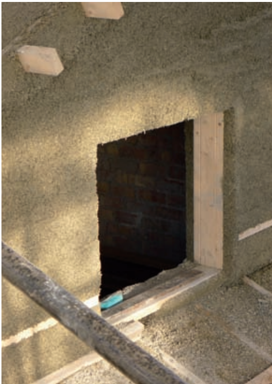
Hempcrete can be used for floor, wall and roof insulation and provides excellent acoustic, as well as thermal, performance.
