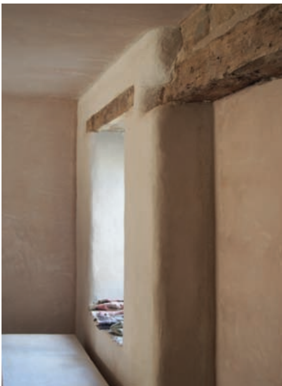
Lime and gypsum plasters side by side. The finish of the cream-coloured lime plaster around the window appears more textured and warm than the smooth gypsum on the surrounding walls and ceiling.
