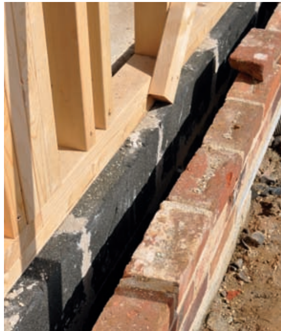
Load-bearing glass foam blocks used in a plinth.
