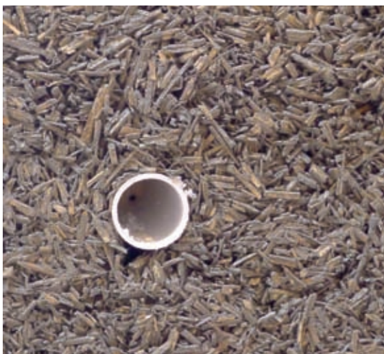
Remove spacers gently before the wall hardens.
