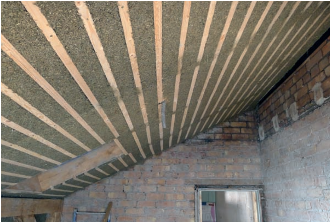
A freshly cast hempcrete ceiling with exposed battens.
