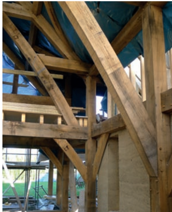
An oak frame, with hempcrete walls under construction.
