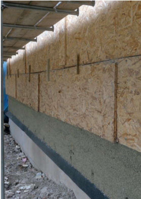
Shuttering made from OSB (oriented strand board).
