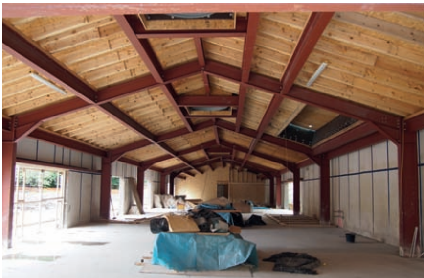
A steel supporting frame in a hempcrete community centre.
