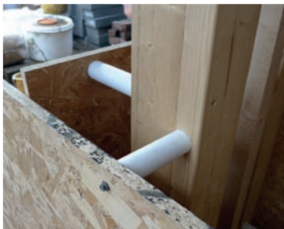
Shuttering for an external corner.
