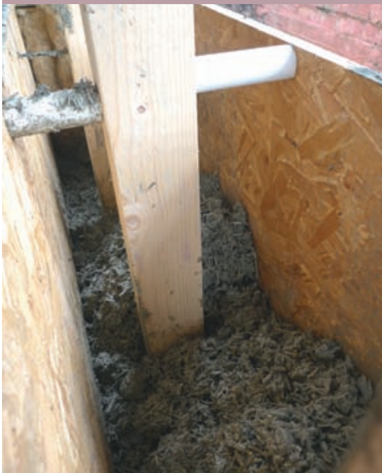
Hempcrete when first tipped into the void.
