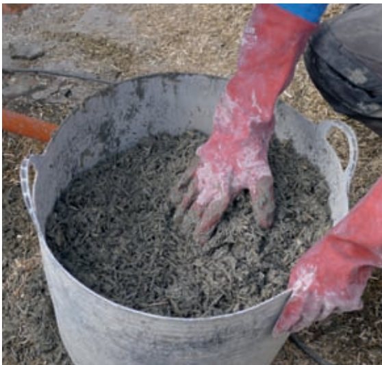
The right consistency is not too wet and not too dry.
