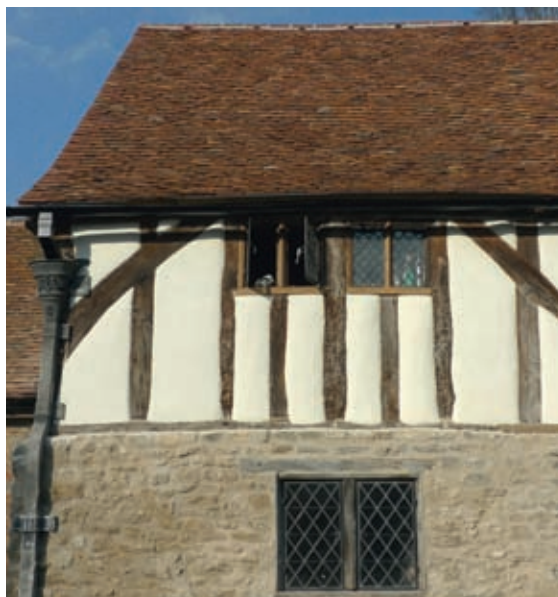
Hempcrete, lime render and limewash complement the original materials and aesthetic of this building.
