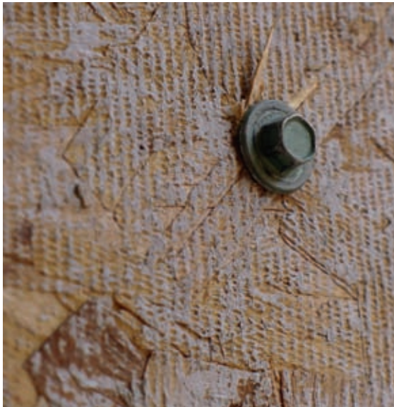
Long heavy-duty screws are ideal for fixing temporary shuttering.
