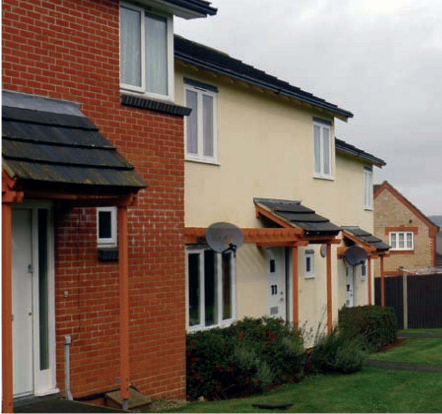
Hempcrete and neighbouring brick houses at Haverhill in Suffolk, which were monitored as part of a BRE study into the viability of hempcrete as a building material.
