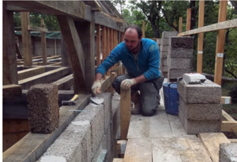
Hempcrete blocks are laid on a thin bed of lime mortar.
