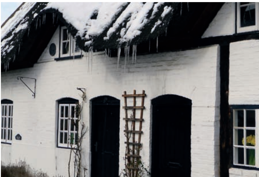
The orientation and shape of vernacular buildings can be a good source of inspiration for building design.
