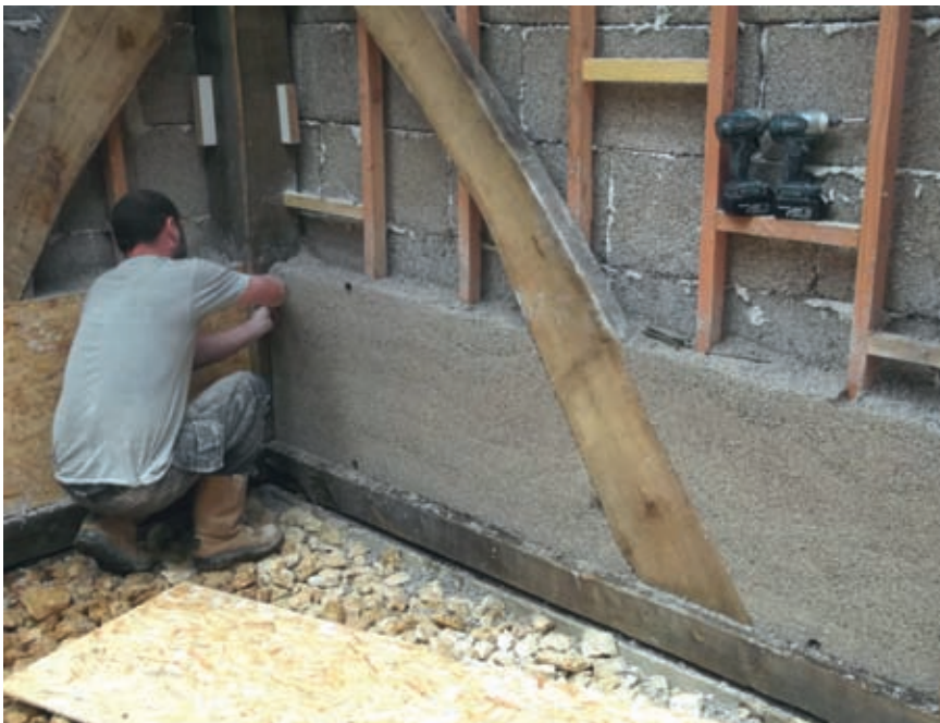
Hempcrete cast up against an outer skin of hempcrete blocks – combining some of the benefits of the pre-cast and cast-in-situ methods.
