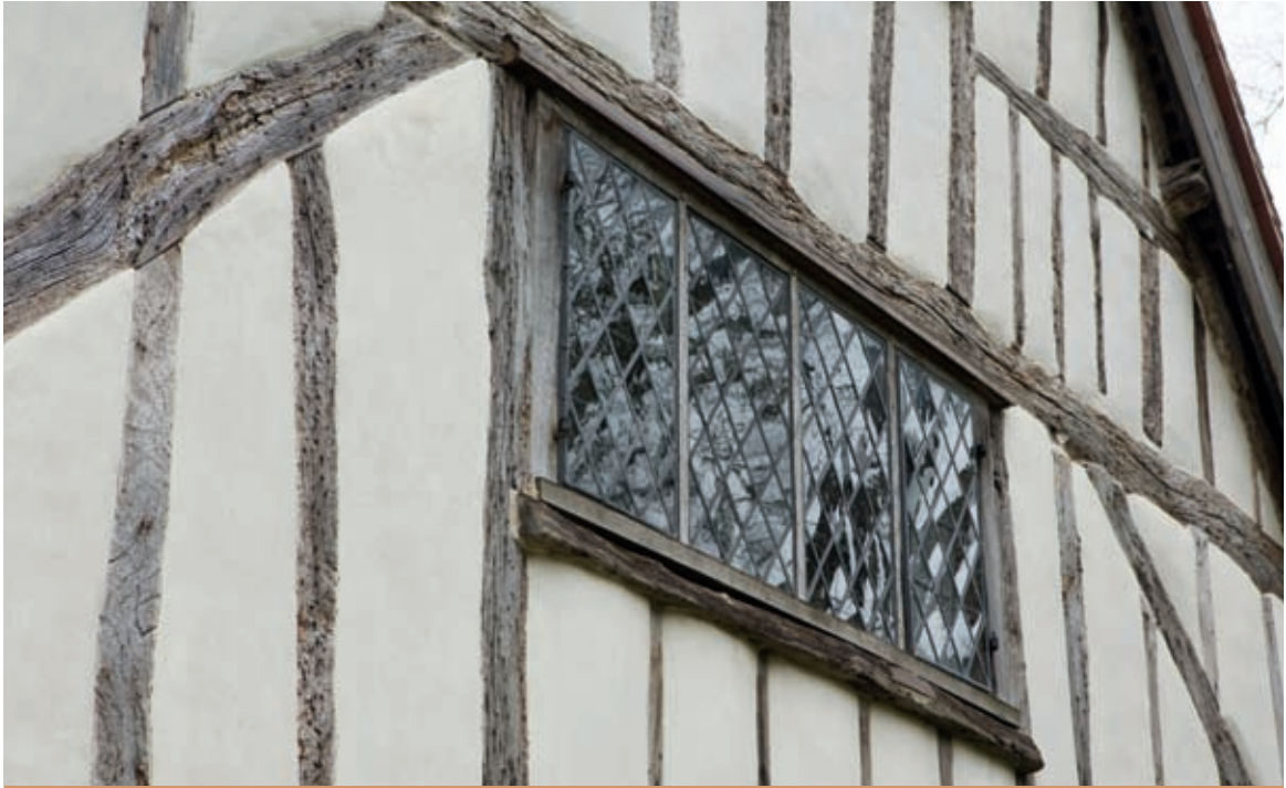
Hempcrete used as a replacement for wattle and daub.
