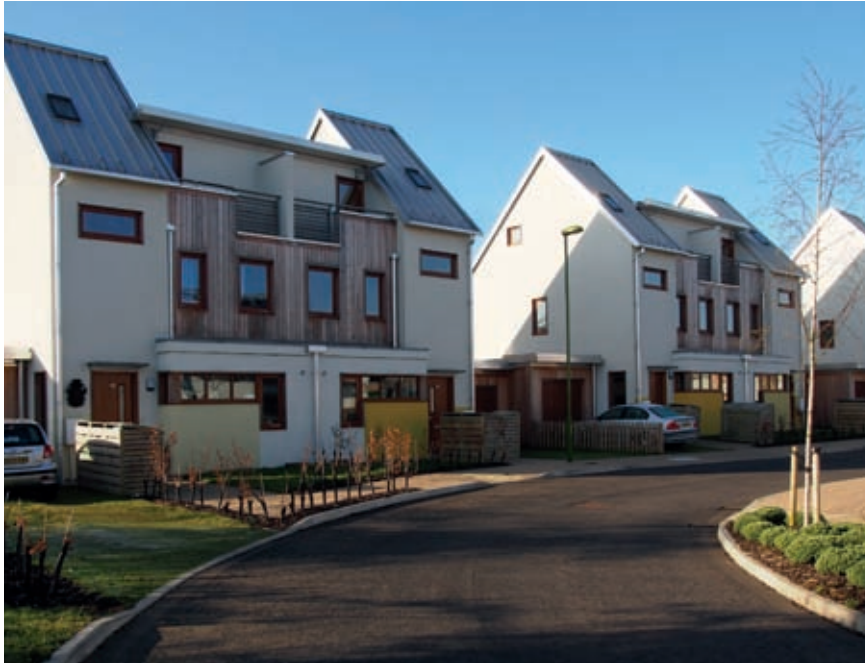
A new-build housing estate constructed with structural timber frames and hempcrete or wood-fibre insulation.
