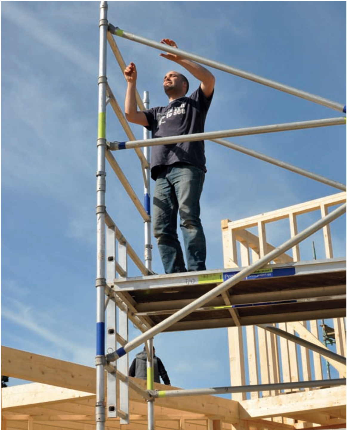
As on any building site, the usual safe working practices must be observed, such as using the correct access equipment when working at height.
