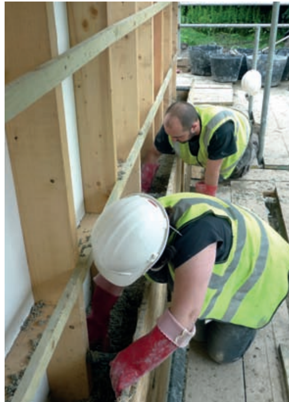
The tamping team at work.
