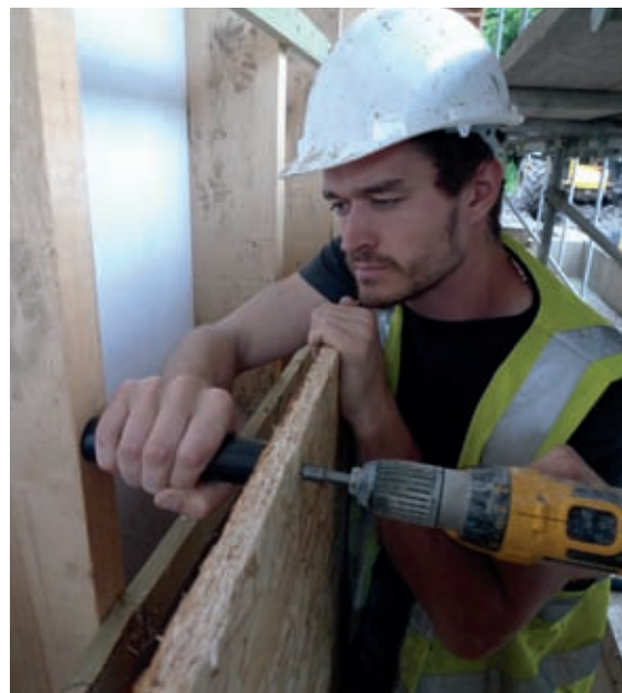
Fixing shuttering with screws and spacers.
