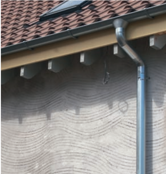
Basecoat render scratched up ready for the topcoat to be applied.
