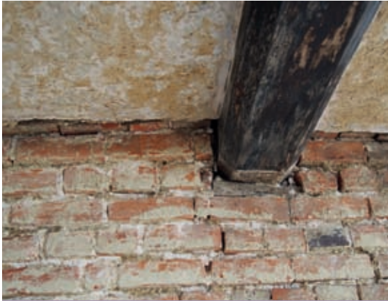
Traditional buildings were always built from natural, breathable materials, such as these clay bricks, oak beams and clay/lime plaster.
