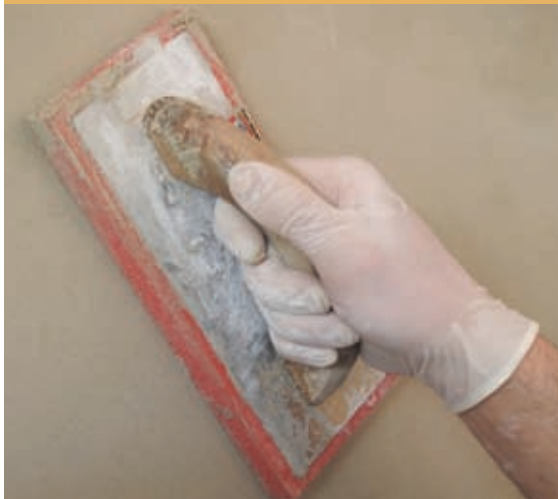
The right timing is crucial when rubbing back the plaster to achieve a finish.
