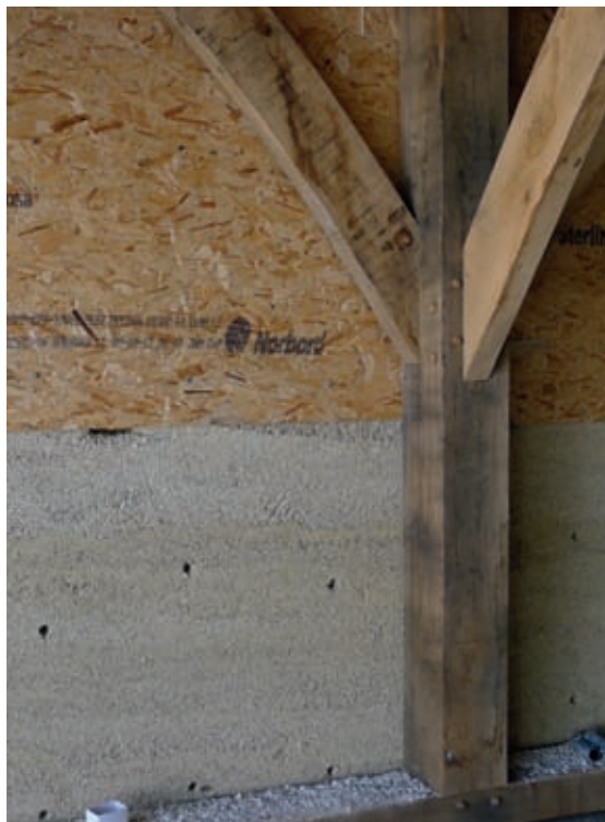
Shuttering partially removed from a wall with a central softwood frame.
