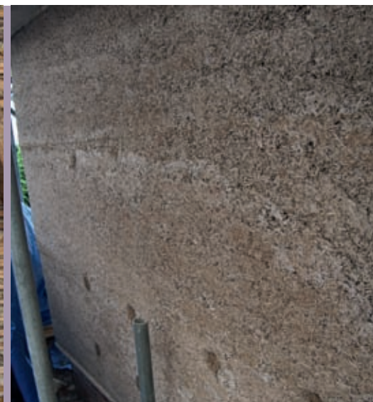
The same wall with hempcrete in place.
