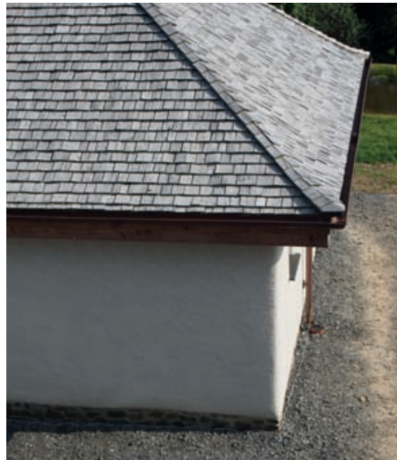
Sensible detailing on a hempcrete building in an exposed location: a moderate pitch of roof with a large overhang at the eaves. Oak shingles on the roof make an attractive counterpoint to the lime render.
