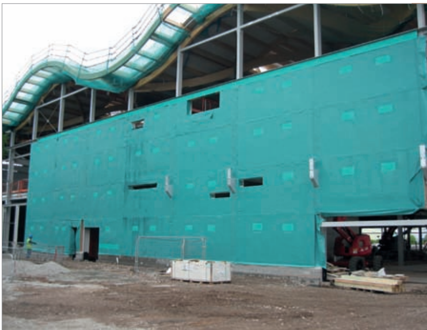
Panels being installed on-site. Image: Lime Technology Ltd
