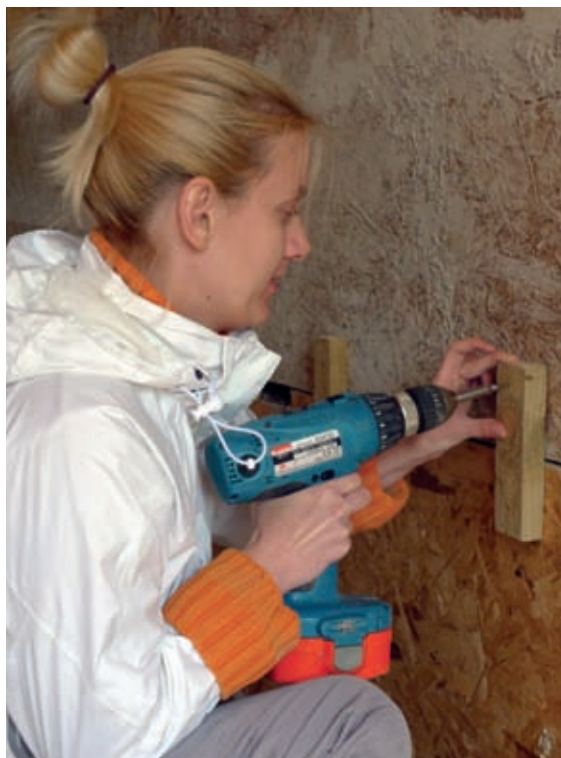
Fixing wooden straps in place to join two shuttering boards.
