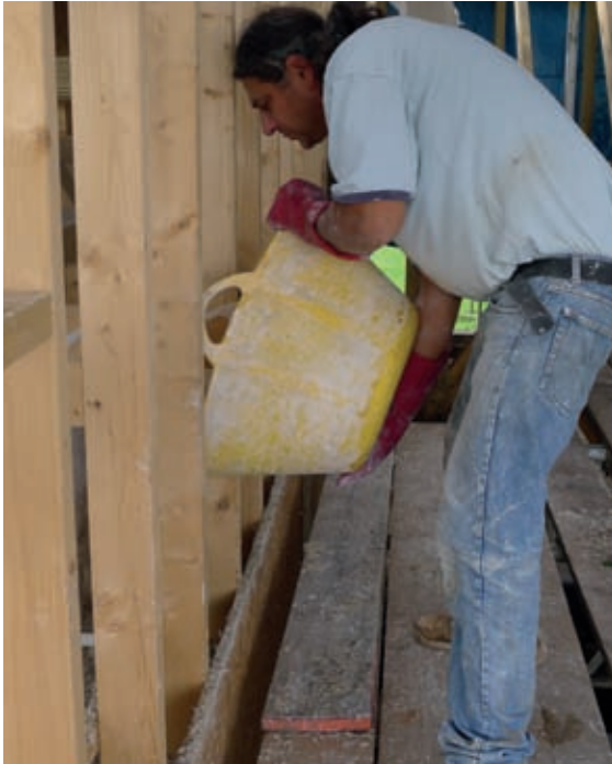
Hempcrete is tipped into the shuttering in layers of 100-150mm.
