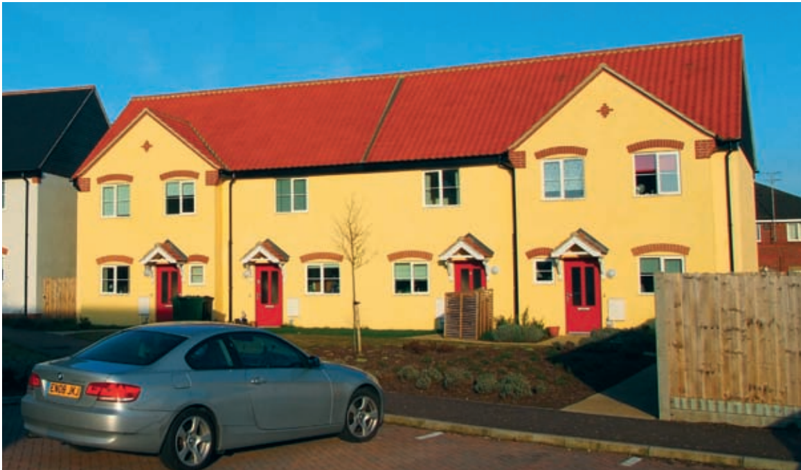
Hempcrete terrace at a housing association development in Diss, in Norfolk, constructed from cast-in-situ hempcrete around a timber frame.
