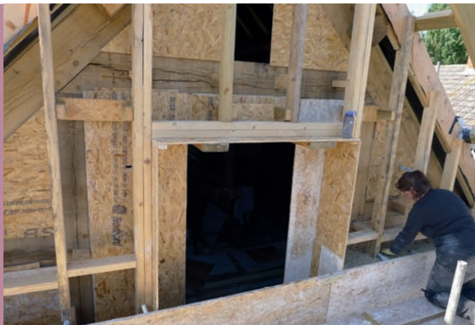
Shuttering for openings in the wall.
