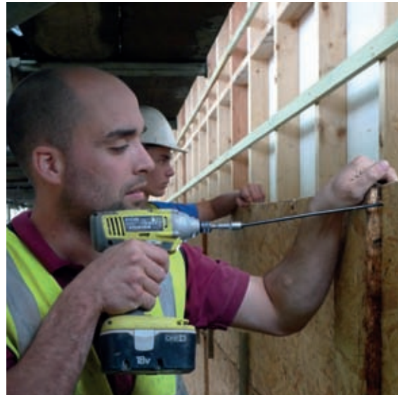
The shuttering team usually consists of two people.
