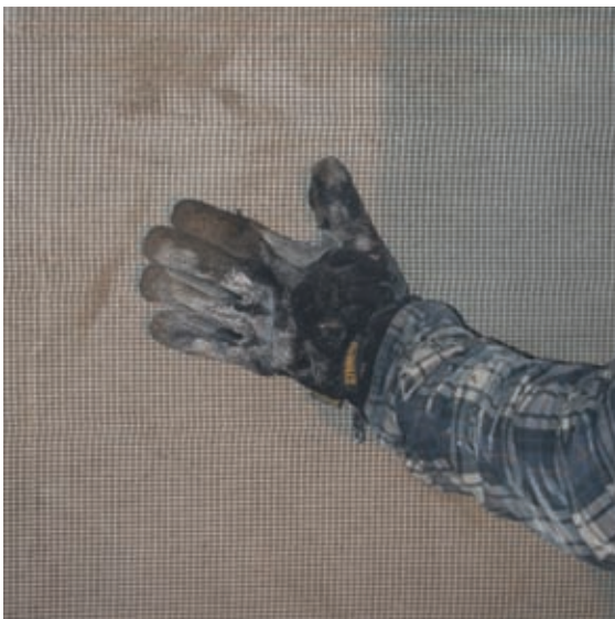
Rubbing glass-fibre mesh into the basecoat.
