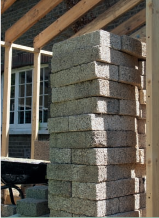
Owing to the unique mechanical properties of hempcrete, blocks still need to be cast around a structural frame.
