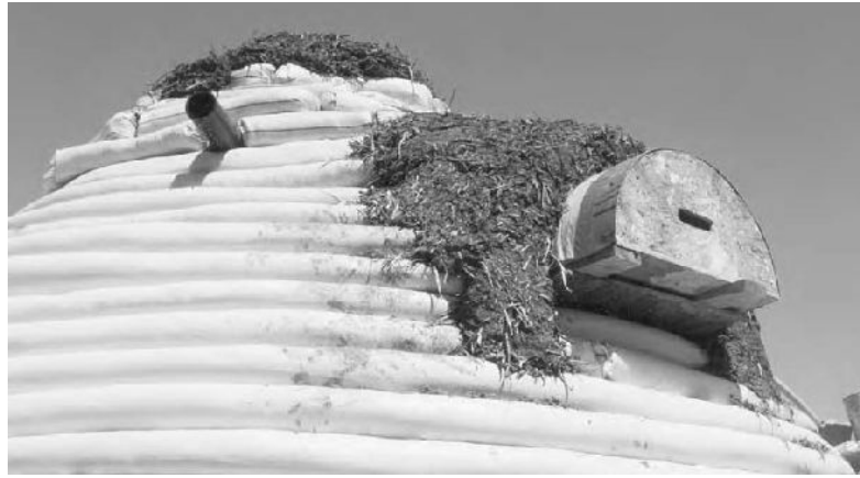
14.11: Sculpting the secondstory dormers around the arch forms of the Honey House.
