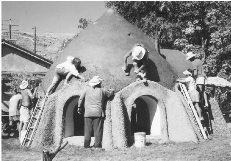
13.1: The Honey House receiving a natural-clay rich earthen roof plaster.
