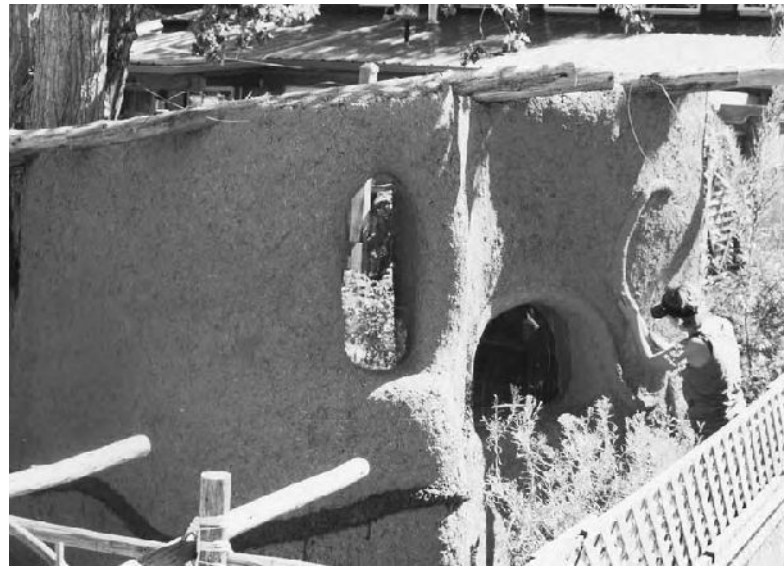
1.8: Michelle Wiley sculpting a cob shed in her backyard in Moab, Utah.
