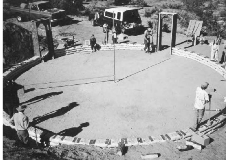
3.41: A 36-foot-diameter kiva-style earthbag home, going up in Wikieup, Arizona.
