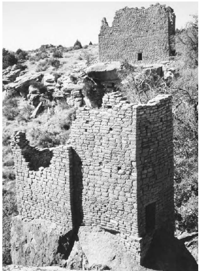
4.1: 1,000-year-old Anasazi dwelling on an exposed bedrock foundation in Hovenweep National Monument.
