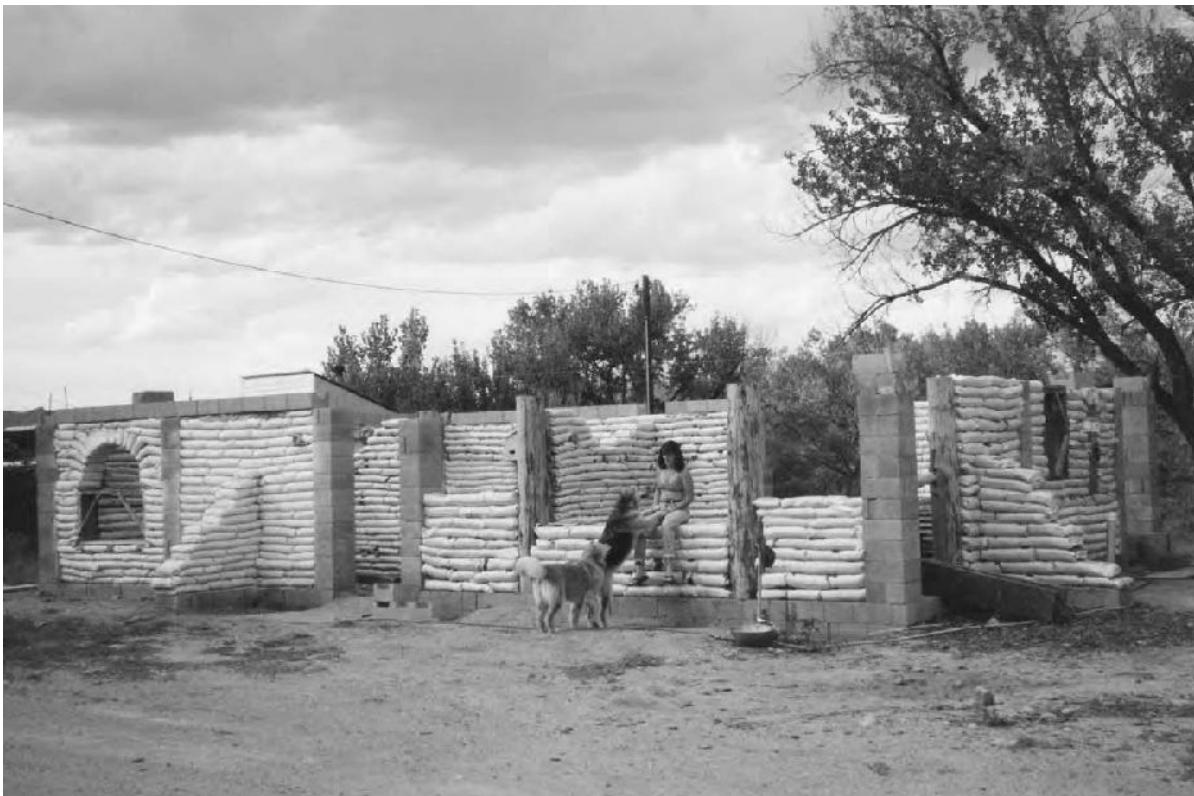
5.17: Alison Kennedy's code-approved earthbag home with concrete-block posts and beams.
