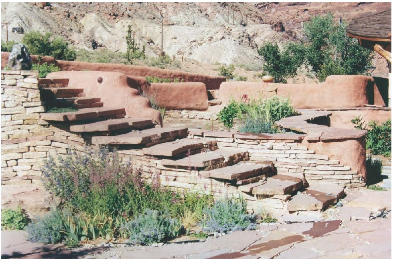
Susie Harrington and Kalen Jones staggered multiple tiers of earth-bag retaining walls to provide level gardening space with grace. Moab, Utah (Fig. 11, below right).
