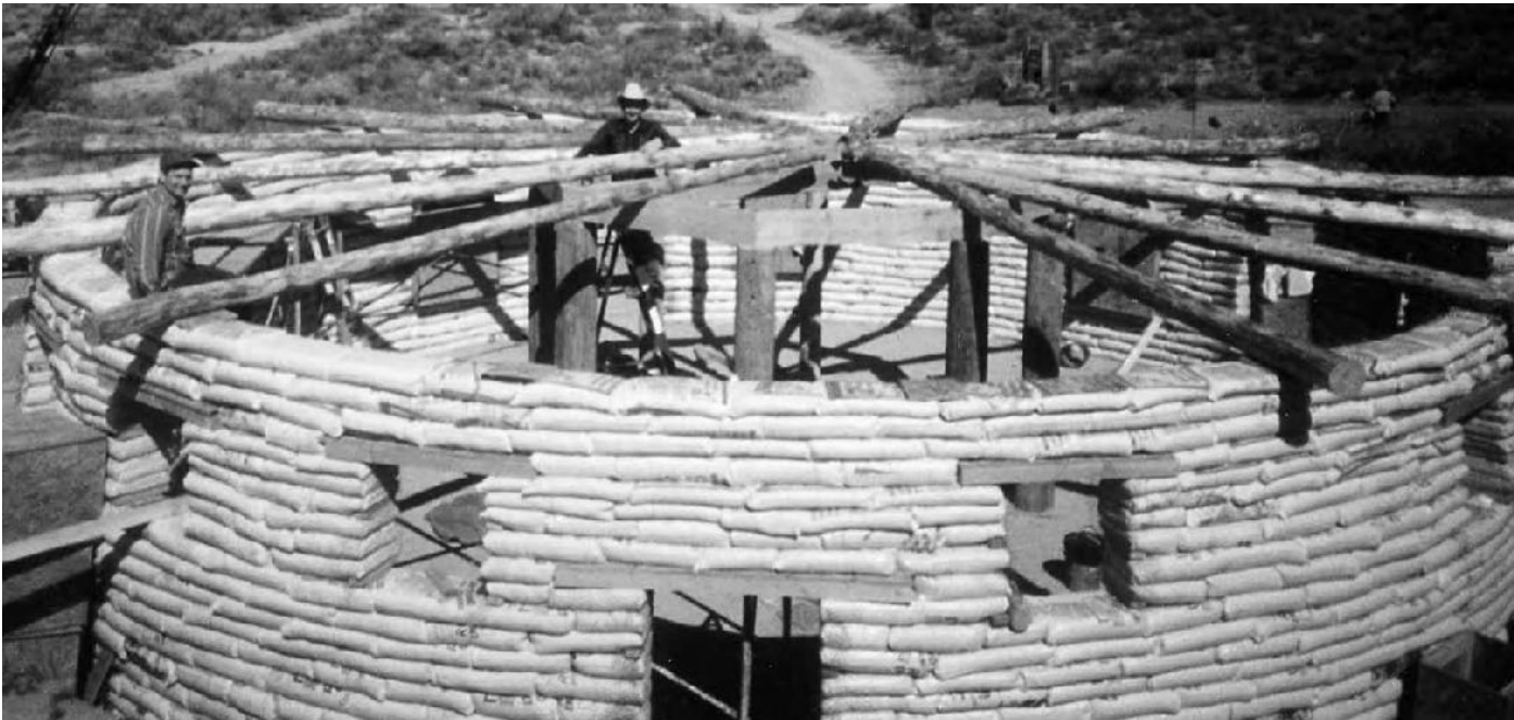
9.18 (below): A great example of the earthbag kiva is Penny Pennell's 36-foot (10.8 m) diameter home that uses a 6-sided post and beam interior support structure for the 20-foot (6 m) long vigas to rest on. (Credit: Penny Pennell)
