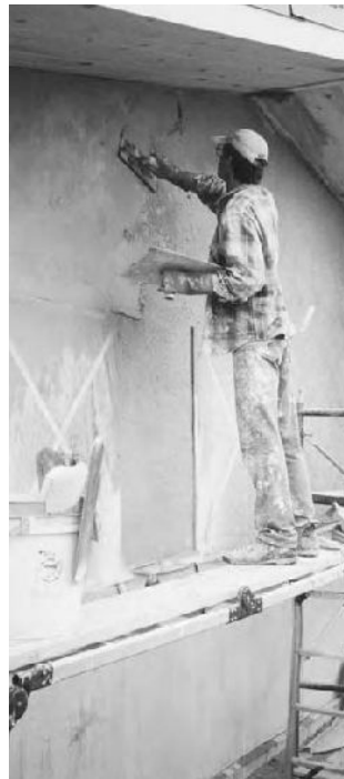
14.16b: Trowel application
