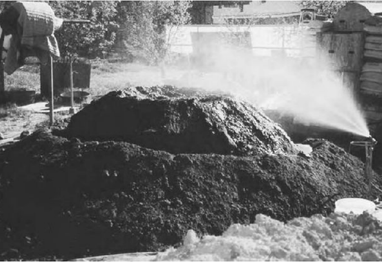
2.8: Using a sprinkler to pre-moisten a pile of dirt in preparation for wall building.
