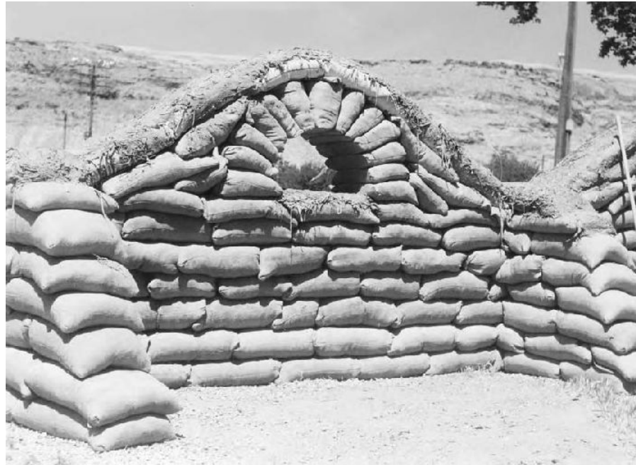
3.4: Our early bag work resembled stacks of feed sacks with their soft corners bulging out.
