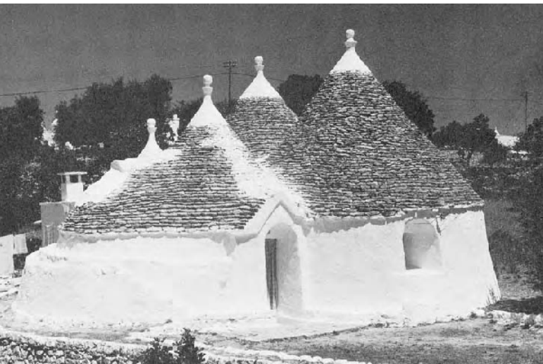
17.2: Lime whitewashed walls reflect the sun's intensity in sunny climates.
