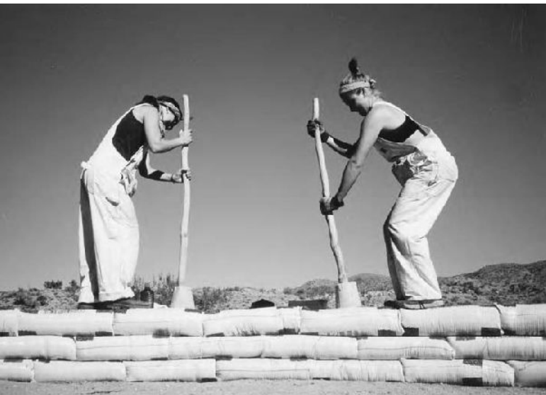
3.12: The row is tamped from above until the dirt goes from making a dull thud sound to a distinctive ringing sound.
