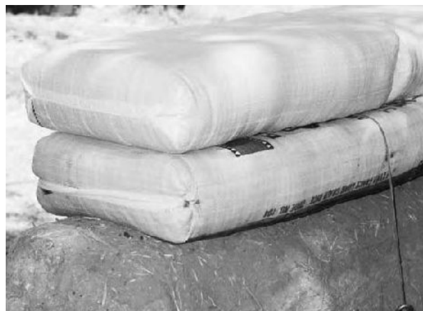
3.6: Inside-out gusseted bag on top of a diddled and locked bag. With the introduction of gusseted bags, diddling may become a lost art.
