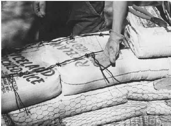
2.20: Tie wire looped around barbed wire.
