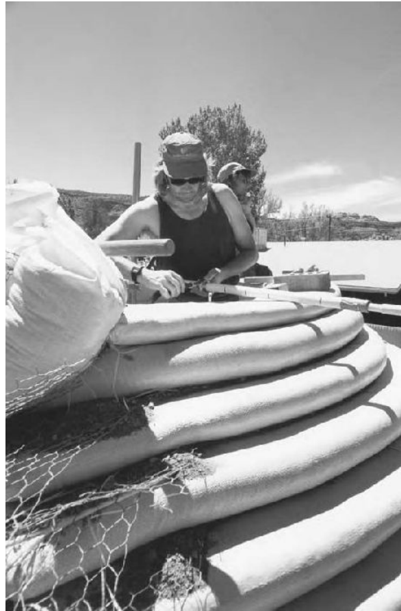
11.21: The further the bags (tubes) are cantilevered over the underlying bags, the more they flatten out.
