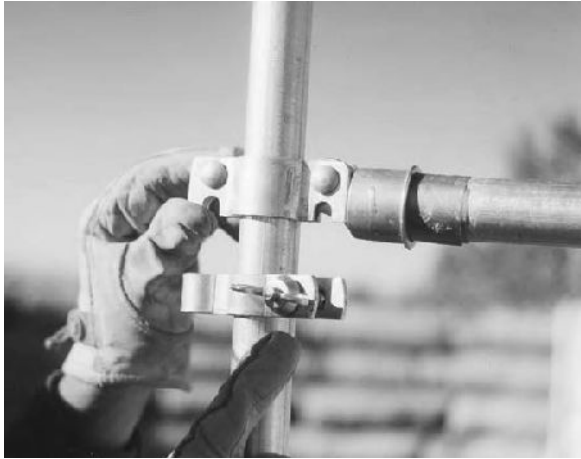
3.43: Compass parts assembled onto vertical post.
