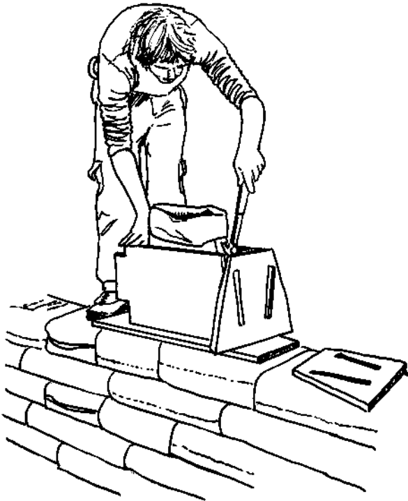
3.21: The ends of the wedge box are removed and the sides drop down for easy removal of the pre-tamped fan bag.
