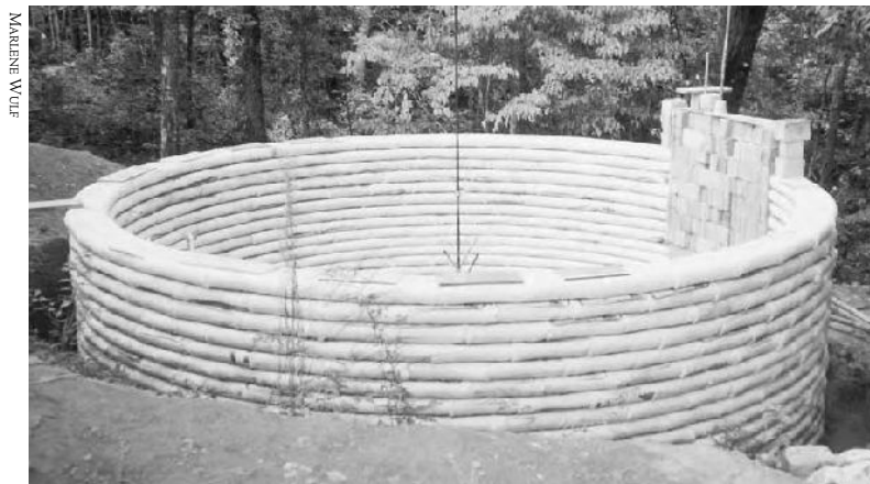
5.7: The ultimate form of buttressing is a complete circle.
