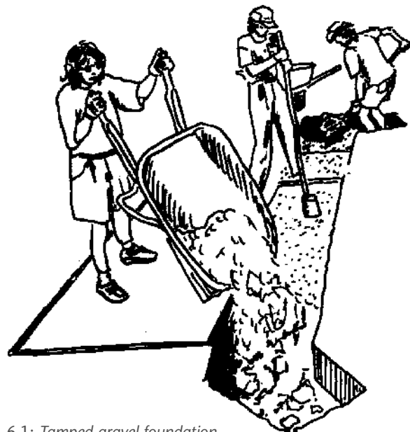
6.1: Tamped gravel foundation.
