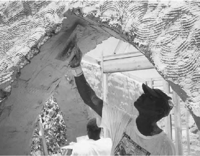
14.18: Applying cement-lime stucco over chicken wire on the Sand Castle on Rum Cay, Bahamas. Photo Credit: Steve Kemble and Carol Escott
