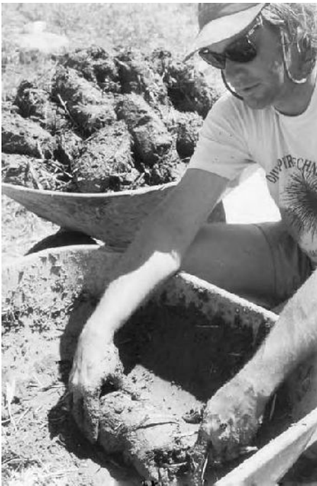
14.12: To mix cob loaves stiffer than the mixer, we throw a chunk of the mix into a wheelbarrow lined with straw and knead it like bread, jabbing the center of the loaves with our thumbs.
