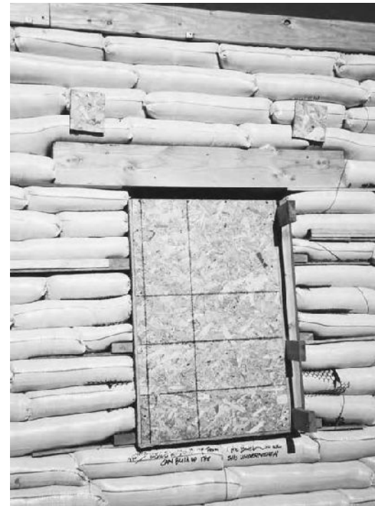
8.2: An example of a lintel pre-attached to Velcro plates that extend another eight inches beyond the ends of the lintel.
