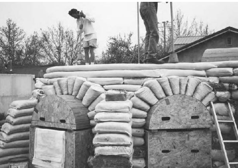
12.22: After tamping, each row should feel as secure as a sidewalk.
