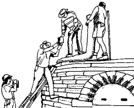
12.27: Laying barbed wire at this height is easiest done with the reel safely located on the ground.
