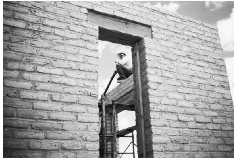
1.3: A freshly laid adobe wall near Sonoita, Arizona.
