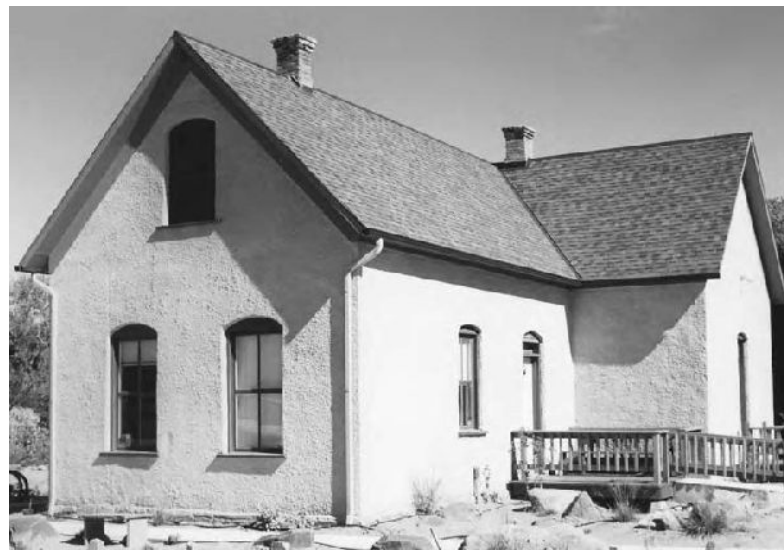
14.17: One-hundred-year-old adobe house protected with a coarse coat of lime plaster.
