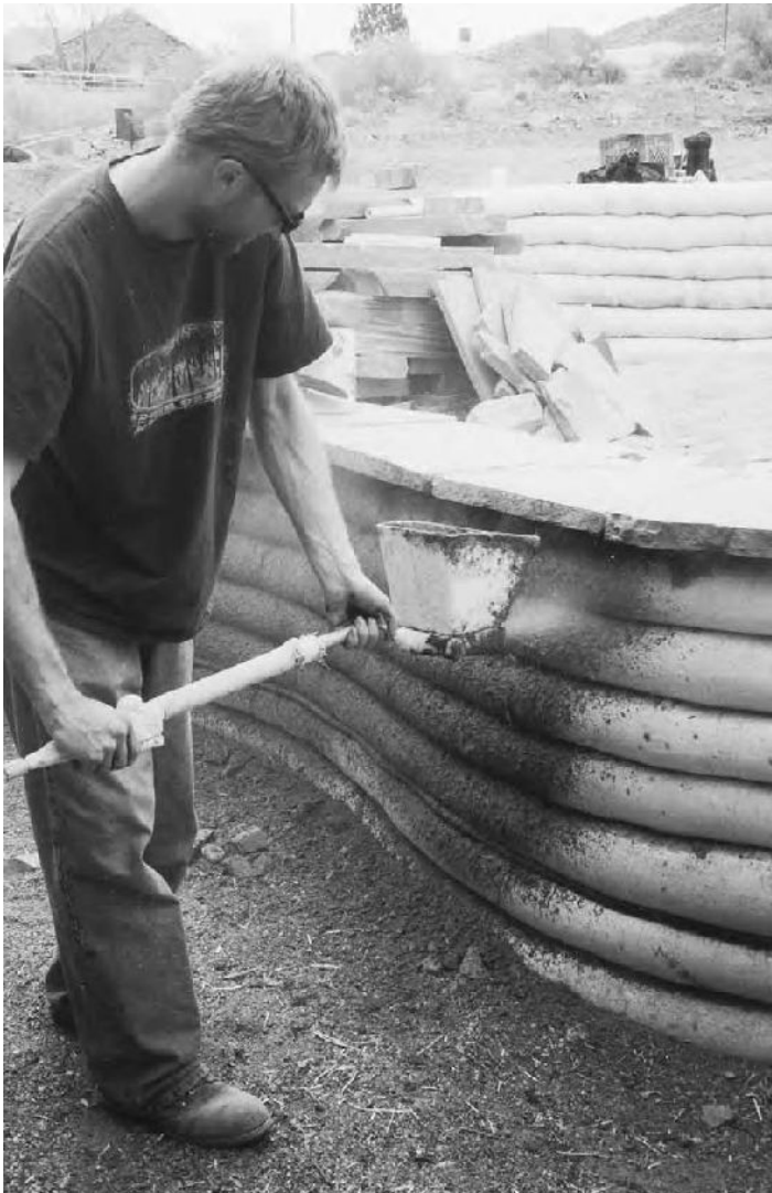
14.9: Shooting mud onto an earthbag wall with a plaster sprayer.
