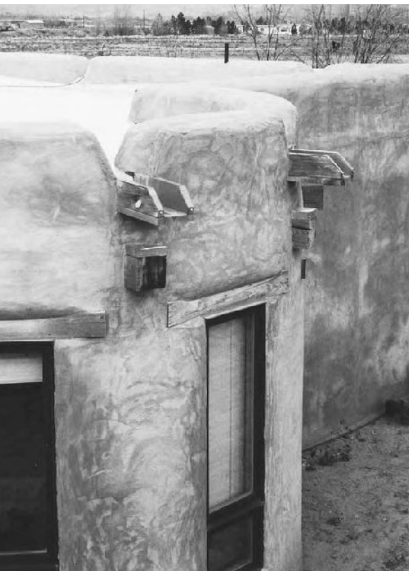
9.14: Flat roof with parapet walls and canales.
