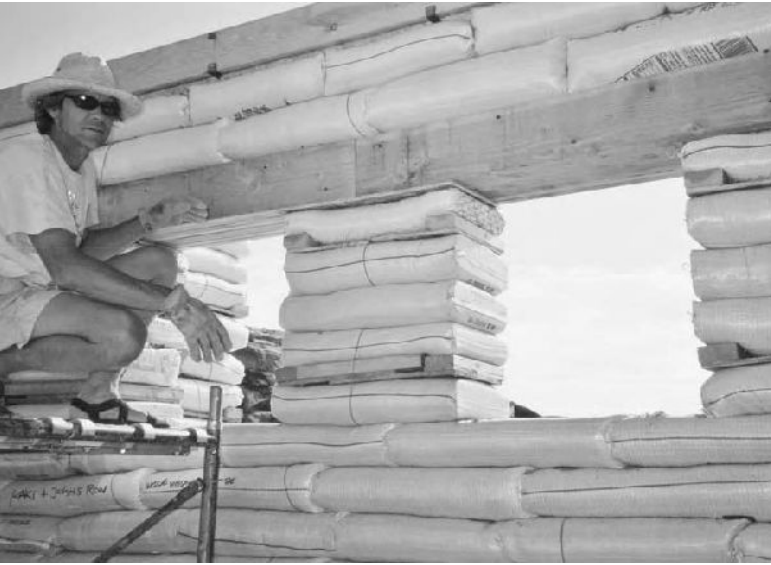
8.3 (above): In designs with multiple windows, they can share Velcro plates or the lintel can span across the top of all the windows.
