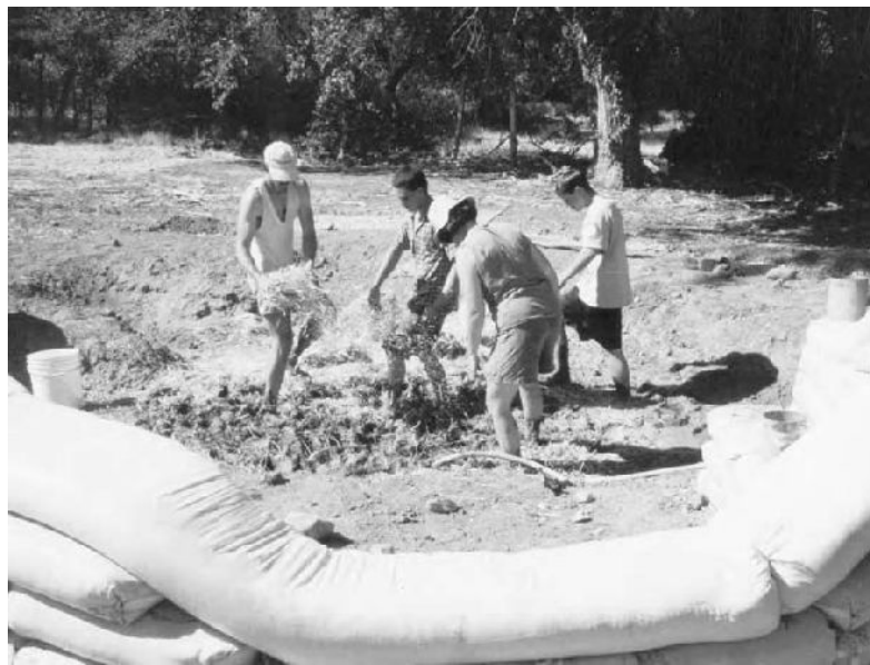
14.6: Presoak the soil in a pit, and add handfuls of straw while stomping around in the muck.
