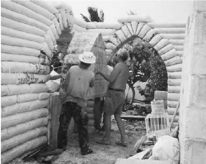
2.23: Arch form being removed from the wall in the Bahamas.
