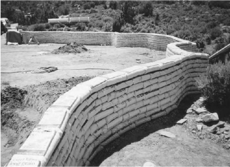
5.4: Sufficiently curved walls are laterally self-supporting.
