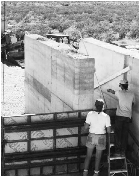
1.6: Rammed earth wall after removal of forms.
