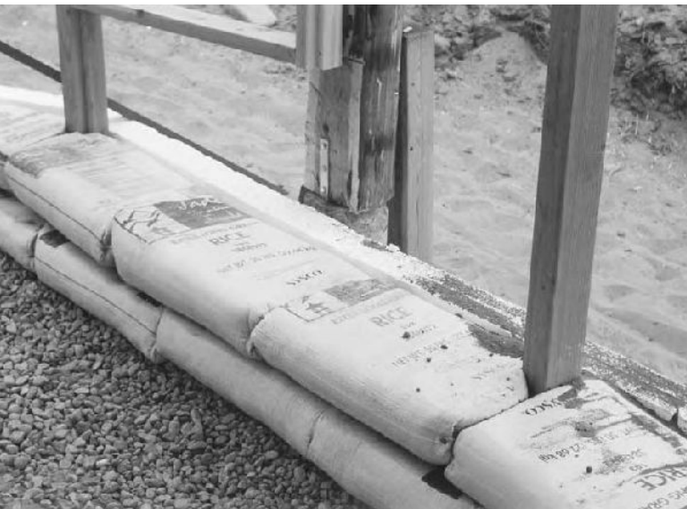
5.16: The second row of bags lock down the Velcro plates and wrap around the posts.
