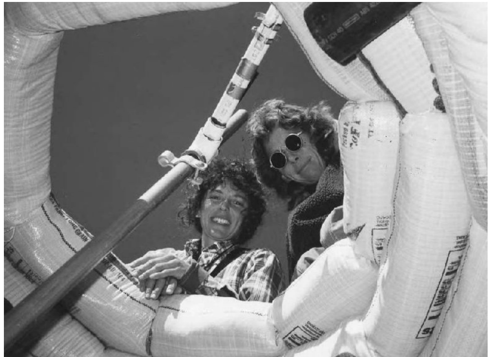
12.29: Providing support for the second-story arch forms may require extra bracing. Note the installation of upper ventilation pipes.
