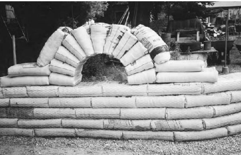
3.18: The fan of an arch.
