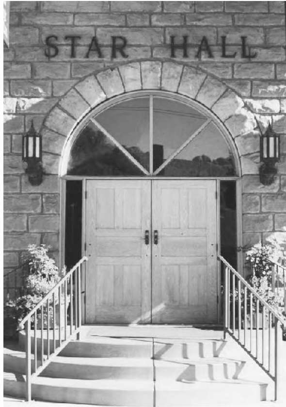
10.4: Built with cut sandstone, this Roman arch (or voussoir) in Moab, Utah, celebrates its 100th birthday.
