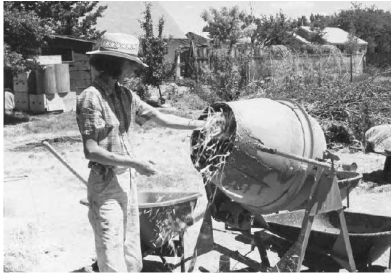
14.5: Adding long straw to a batch of earthen plaster.
