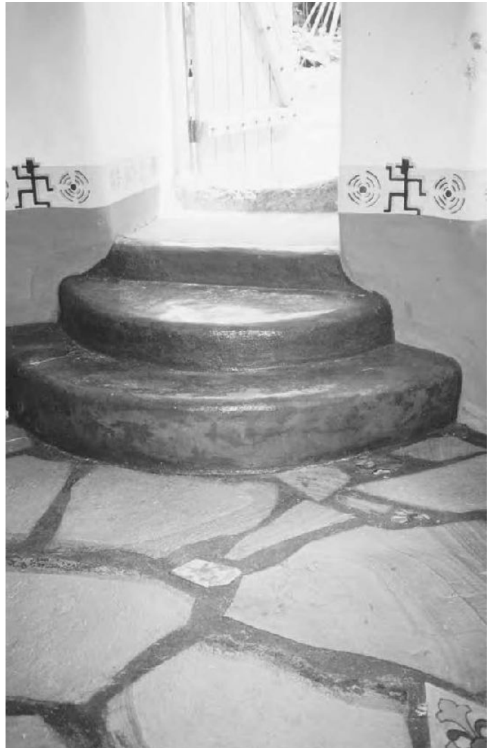
16.8: Mud-mortared flagstone and antique Malibu tiles grace the floor of the Honey House dome.
