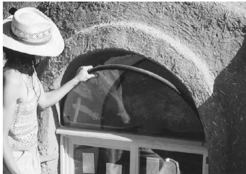
8.6: (Above) Side view detail of vinyl window installation. 8.7: (Right) Split a length of five-eighths-inch (1.56 cm) soaker hose as a gasket over a one-quarter-inch thick plate or thermopane glass that has been pre-cut in a half-round shape.
