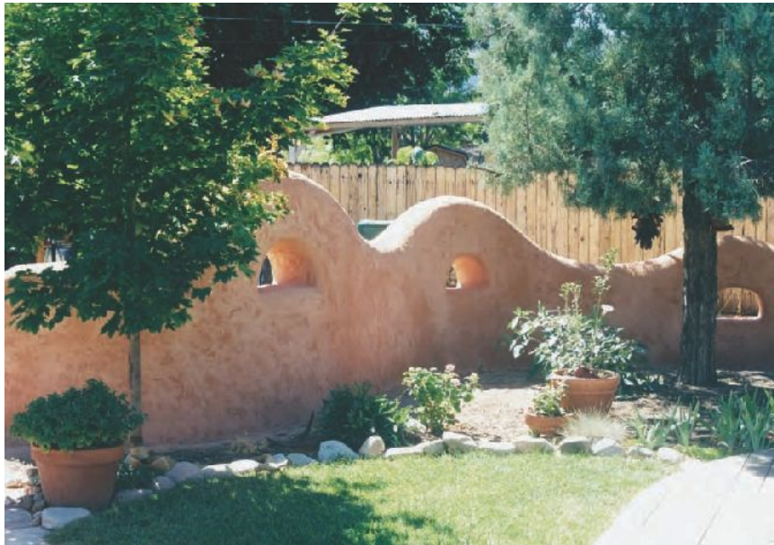
Earthbag walls make attractive sturdy privacy walls, sound, and wind barriers that can be adapted to suit many climates. Mitchell May's 300 yard long earthbag wall is covered with a cement/lime plaster in Castle Valley, Utah (Figs. 12, top and 13, right).
