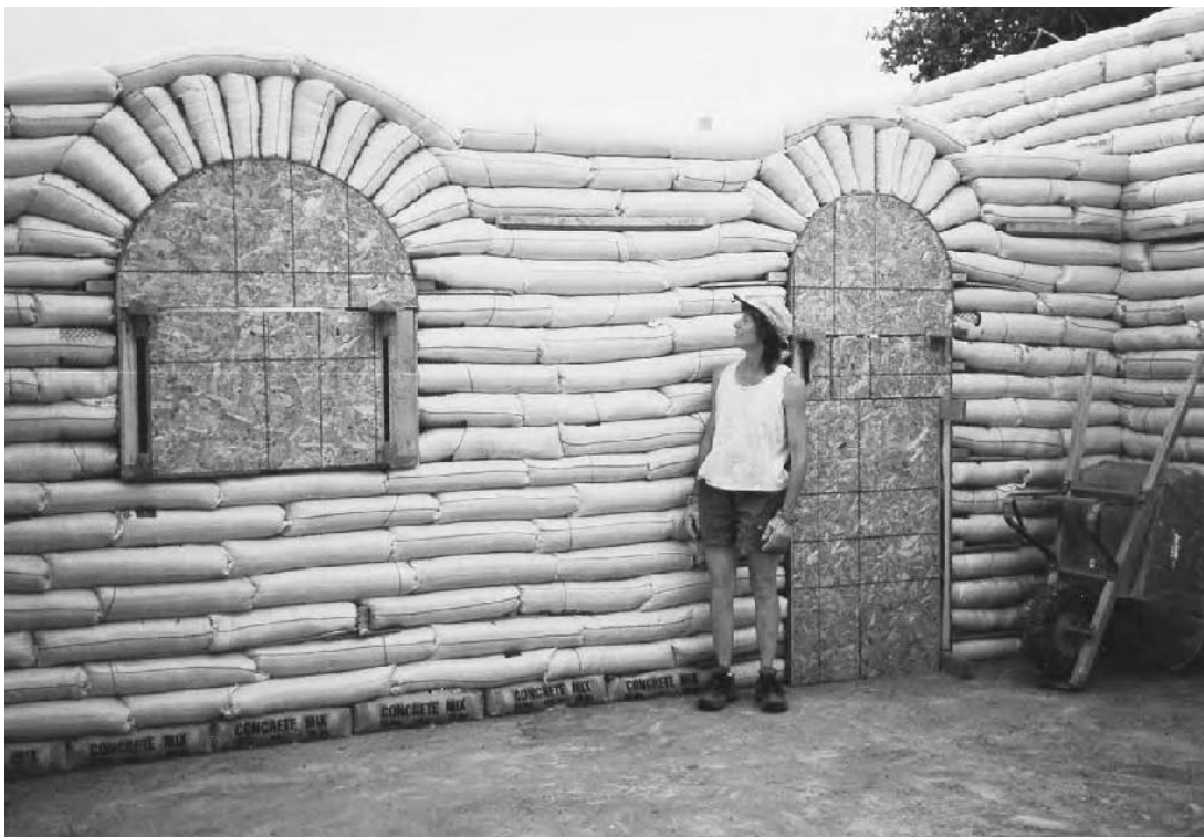
2.22: Rigid form supporting door and window placement.
