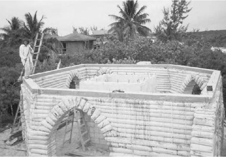
9.2: The bond beam must be continuous, covering the full perimeter of the wall.
