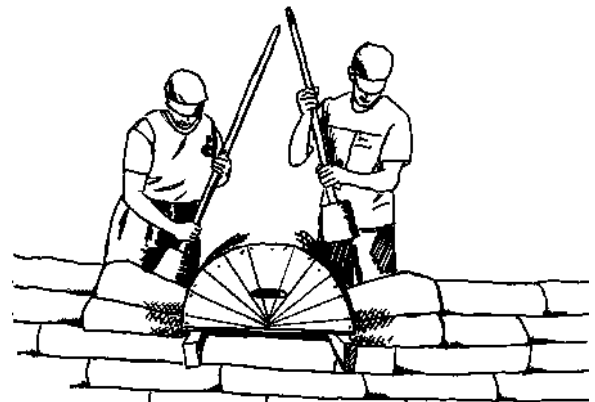
6.58: Shaping the fan bags.
