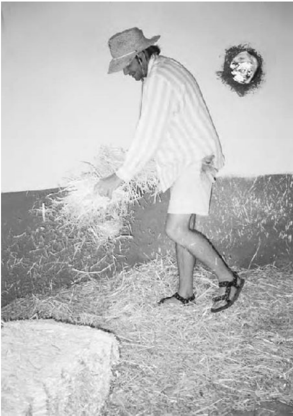
16.4: The loose straw soaks up any extra moisture from the adobe and provides that much more insulation.
