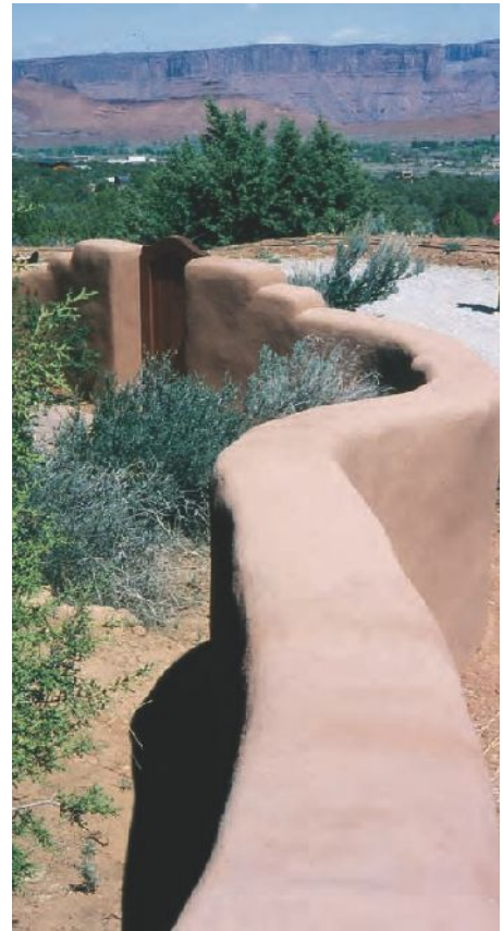
Earthbag walls make attractive sturdy privacy walls, sound, and wind barriers that can be adapted to suit many climates. Mitchell May's 300 yard long earthbag wall is covered with a cement/lime plaster in Castle Valley, Utah (Figs. 12, top and 13, right).
