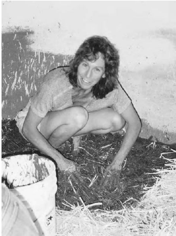
16.5: Mixing a straw-rich adobe insulative layer can be likened to shampooing a big shaggy dog.
