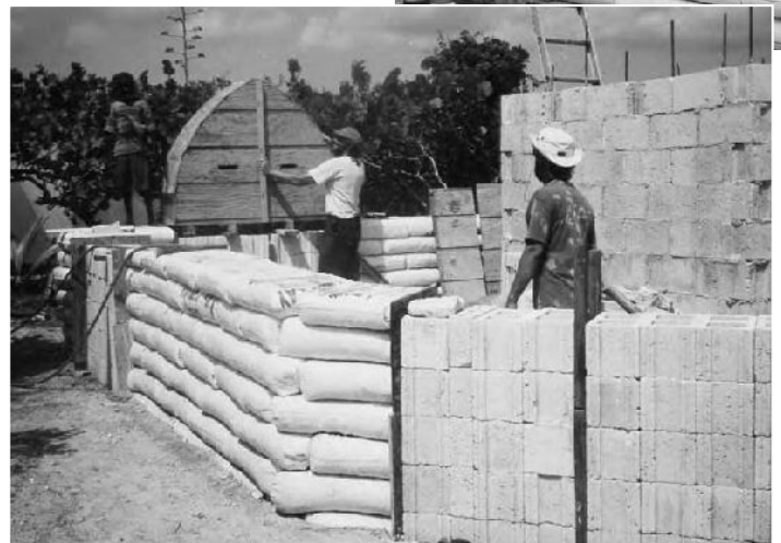
2.27: Cinder blocks work well as temporary door forms.
