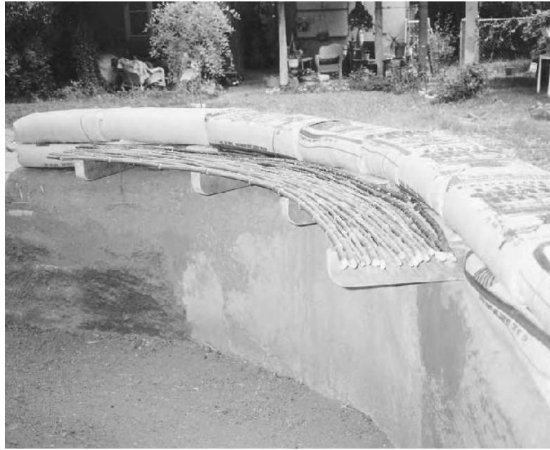
7.12: Shelf brackets on a curved wall sheathed with bamboo and/or saplings.
