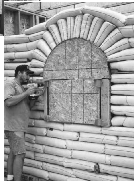
2.26: Split box forms can be adjusted to accommodate various size openings.
