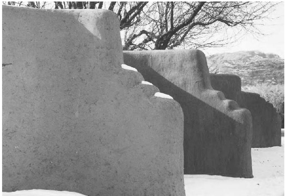
14.1: Earthbag walls with an earthen plaster coat, in mid-winter.
