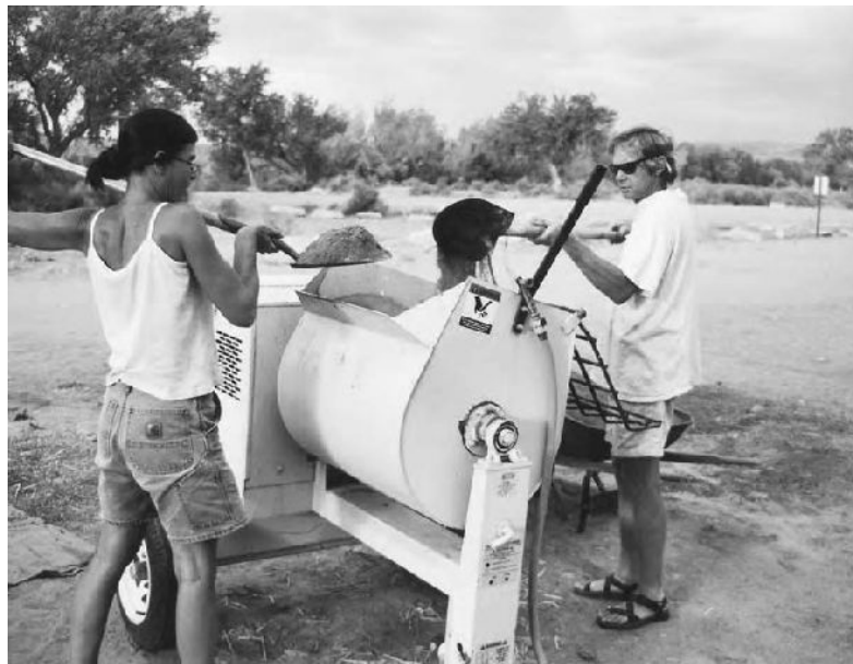
15.3: A mortar mixer makes short work of fat plaster.
