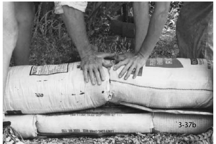
3.37a & b: Kaki and Kay demonstrate closing in a row.
