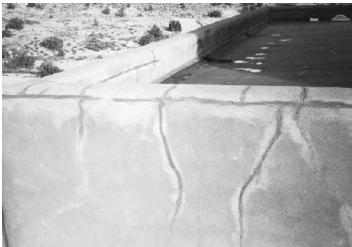
14.19: Even cement plaster over stabilized adobe has continued to crack on the walls of this high-end Southwest-style home.
