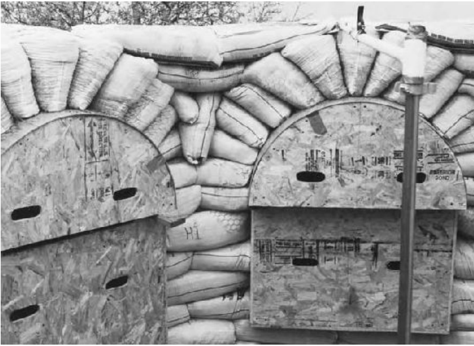
12.21: Placement of the inside edge of the fan bags should be aligned with the compass.
