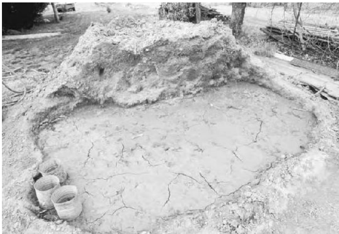
14.3: Softening clay lumps in a mud soaking pit.
