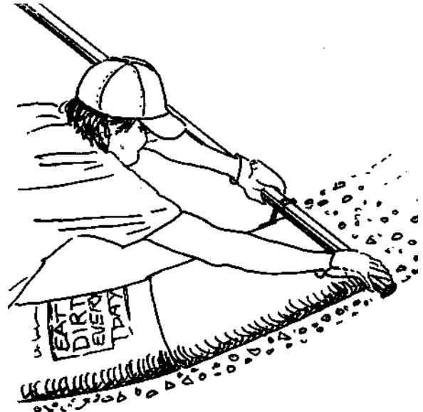
12.7: Use the compass arm to delineate the contour of each bag to conform to the circle.
