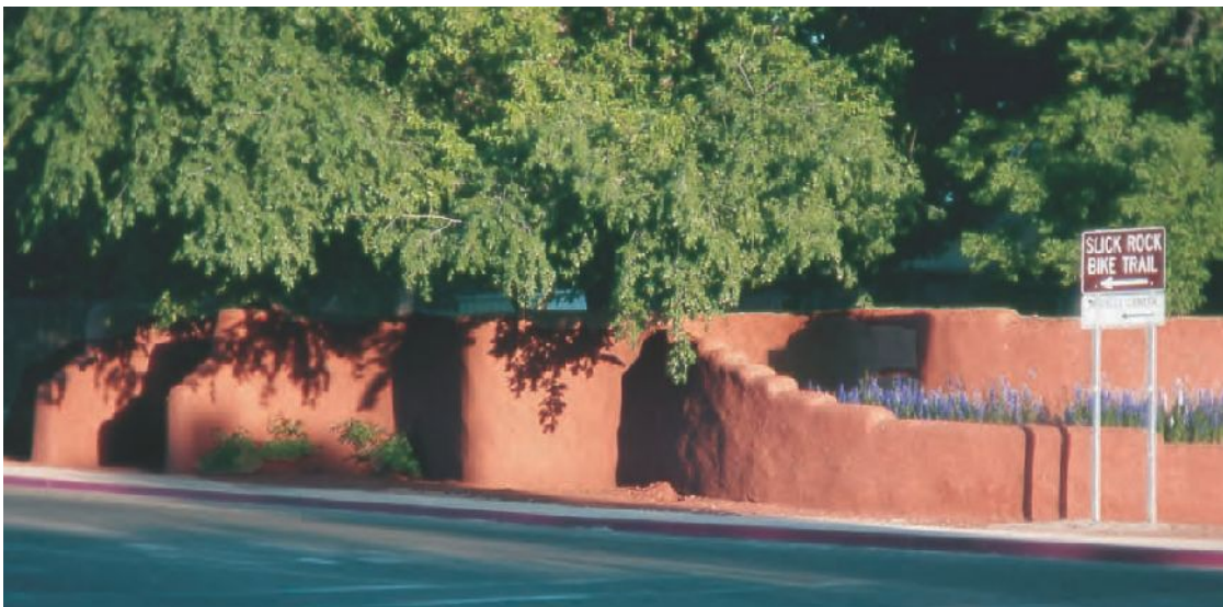
Serena Supplee and Tom Wesson's Earthbag walls built on a busy street corner provide privacy, sound protection, as well as a built-in flower planter. Moab, Utah (Fig. 2, below).
