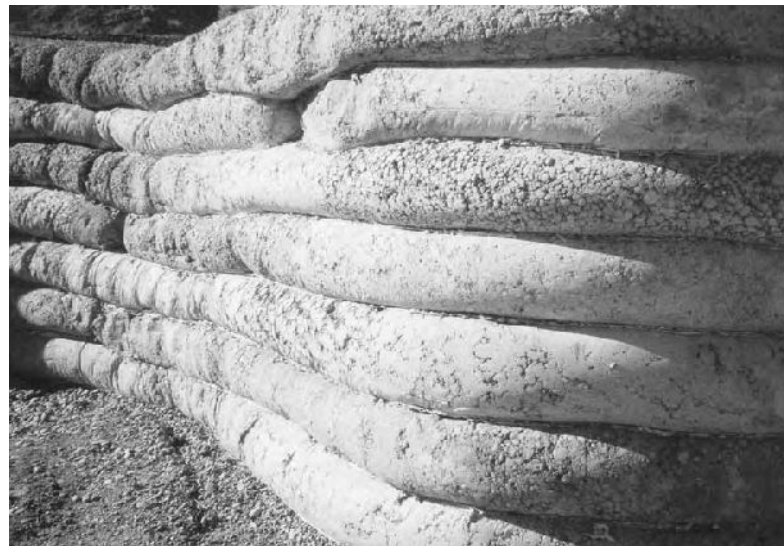
4.7: Because of the lack of tensile strength (e.g. rebar), a continuous tube is more likely to crack in a cold, wet climate, so using tubes would probably work best in a dry or frost-free locale.
