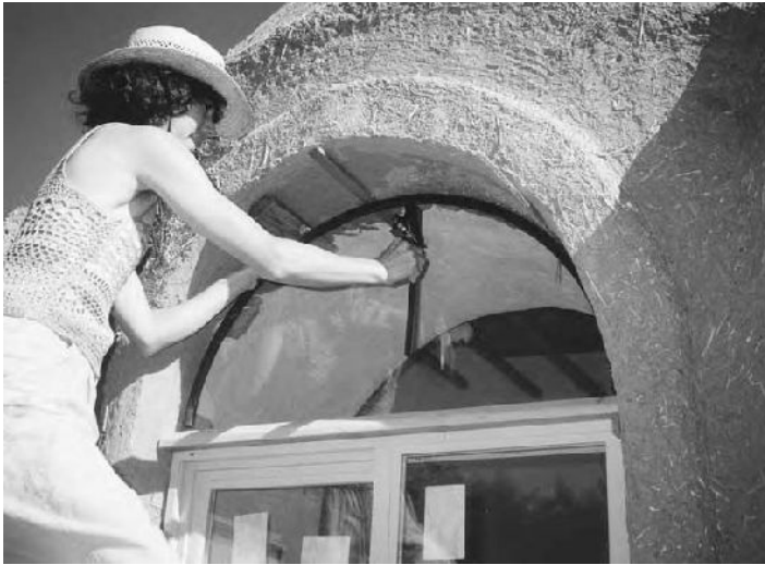
8.8 (left): Install the half-round pane of glass up against the stop that was installed previously on top of the vinyl window. Plumb with a level and secure with shims.
