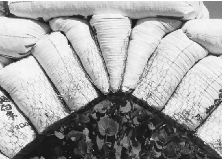
3.23: It is stronger to have too narrow of a gap for the keystones to fit into than one too wide.
