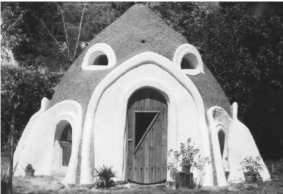
1.1: Using earthbags, a whole house, from foundation to walls to the roof, can be built using one construction medium.
