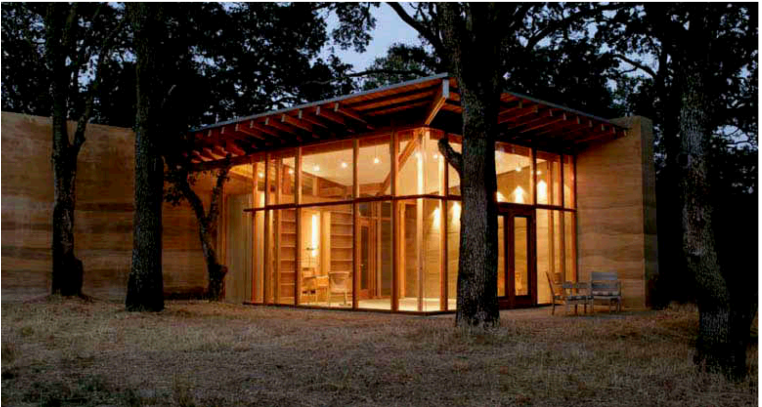
top left: Wood joinery is a counterpoint to the canted rammed earth walls.
