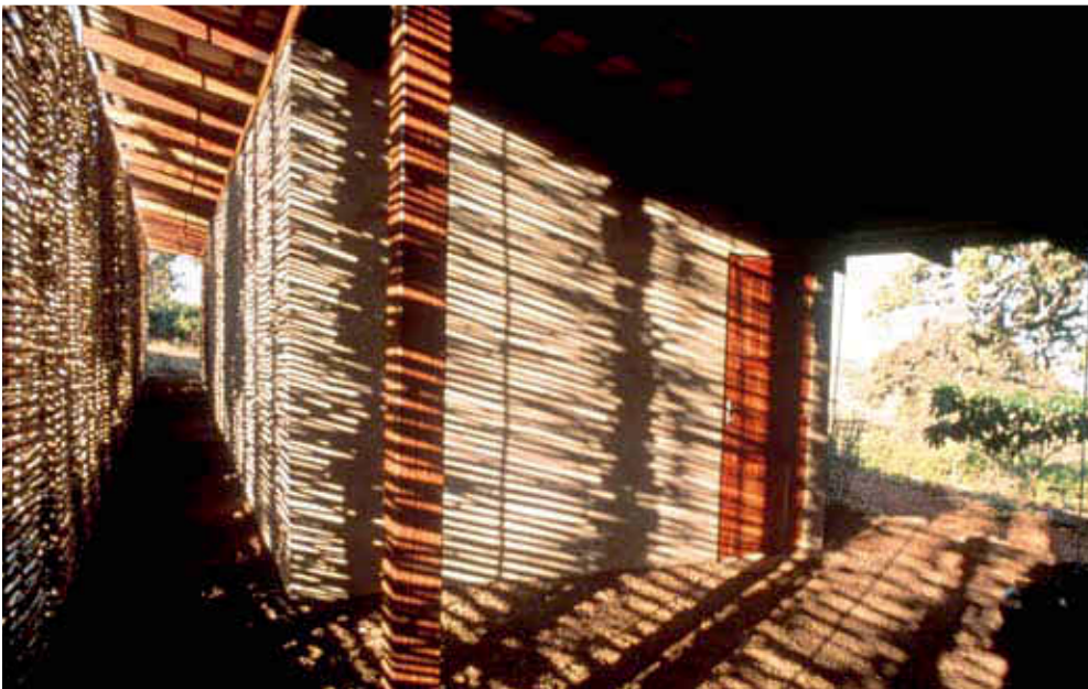
top: The east facade is camouflaged by a woven bamboo screen that blends with the Fouta Djallon highlands in the background.
