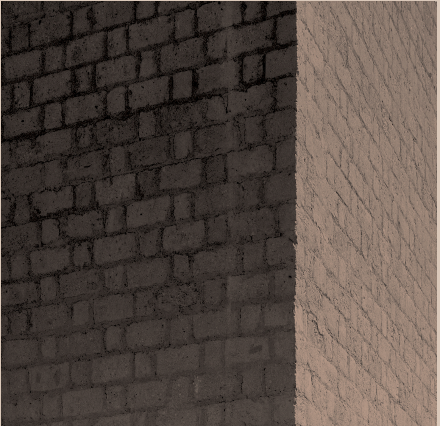
A detail of naturally compressed earth, called tepetate, which was carved from the ground.
