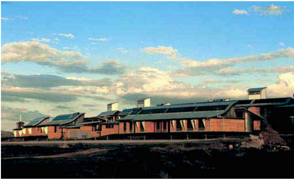
left: Thermal chimneys, which draw out rising hot air, punctuate the roofline of the School of Environmental and Information Sciences.
