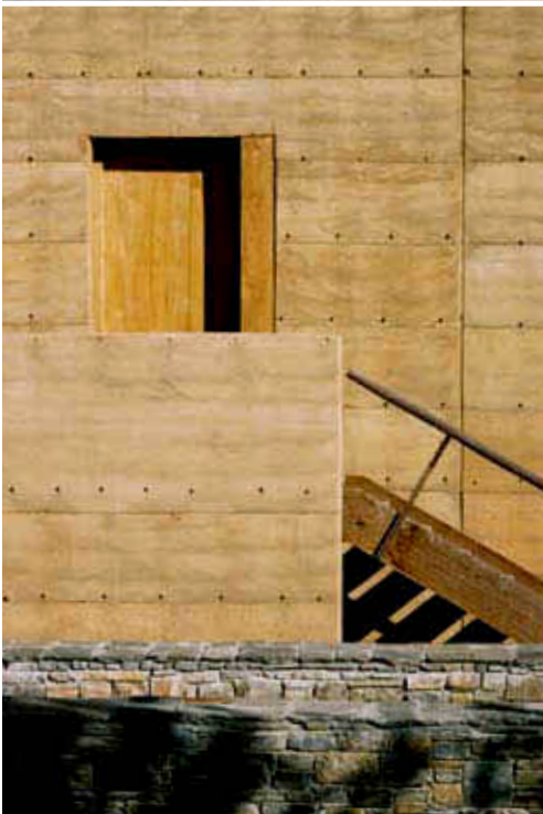
top: Canted rammed earth walls and refined wood detailing are modern takes on a centuries-old Bhutanese building tradition.
