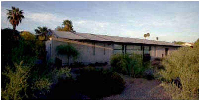
The House of Earth and Light is the first modern residential building with a tensile fabric roof structure.
