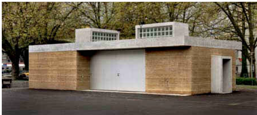
left: The northern toolshed/kiosk is located near the entrance to the grounds.
