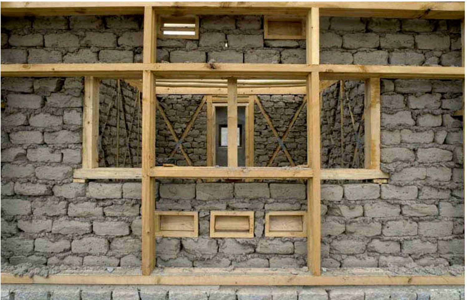
top left: Granite cladding protects the mud brick walls.
