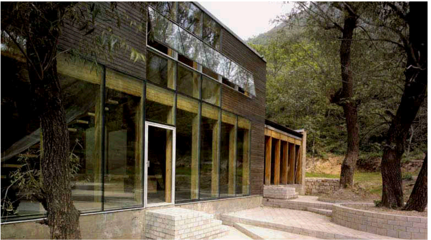
top: The house was split in the center to preserve existing trees and separate the public and private functions of the house.
