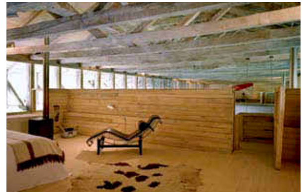
The second-story platform is made of pine flooring; the heavy timber beams original to the building are overhead.
