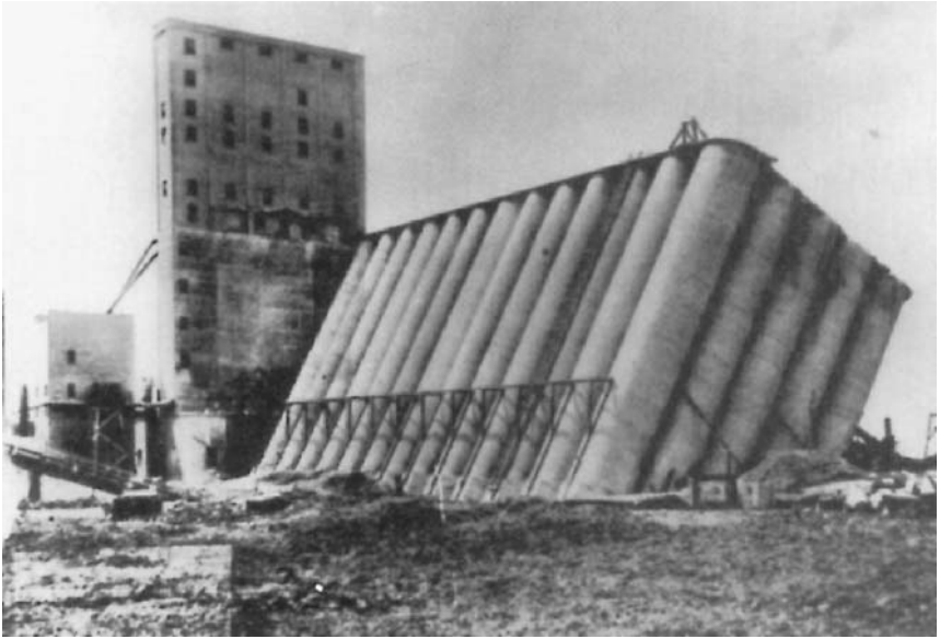
FIGURE 6.27 Transcona grain elevator bearing capacity failure.
