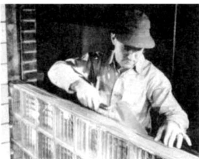
FIGURE 11.15 (Top left) First step in installation of a glass-block panel is to coat the sill with an asphalt emulsion to allow for movement due to temperature changes. Continuous expansion strips are installed at side and head jambs. (Top right) Blocks are set with full mortar joints. (Bottom left) Welded-wire ties are embedded in the mortar to reinforce the panel. (Bottom right) After all the blocks are placed, joints tooled to a smooth, concave finish, and the edges of the panel calked, the blocks are cleaned.
