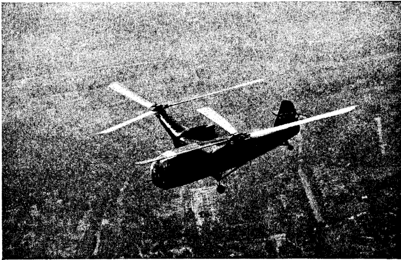
Fig. 2-4 McDonnell XHJD-1 side-by-side helicopter. Courtesy McDonnell Aircraft Corporation.
