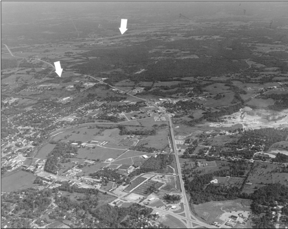
Figure 24-4. Lewisburg, with the quarry on the northeast edge and the airport seen off to the north of town (arrow). You'd see on the actual cross-country that a railroad runs through the western edge of the town (photo arrow and chart).
