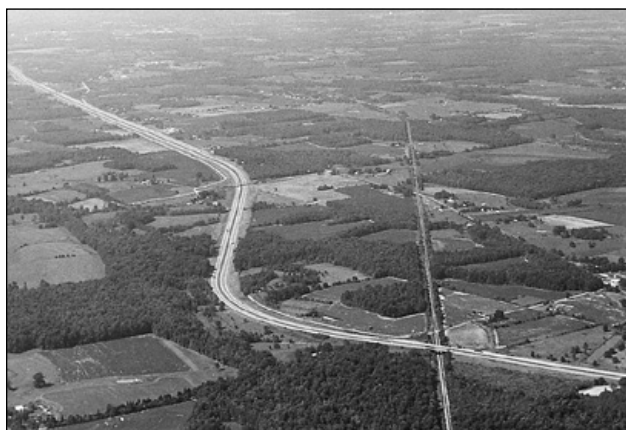
Figure 24-11. Over the railroad after crossing the interstate. Athens (Alabama) is 7 miles south-southwest.
