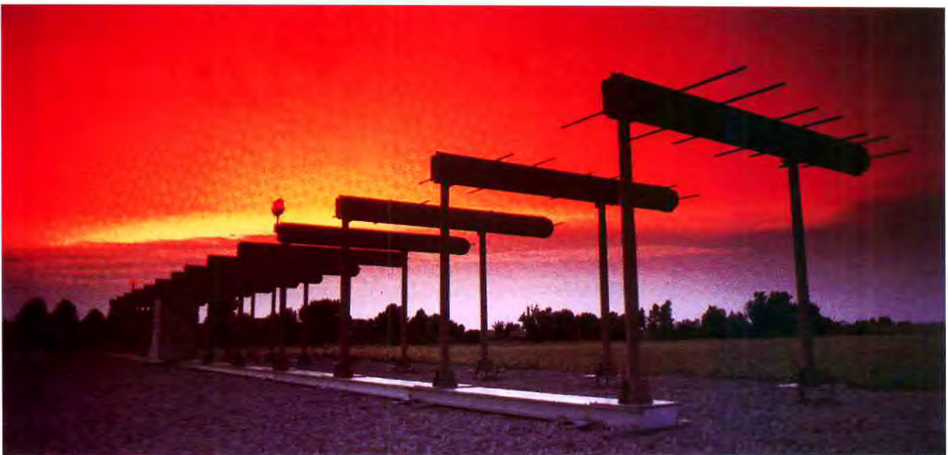
An array of antennas launches the localizer signal near the end of an ILS runway. The beams are pointed toward an airport runway at the right and reach out to about 50 miles.
