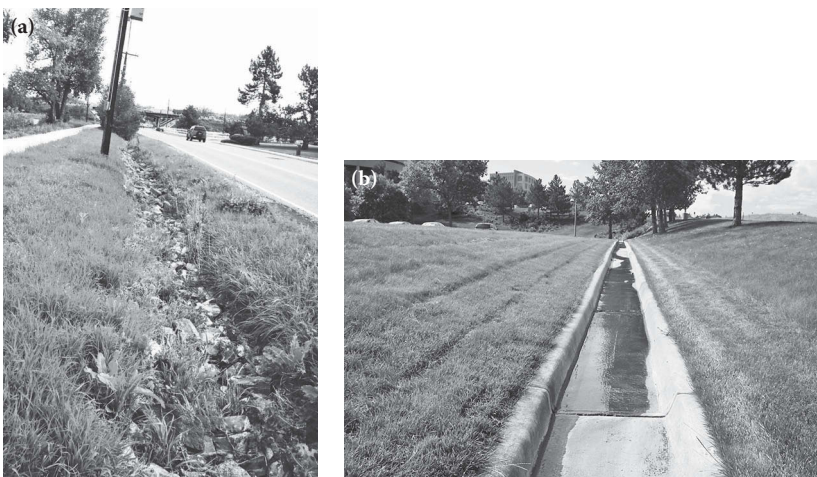
Figure 1.5 Street conveyance system. (a) Grass swale as roadside ditch and (b) trench for flow collection.
