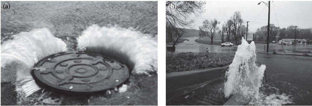
Figure 12.8 High pressure buildup in sewer line. (a) Pressurized manhole and (b) pressurized inlet.
