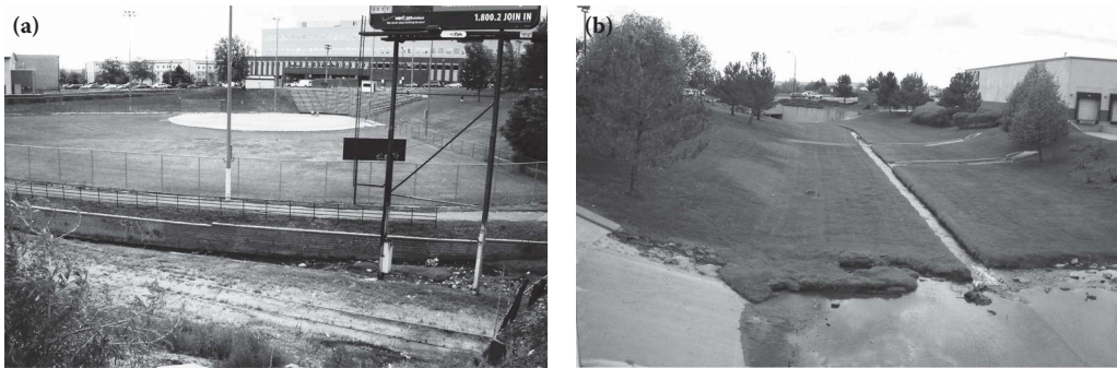
Figure 13.5 Offstream and onstream detention basins. (a) Offstream detention basin (sport field) and (b) onstream detention basin (floodplain).
