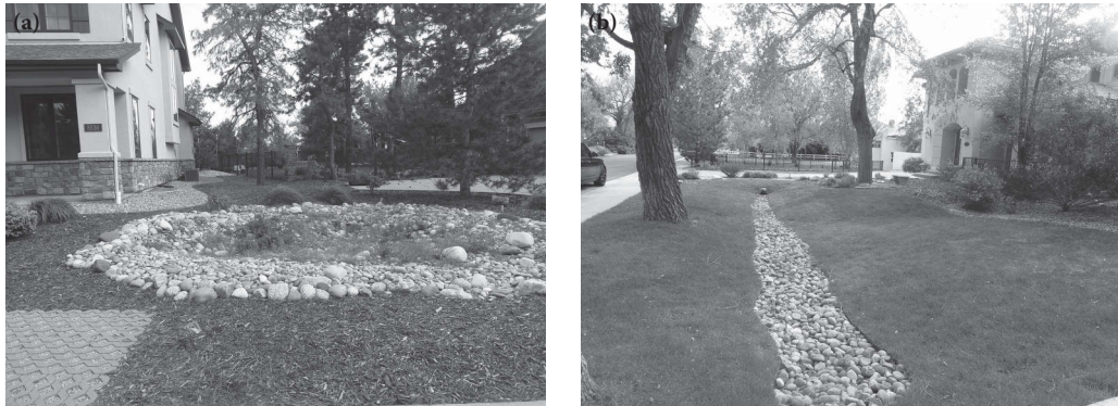
Figure 17.2 Examples of LID designs. (a) Rain garden and (b) infiltration swale.
