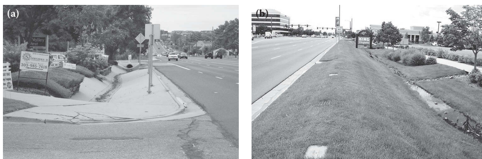
Figure 1.4 LID facilities blended into street drainage system. (a) Streets without LID concept and (b) streets with LID concept.
