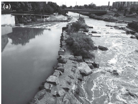
Figure 7.23 Public safety on and along urban floodplains. (a) Vertical and sloping composite drop and (b) trail between high banks without exit.
