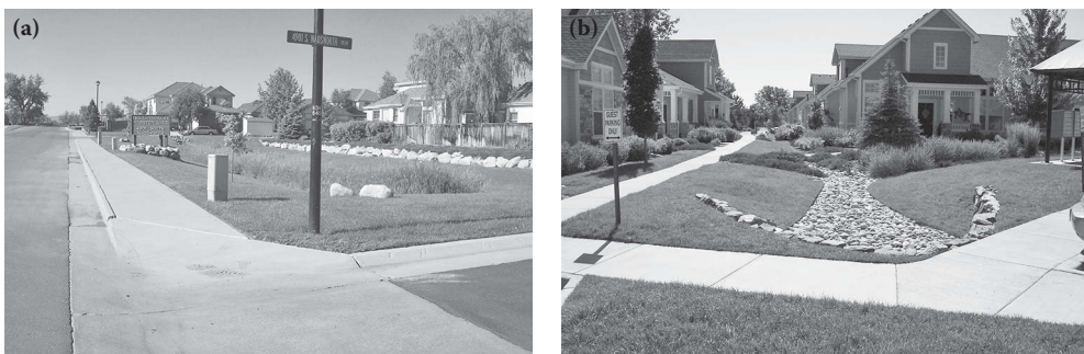
Figure 1.10 Example for WQCB. (a) WQCB at the outfall point and (b) LID units as runoff source control.
