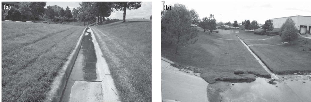
Figure 7.18 Examples of trickle channel. (a) Concrete trickle channel and (b) grass trickle channel.
