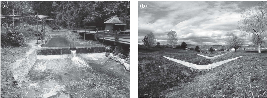
Figure 7.2 Drop structure for grade control. (a) Drop built on natural waterway and (b) drop across grass channel.
