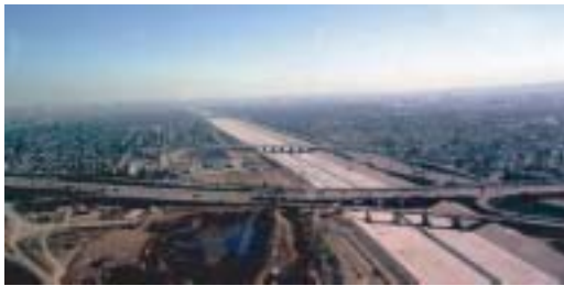
Figure 4.39 Los Angeles River and roadway crossings.
