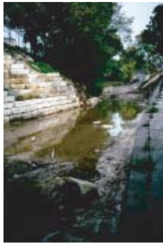
Figure 3.8 Lined embankment along Waller Creek, Austin, TX.
