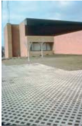
Figure 3.15 Paver blocks for emergency and utility vehicle access, Madison, WI (under construction).
