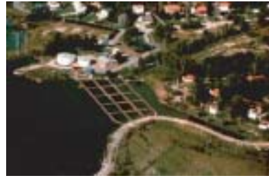
Figure 4.24 FBM installation located at Lake Trehormingen, Sweden. (Used with permission of Fresh Creek Technologies, Inc.)
