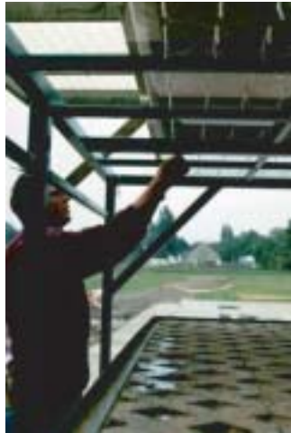
Figure 6.33 Adjustments being made to rain drop tubes at Essen infiltration test apparatus.
