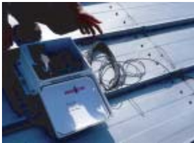
Figure 6.55 Rooftop temperature data logging used by WI DNR.
