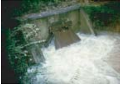
Figure 4.44 Five-Mile Creek SSO discharge during large flow.
