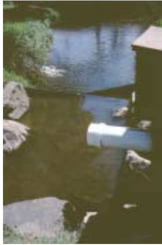
Figure 4.19 Stilling well at Bellevue flow monitoring station.
