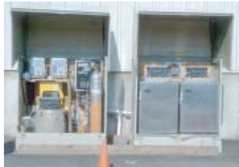
Figure 5.26 .Multiple flow monitor and sampler setup for simultaneously monitoring influent and effluent over wide range of flow conditions at a small treatment device in Madison, WI.
