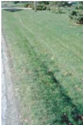
Figure 3.17 Grass swale in residential area, Milwaukee, WI.
