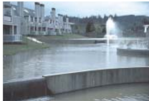
Figure 2.16 Stormwater pond adding value to apartment complex (Lake Oswego, OR).
