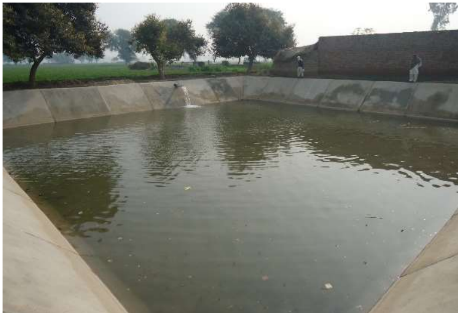
Fig.3.16 Water Storage Tank (20 × 20 × 2 m) for drip irrigation system
