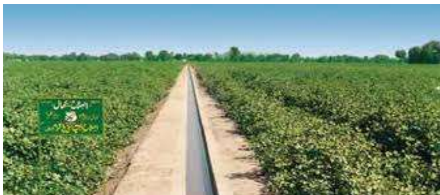
Fig.1.18 A Brick Lined Rectangular Watercourse
