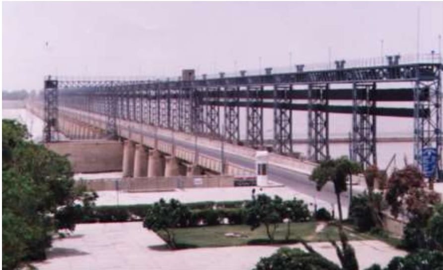
Fig. 1.11 Taunsa Barrage on River Indus
