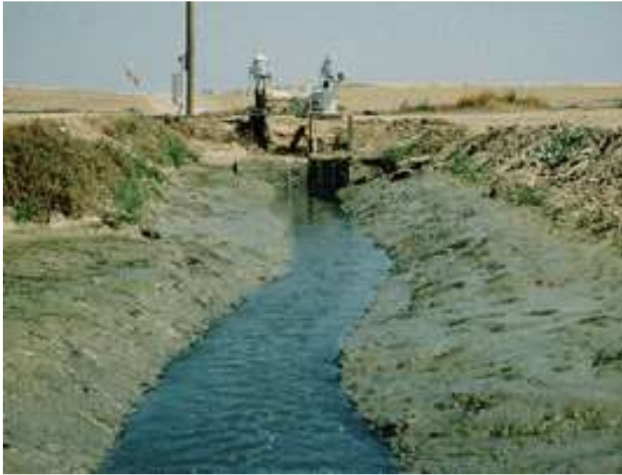
Fig. 7.2 Surface Drain at Khan Garh, Distt. Muzaffer Gardh, Pakistan
