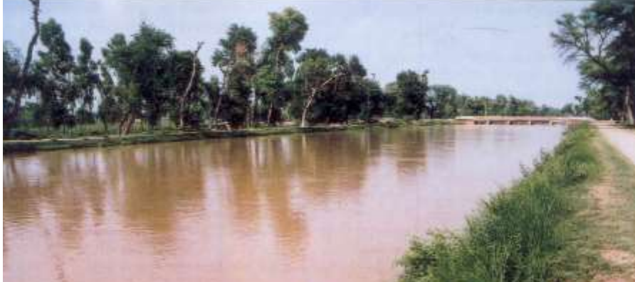
Fig. 1.13 A Typical Main Irrigation Canal in Sargodha
