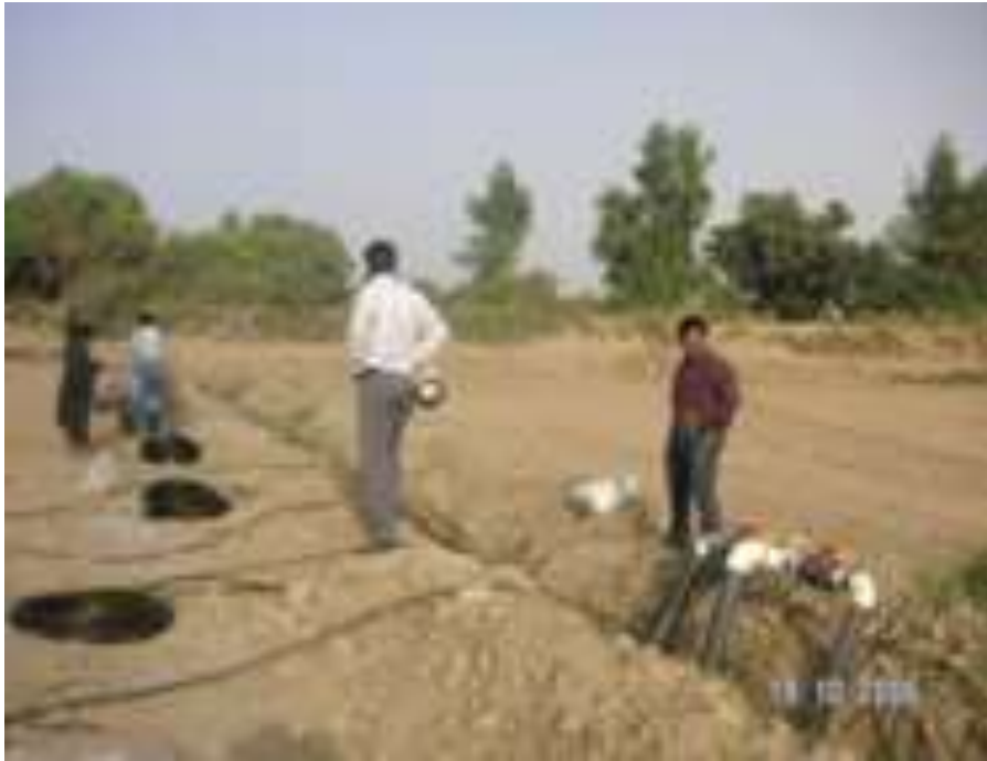
Fig. 3.15 Installation of Drip System in progress (LBDC Project)
