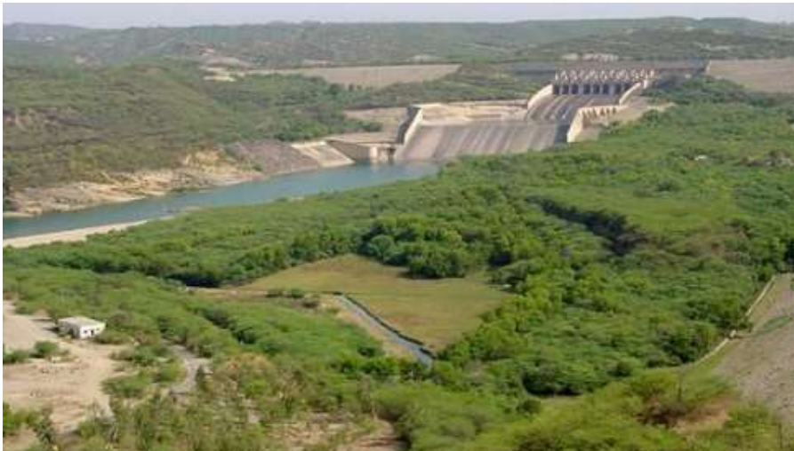
Fig. 1.9 Mangla Dam in Pakistan
