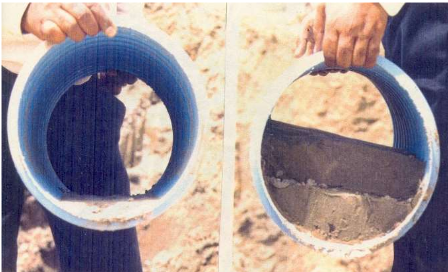
Fig. 7.12 Sediment Settling in the pipe drains at FDP, Faisalabad
