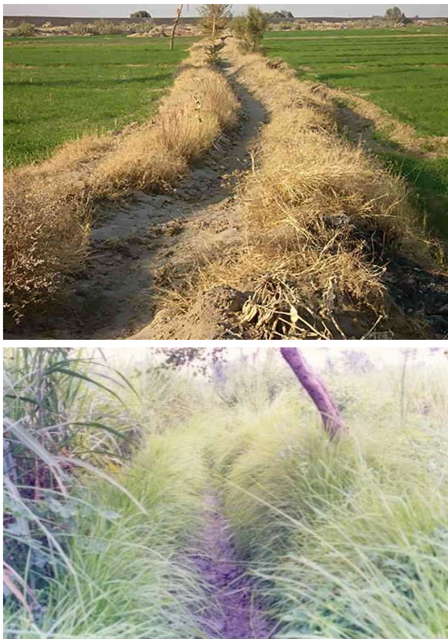
Fig. 1.15 Examples of Unimproved and Poorly Maintained Watercourses
