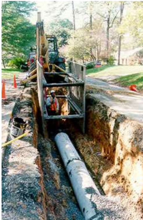
Fig. 7.9 Laying of Pipe Drainage System
