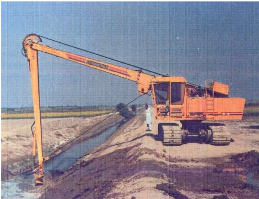
Fig. 7.5 Cleaning and Maintenance of Surface Drain at FDP, Faisalabad
