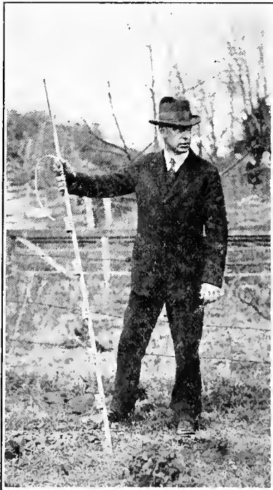
CHARGE WITH PRIMER ON LATH FOR BLASTING A DEEP POLE HOLE
