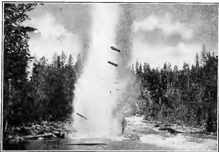
BLASTING OUT A LOG JAM WITH DU PONT DYNAMITE AT BIG FORK, MONT.
