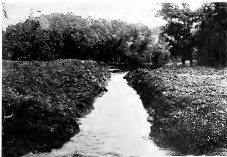
ANOTHER BLASTED DITCH
