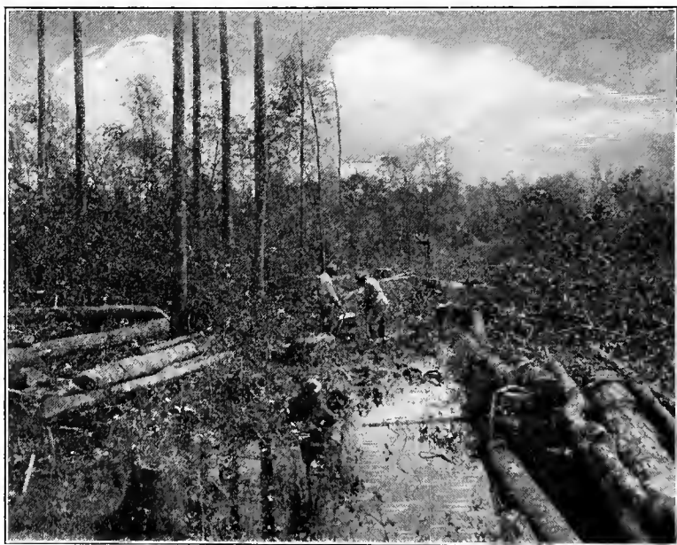
LOADING THE DITCH
