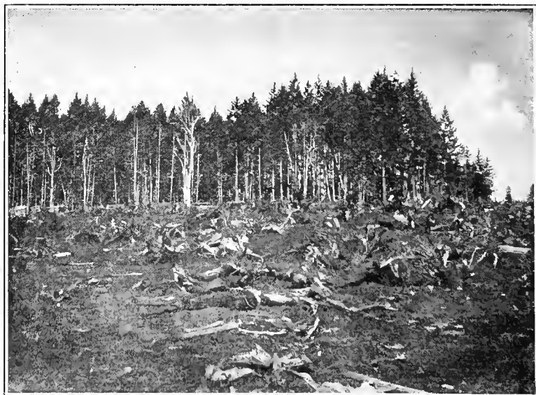
GENERAL VIEW OF BLASTED STUMP FRAGMENTS ON LIGHT CLEARING
