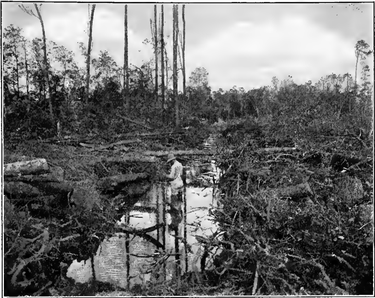
THE FINISHED DITCH
