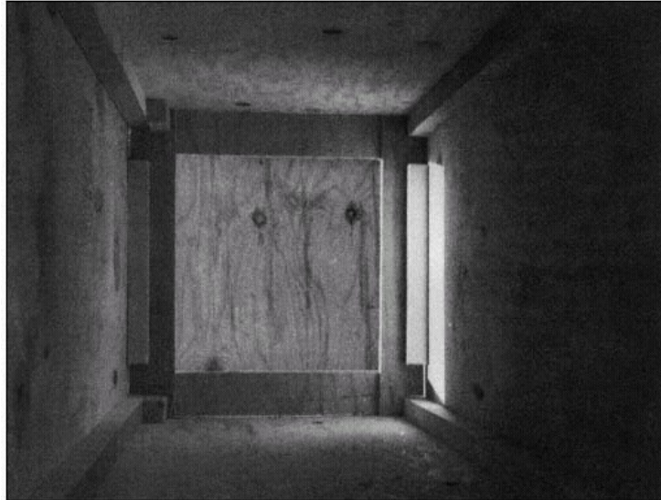
This is a quail's eye view of the tower looking up from the bottom toward the resting shelves and showing the simple 2-by-2 and plywood construction.
