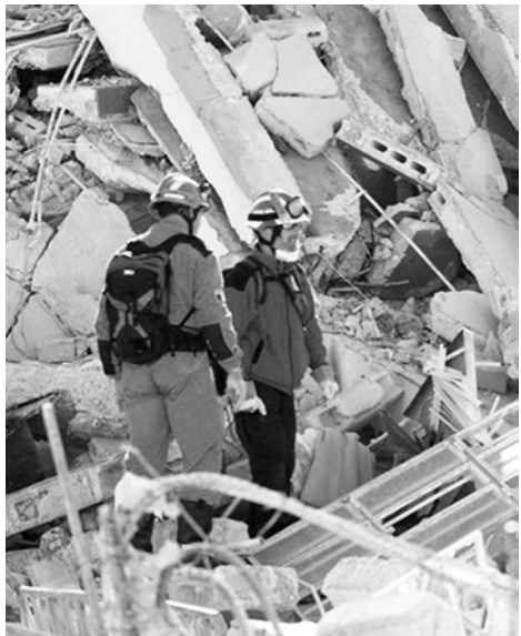
Figure 11.21 “With layers pressed” room. (Haiti, 2010)
