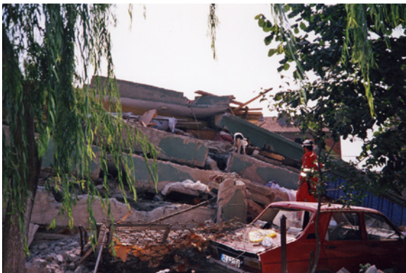
Figure 10.36 The concrete layers are so close together that we hardly dare to think of survivors.
