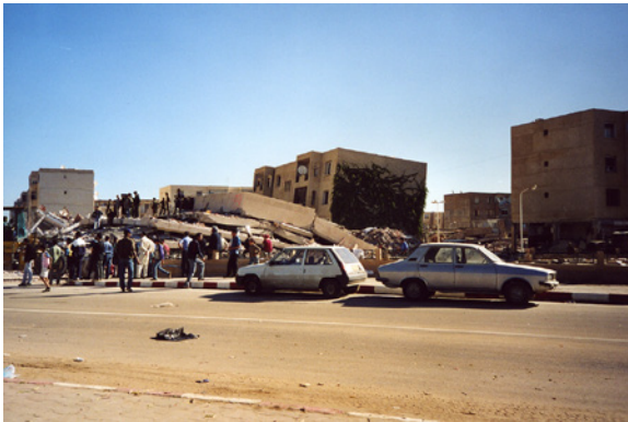
Figure 11.33 Horizontal layers. (Beaumerde, Algeria, 2003)
