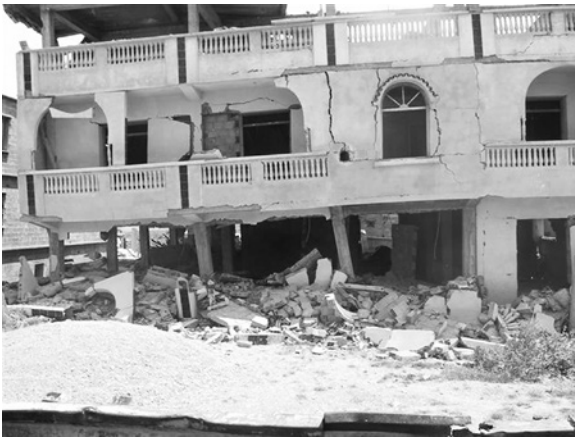
Figure 11.24 Chipped rooms. (Algeria, 2003)
