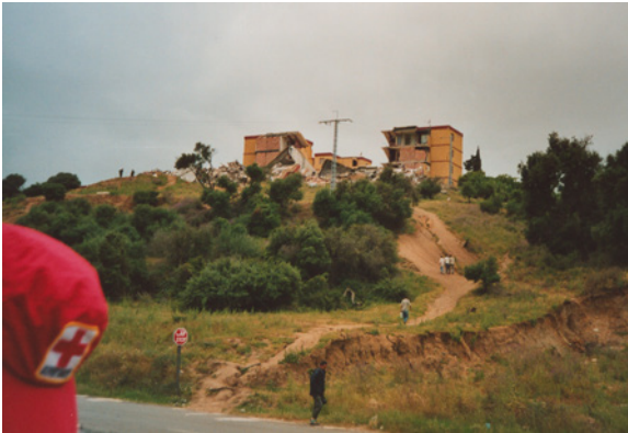
Figure 11.4 Damage crater. (Algeria, 2003)
