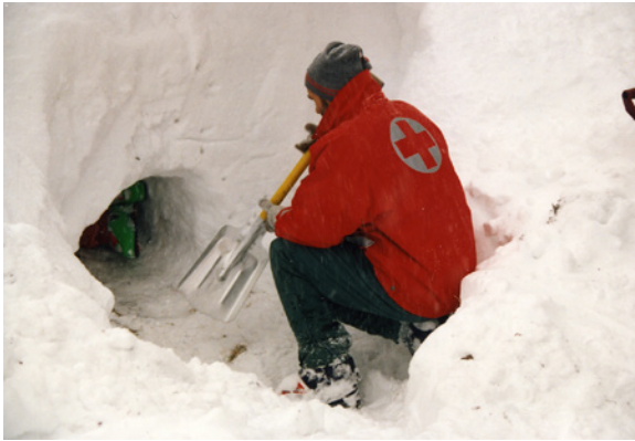
Figure 12.5 Make a twenty by thirty-six inch (50 cm x 100 cm) cylindrical entrance. Then dig an arched cavity measuring about thirty-six inches (1 m) in diameter and thirty inches (75 cm) high.
