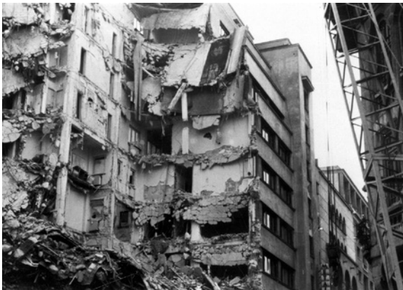
Figure 1.8 After the earthquake in the Romanian capital of Bucharest on March 4, 1977, search and rescue dog teams successfully searched in the partially collapsed reinforced concrete frame and masonry wall offices and apartment buildings.
