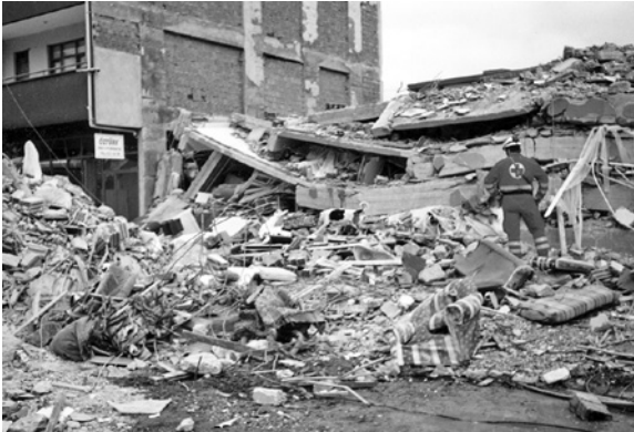
Figure 11.36 Debris cone. (Izmit, Turkey, 1999)
