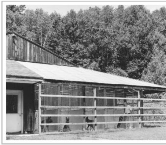
East side view of New Skete's puppy kennel. These are the secure runs for older pups and the German shepherds being bred. The horizontal purlins are to hold a clear poly cover to protect from winter wind and snow.
