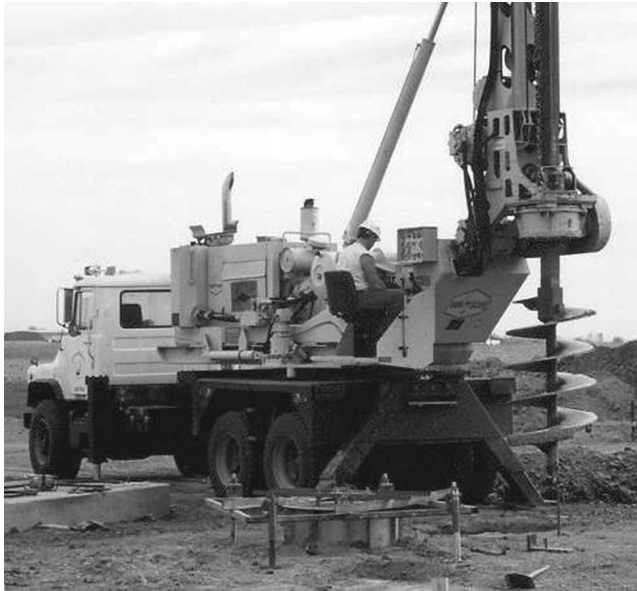
Figure 3.26 Watson 2100 truck-mounted auger drill.
