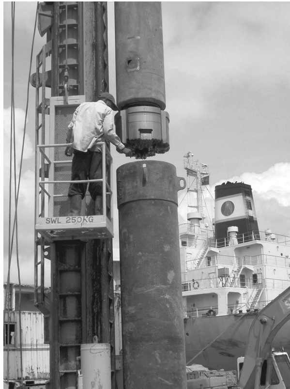
Figure 3.33 Numa hammer with extending under-reaming drill bit for simultaneously drilling and inserting casing. (Courtesy of Numa Hammers, Thompson, CT.)
