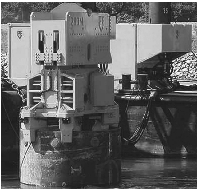
Figure 3.14 Driving a pile casing with a PVE 200 m free hanging vibrator.
