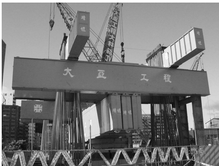
Figure 11.10 Patented arrangement for a 5800 tonne static load test.
