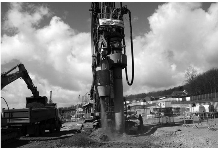
Figure 3.35 Self-erecting drill rigged for installing cased CFA piles with telescopic spoil chute. (Courtesy of Bachy Soletanche Ltd, Ormskirk, UK.)
