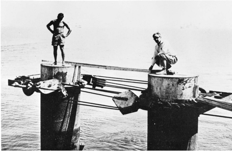
Figure 11.22 Lateral loading test on two steel tubular piles forming part of a breasting dolphin.
