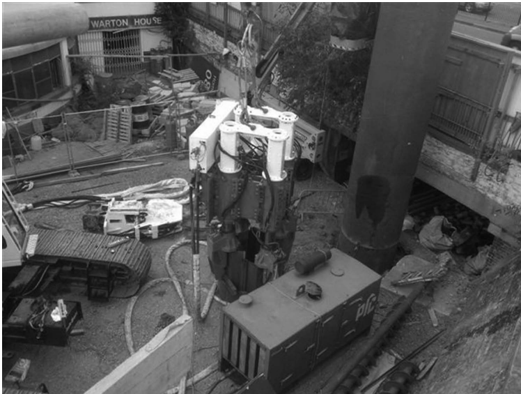
Figure 3.20 Crane-suspended push-pull piler. (Courtesy of Dawson Construction Plant Ltd, Milton Keynes, UK.)
