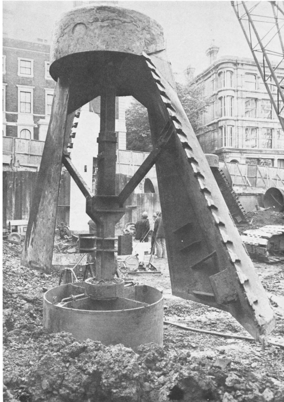
Figure 3.30 Top-hinged under-reaming bucket.
