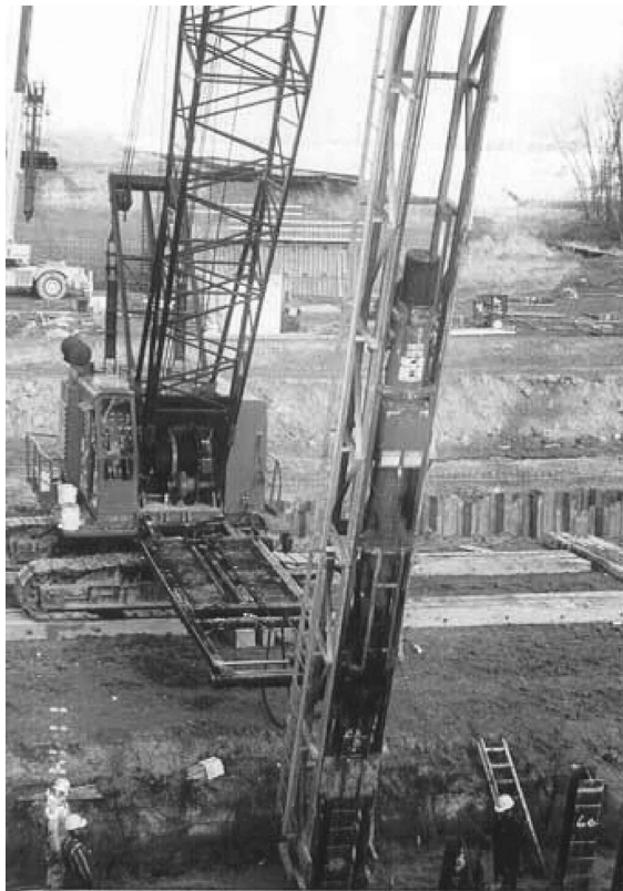
Figure 3.13 Delmag D30-20 diesel hammer on American-style leaders with helmet for driving steel H-piles.
