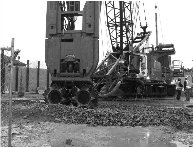
Figure 3.38 Hydromill for forming barrettes. (Courtesy of Sound Transit, Seattle, WA.)
