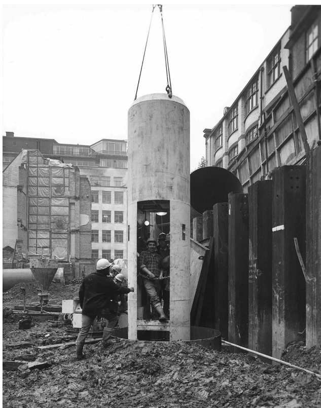
Figure 11.6 Safety cage used for inspection of pile boreholes.
