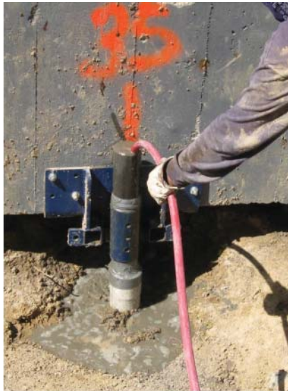
FIGURE 12.13. Installation of micropile during grouting.
