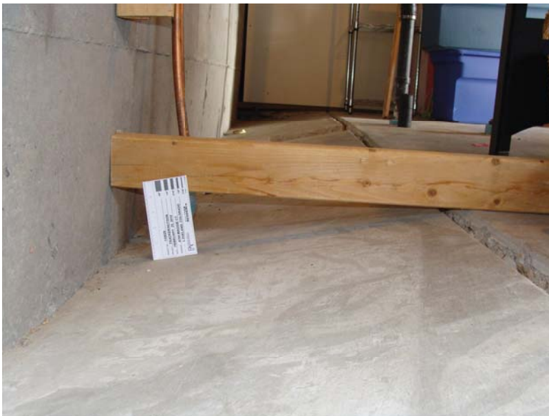
FIGURE 9.7. Basement concrete slab for Very High RF Site.
