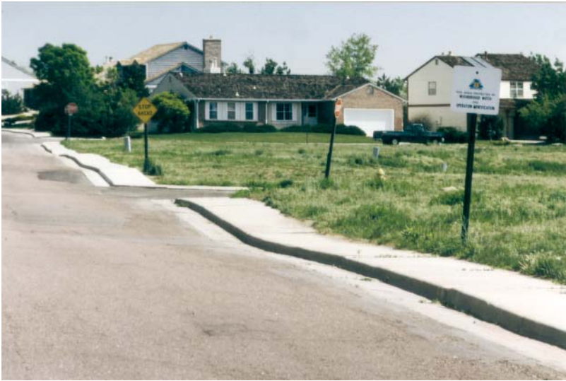
FIGURE 7.6. Linear heave ridges in a steeply dipping bedrock area near Denver, Colorado (Noe 2007).
