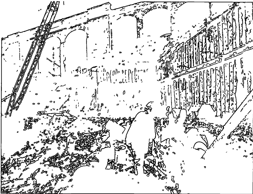
Figure 10.30 A contiguous bored pile retaining wall supported by ground anchors and reinforced cast-in-place walings
