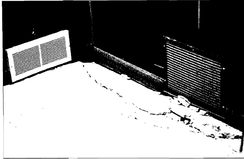
FIGURE 15.2 Typical cracking pattern around a basement slab that was meant to perform as a "floating slab"
