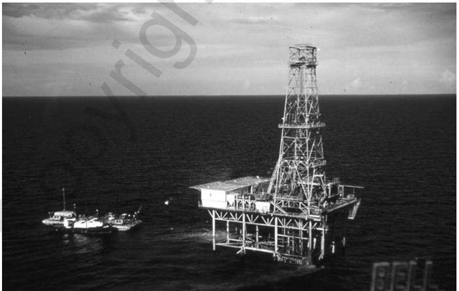
Figure 12.1 Helicopter view of an offshore drilling platform in the Gulf of Mexico.
