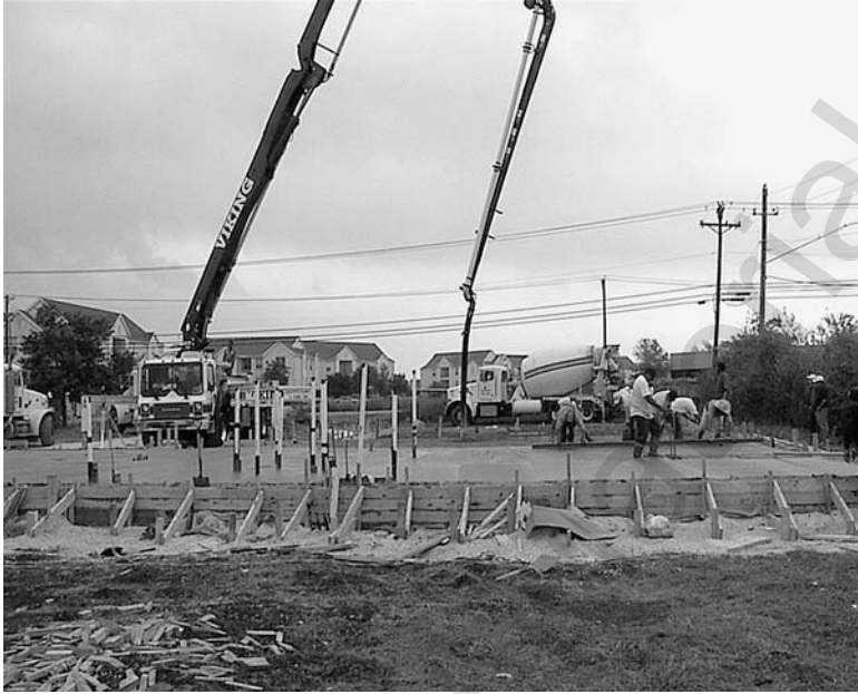
Figure 5.1 Construction of a shallow foundation in progress.
