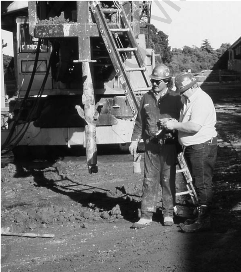
Figure 5.8 Drilling head used in construction of the GeoJet pile.
