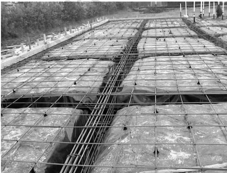
Figure 1.3 Shallow foundations under construction.
