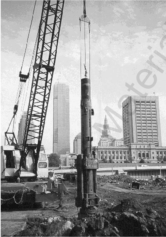
Figure 5.3 Impact hammer atop a driven pile.
