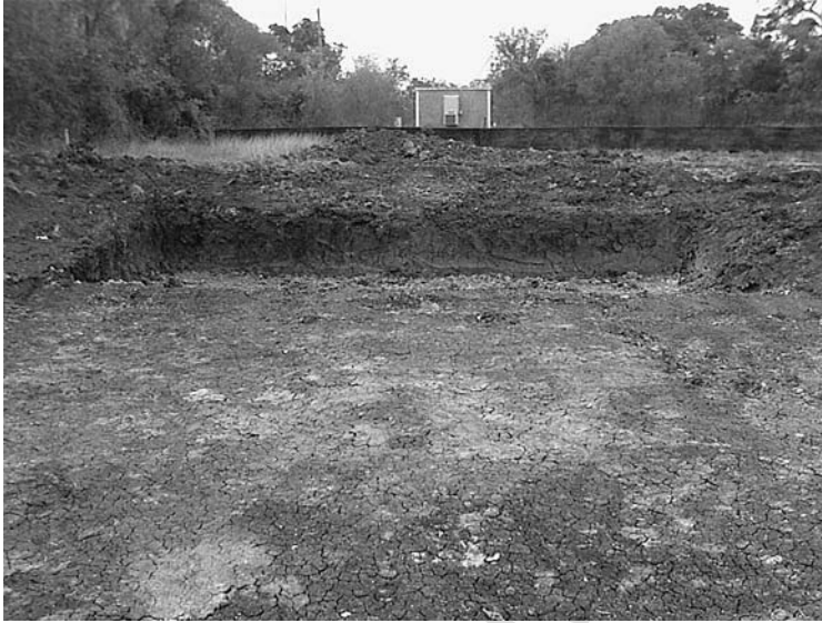
Figure 2.2 Desiccation cracking in expansive clay.
