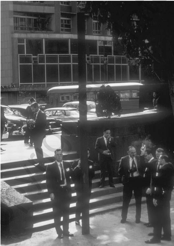
Figure 9.1 Photograph from Mexico City showing conference attendees standing next to a well casing showing subsidence over many years.
