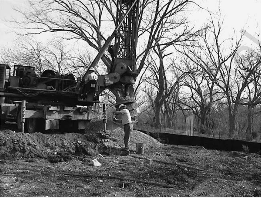
Figure 5.4 Construction of a drilled shaft with a truck-mounted unit.
