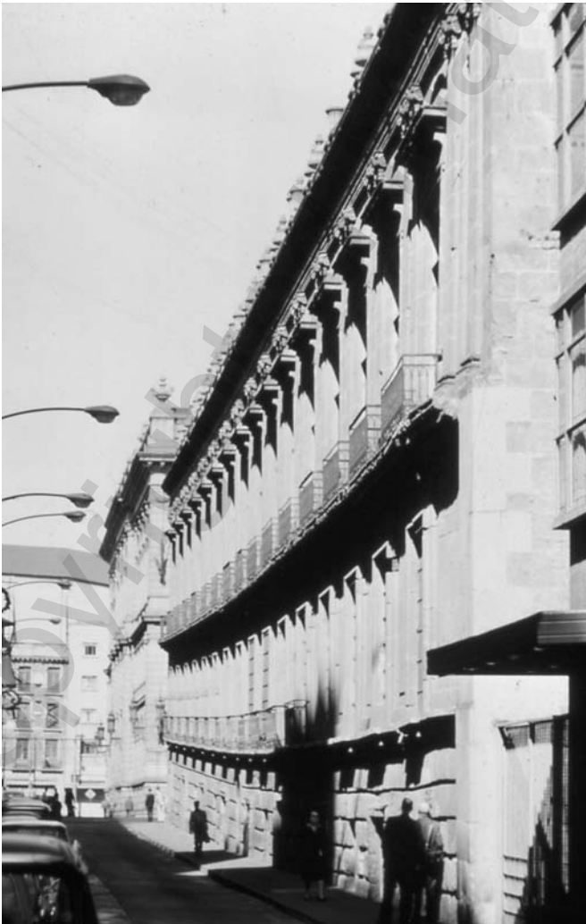
Figure 6.1 Photograph showing settlement of a government building in Mexico City.
