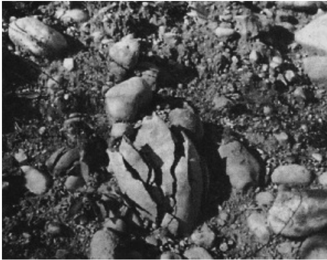
Fig. 5—Cobbles of argillaceous limestone disrupted by freezing-thawing in the deposit, near Charlesvoix, Michigan. Observation of natural disintegration forewarns of possible difficulty in service as concrete aggregate (courtesy of Michigan Department of Transportation).
