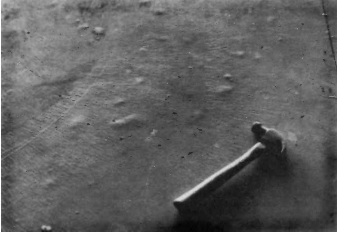
Fig. 22—Blisters (photo courtesy of the National Ready Mixed Concrete Association).
