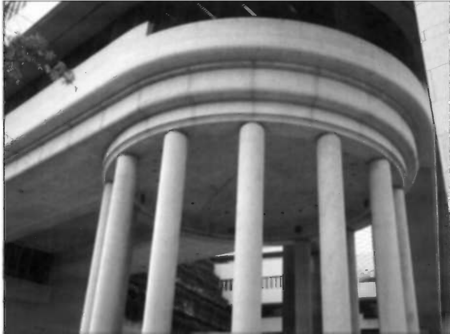
Fig. 17 —Canadian embassy in Washington, DC used slag cement in architectural concrete to achieve a very light color.
