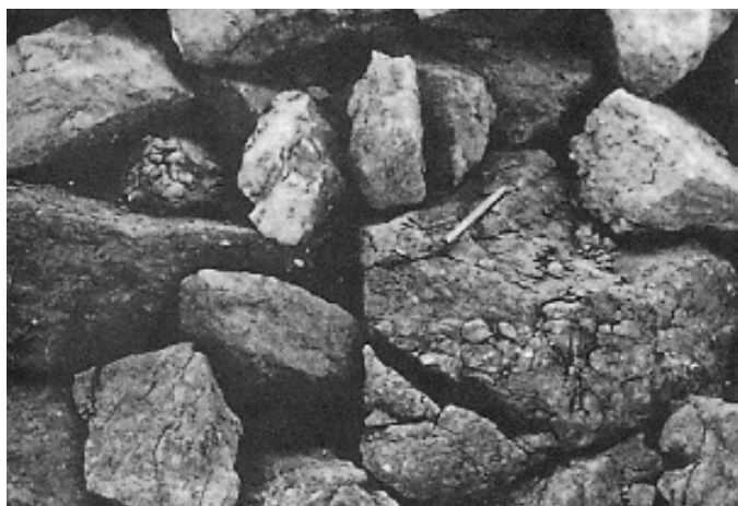
Fig. 8 —Disintegration of argillaceous facies of limestone used as riprap at Chickamauga Dam, Tennessee. Observation of such disintegration indicates unsoundness of stone in at least portions of a quarry (courtesy of the Bureau of Reclamation, U.S. Department of the Interior).
