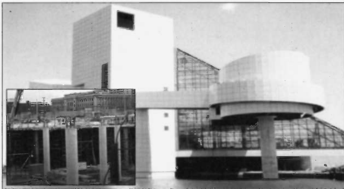
Fig. 18 —Rock ‘n Roll Hall of Fame in Cleveland used slag cement concrete in the exposed concrete pier foundation (inset) in lieu of white portland cement to closely match the white color of the tile exterior.
