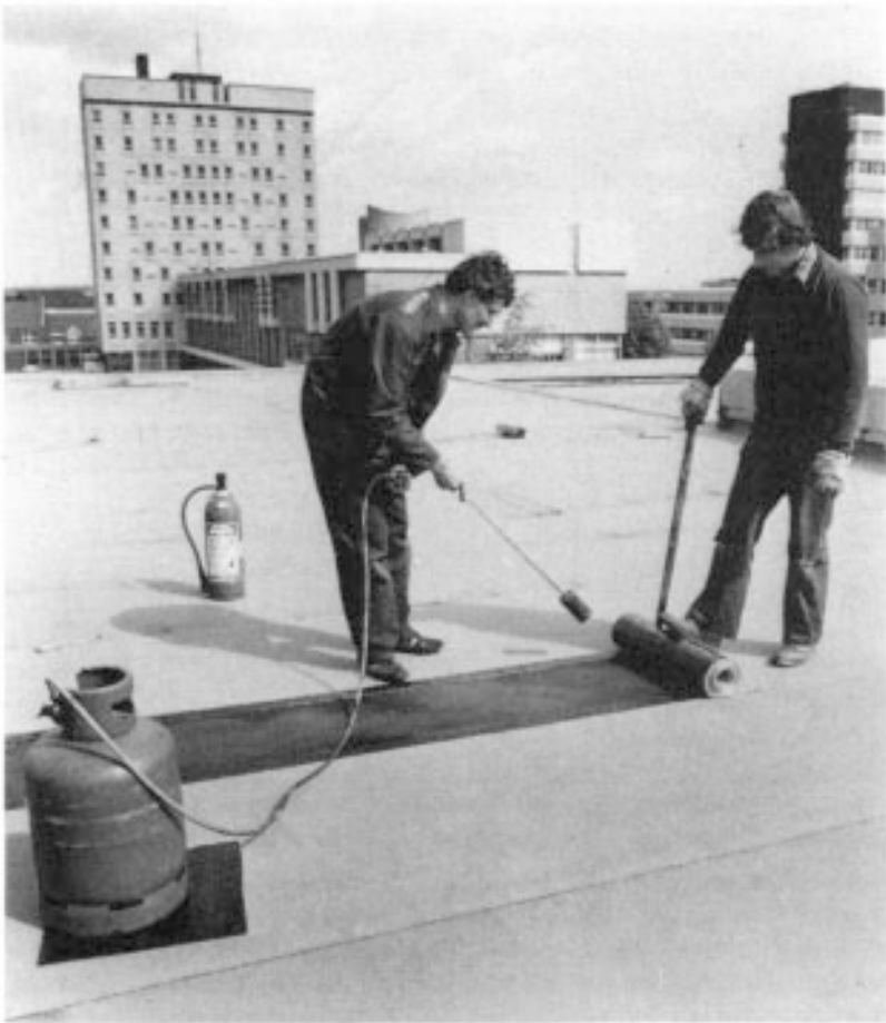
Figure 8.6 'Torch-on' roofing membrane. Courtesy, Ruberoid Ltd.
