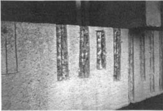
Figure 5.2 Preparation of concrete beam damaged by corrosion of stirrups.
