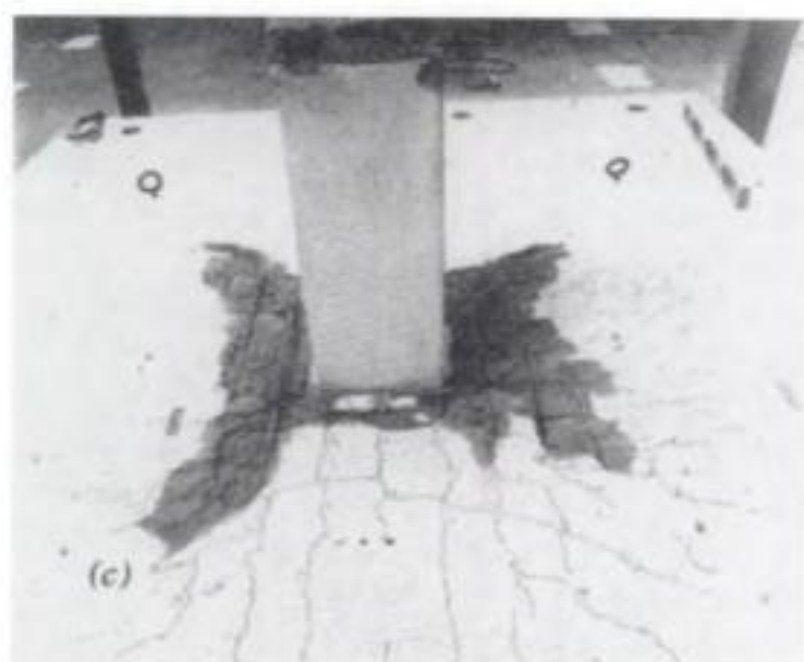
Figure 10.25 Reinforced concrete interior slab-column test specimen with closed stirrups as shear reinforcement 10,30 : (a) arrangement of reinforcement; (b) cracking in specimen after test; (c) broken concrete removed from specimen after test.
