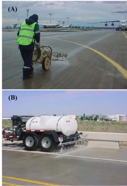
Figure 10.1 Application of the DCE solution by spraying onto cured concrete for an airport runway (A) and a pavement (B).
