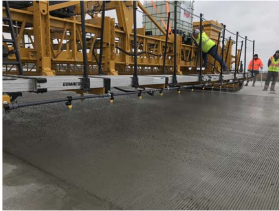
Figure 6.5 Application of waterproofing solution by spraying onto the surface of freshly poured concrete pavement.
