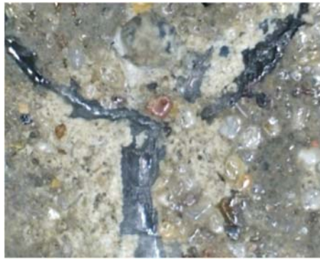
Figure 10.9 Large surface cracks ( > 1 mm) obtained in adverse curing conditions filled with the DCE crystals at 28 days (when the DCE solution is applied to fresh concrete) [30].
