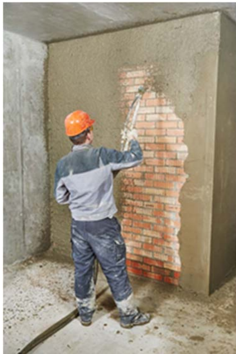
Figure 6.4 Application of cementitious coating by spraying.
