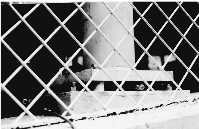
Figure 1.11 Flat jacks fitted under each new column.
