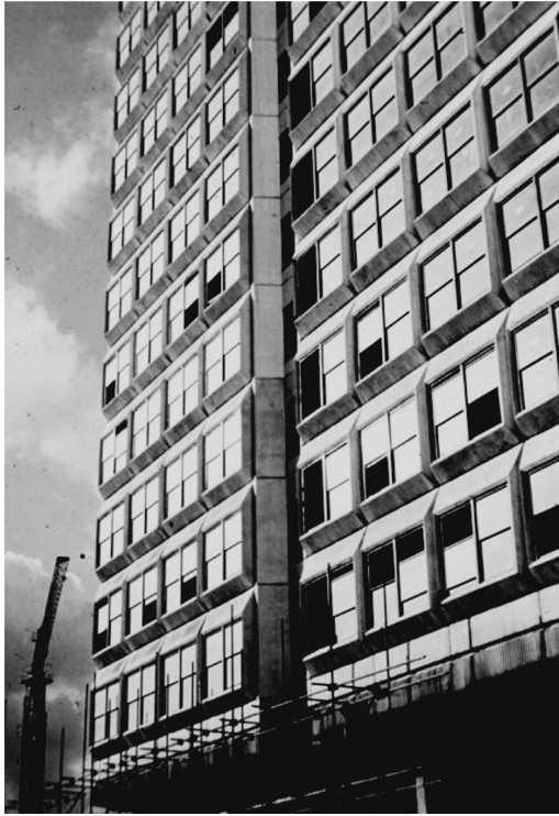
Figure 8.16 Office block with sculptured panel facades. (Courtesy of Poul Beckmann.)
