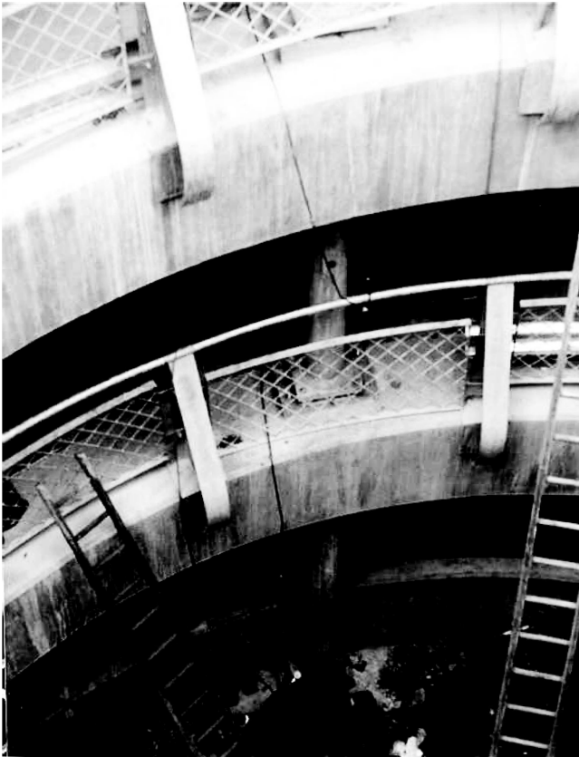
Figure 1.10 Additional steel columns.
