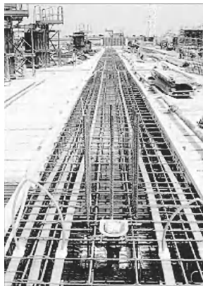
Figure 1.13 Typical beam under construction.
