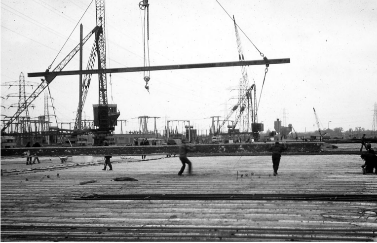
Figure 10.1 Pile casting yard.
