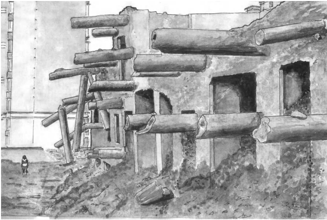
Figure 10.8 View of piles that failed in shear. (Courtesy of Gillian Whittle; redrawn from Reuters, http://www.telegraph.co.uk/news/worldnews/asia/china/5685963/Nine-held-over-Shanghai-building-collapse.html .)
