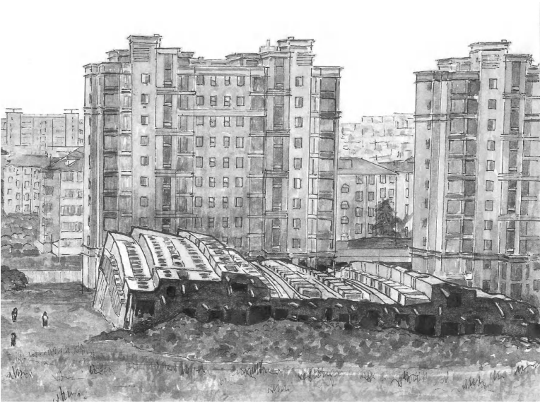
Figure 10.7 View of underside of collapsed building. (Courtesy of Gillian Whittle; redrawn from Reuters, http://www.telegraph.co.uk/news/worldnews/asia/china/5685963/Nine-held-over-Shanghai-building-collapse.html .)
