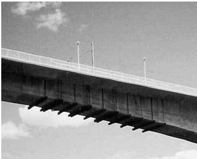
Figure 3.5 Temporary repair work on bridge.
