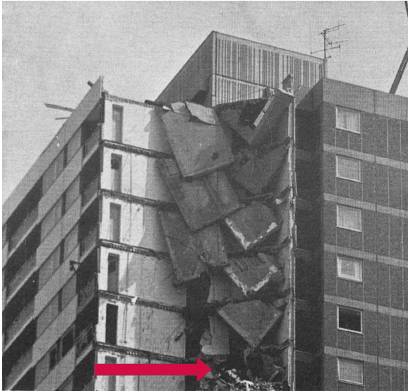
Figure 6.11 Closer view of upper floors showing point of explosion. (Ronan Point building collapse, May 16, 1968, London. Courtesy of Building Research Establishment.)
