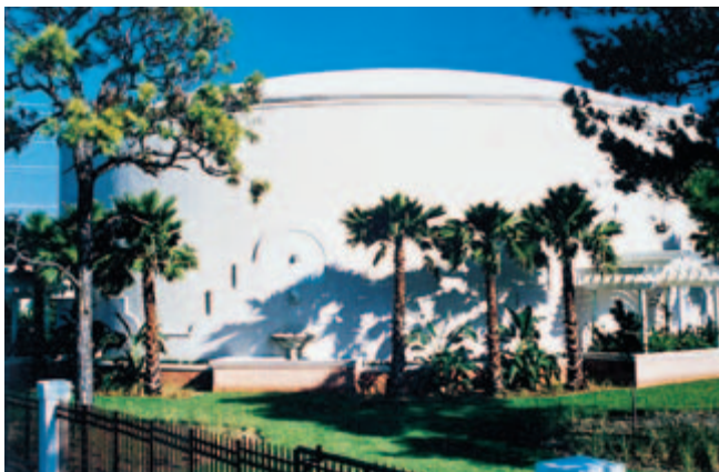
Fig. 2-24. Concrete has demonstrated decades of safe use in drinking water applications such as concrete tanks. (IMG12467)
