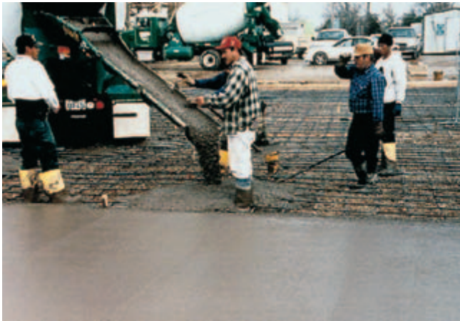
Fig. 6-10. Plasticized, flowing concrete is easily placed in thin sections such as this bonded overlay that is not much thicker than 1½ diameters of a quarter. (IMG12207)
