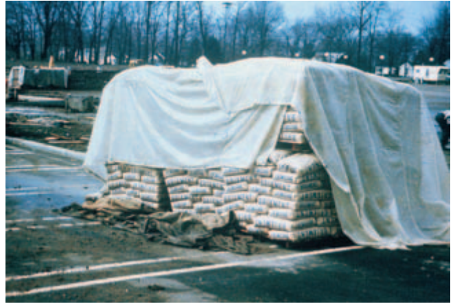
Fig. 2-54. When stored on the job, cement should be protected from moisture. (IMG12438)
