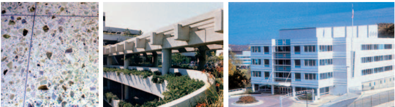
Fig. 2-18. White portland cement is used in white or light-colored architectural concrete, ranging from (left to right) terrazzo for floors shown here with white cement and green granite aggregate (IMG12475), to decorative and structural precast and cast-in-place elements (68981), to building exteriors. The far right photograph shows a white precast concrete building housing the ASTM Headquarters in West Conshohocken, Pennsylvania. Photo courtesy of ASTM.
