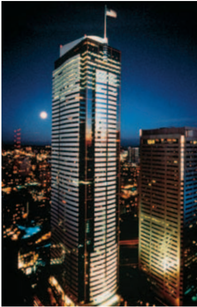
Fig. 17-5. The Two Union Square building in Seattle used concrete with a designed compressive strength of 131 MPa (19,000 psi) in its steel tube and concrete composite columns. High-strength concrete was used to meet a design criteria of 41 GPa (6 million psi) modulus of elasticity. (IMG12343)
