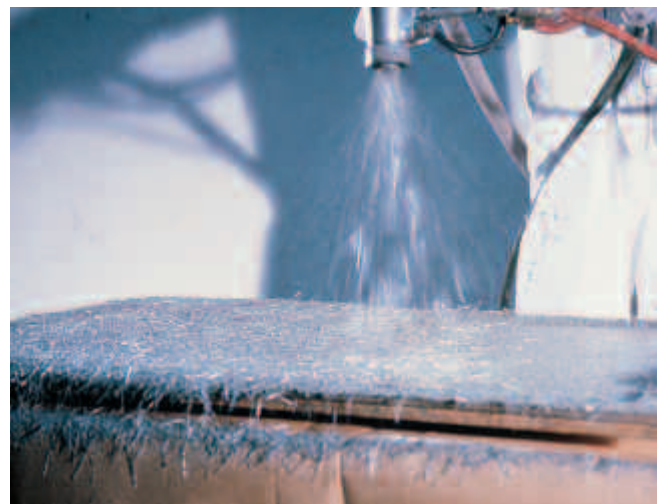
Fig. 7-5. (top) Glass-fiber-reinforced concrete panels are light and strong enough to reduce this building's structural requirements. (bottom) Spray-up fabrication made it easy to create their contoured profiles. (IMG12404, IMG12327)
