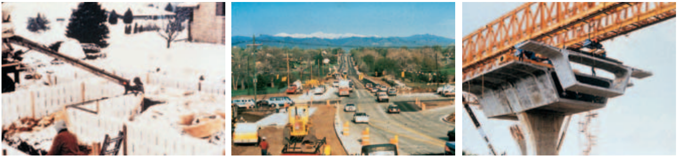
Fig. 2-17. High early strength cements are used where early concrete strength is needed, such as in (left to right) cold weather concreting, fast track paving to minimize traffic congestion, and rapid form removal for precast concrete. (IMG12350, IMG12477, IMG12476)
