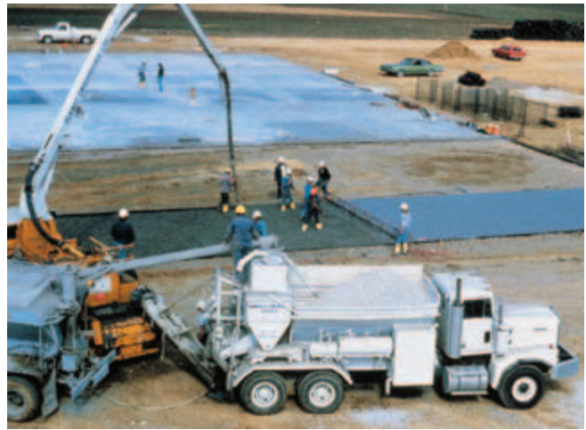
Fig. 10-7. Mobile batcher measures materials by volume and continuously mixes concrete as the dry ingredients, water, and admixtures are fed into a mixing trough at the rear of the vehicle. (IMG12248)
