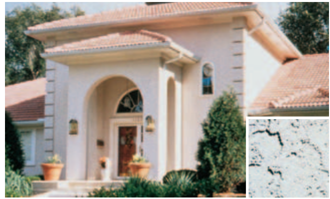
Fig. 2-21. Masonry cement and plastic cement are used to make plaster or stucco for commercial, institutional, and residential buildings. Shown are a church and home with stucco exteriors. Inset shows a typical stucco texture. (IMG12470, IMG12469, 68805)
