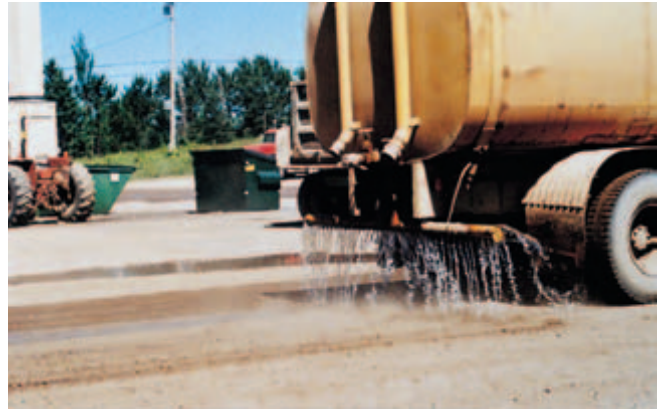
Fig. 11-2. Water trucks with spray-bars are used to moisten subgrades and base course layers to achieve adequate compaction and to reduce the amount of water drawn out of concrete as it's placed. (IMG12371)
