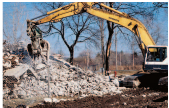
Fig. 5-25. Heavily reinforced concrete is crushed with a beam crusher. (IMG12419)
