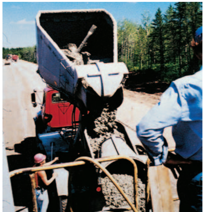
Fig 10-4. (top) Nonagitating trucks are used with central-mix batch plants where short hauls and quick concrete discharge allows the rapid placement of large volumes of concrete. (bottom) Truck agitators are also used with central-mix batch plants. Agitation mixing capabilities allow truck agitators to supply concrete to projects with slow rates of concrete placement and at distances greater than nonagitating trucks. (IMG12390, IMG12389)
