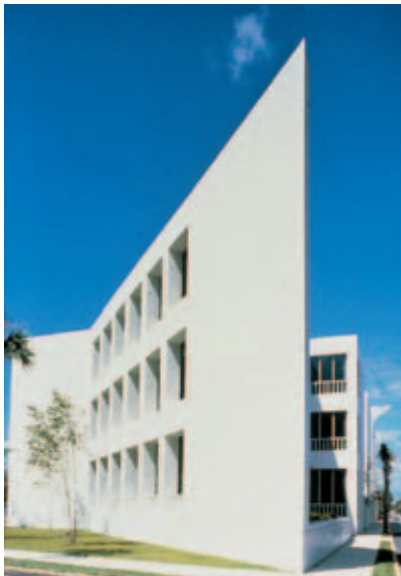
Fig. 18-15. Office building constructed with white cement concrete. (IMG12287)
