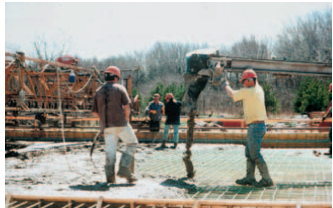
Fig. 11-5. The swing arm on a conveyor belt allows fresh concrete to be placed fairly evenly across a deck. (IMG12367)
