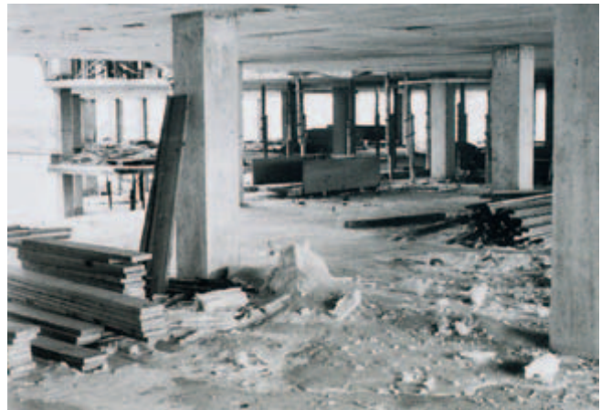
Fig. 14-11. Example of a concrete floor that was saturated with rain, snow, or water and then frozen, showing the need for air entrainment. (IMG12353)
