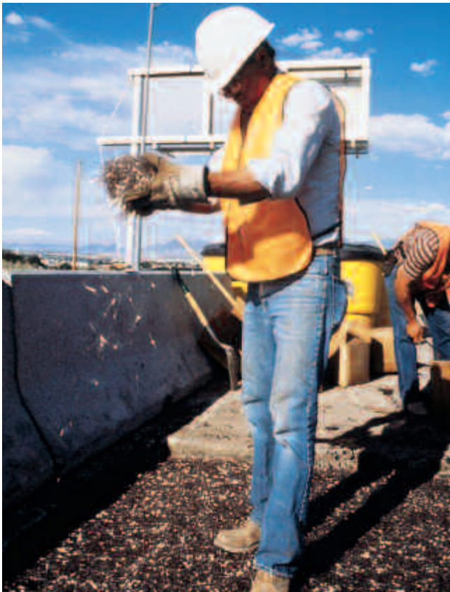
Fig. 7-4. Tightly bunched steel fibers are placed in a form, before cement slurry is poured into this application of slurry-infiltrated steel-fiber concrete (SIFCON). (IMG12409)
