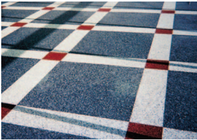
Fig. 6-19. Red and blue pigments were used to color this terrazzo floor. (IMG12208)
