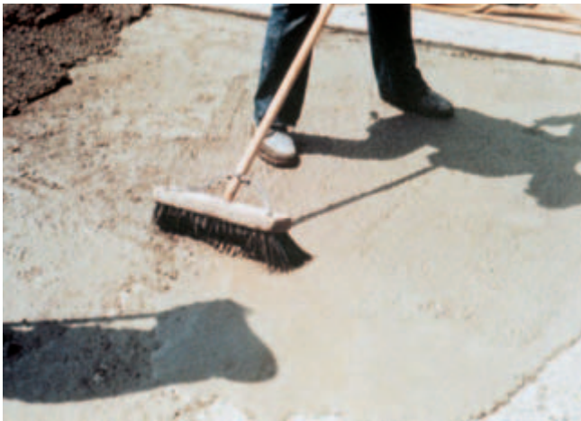
Fig. 11-25. Application of a bonding grout just ahead of the overlay concrete. The grout must not dry out before the concrete is placed. (IMG12254)
