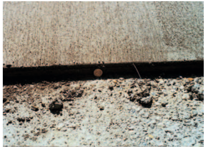
Fig. 6-10. Plasticized, flowing concrete is easily placed in thin sections such as this bonded overlay that is not much thicker than 1½ diameters of a quarter. (IMG12207)
