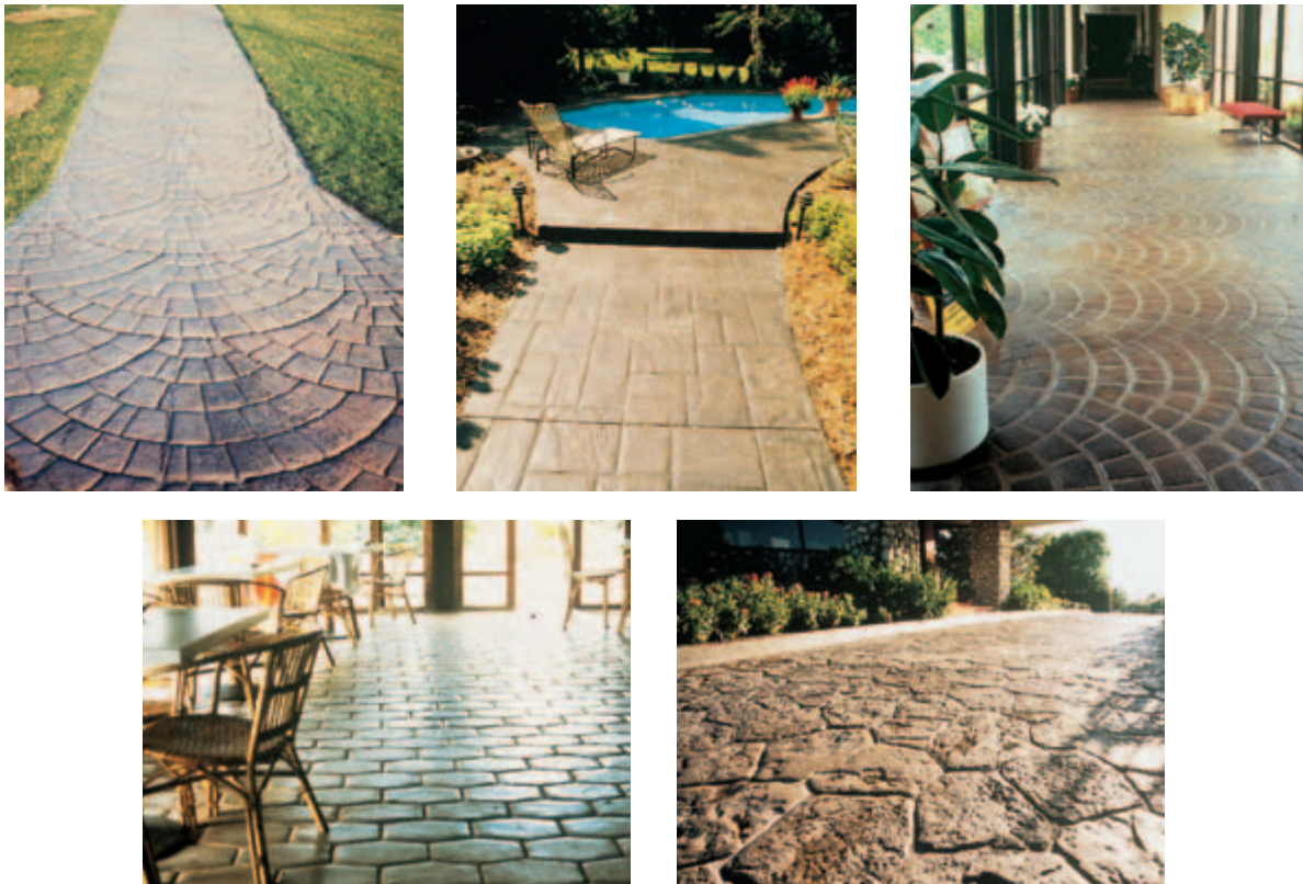
Fig. 11-35. Patterned, textured, and colored concretes are very attractive. (IMG9012, IMG7085, IMG12259, IMG12260, IMG12258)
