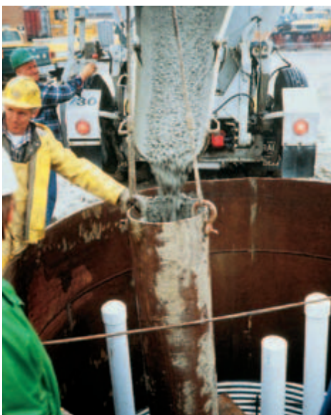
Fig. 18-8. (left) A drilled shaft (caisson), 3 m (10 ft) in diameter and 12.2 m (40 ft) in depth in which “low-heat” high-strength concrete is placed and (right) temperatures of this concrete measured at the center and edge and at three different levels in the caisson (Burg and Fiorato 1999). (IMG12290)
