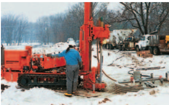
Fig. 2-22. (left) A slurry of finely ground cement and water can be injected into the ground, as shown here, to stabilize in-place materials, to provide strength for foundations, or to chemically retain contaminants in soil. (IMG12468) Illustration (right) of grout penetration in soil.
