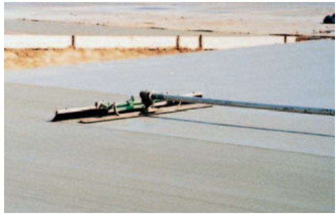
Fig. 11-20. Brooming provides a slip-resistant surface mainly used on exterior concrete. (IMG12377)
