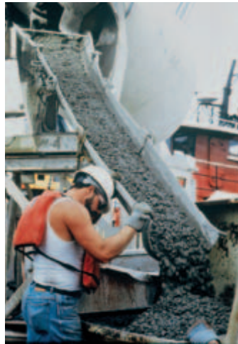
Fig. 1-5. Workable concrete should flow sluggishly into place without segregation. (IMG12299)
