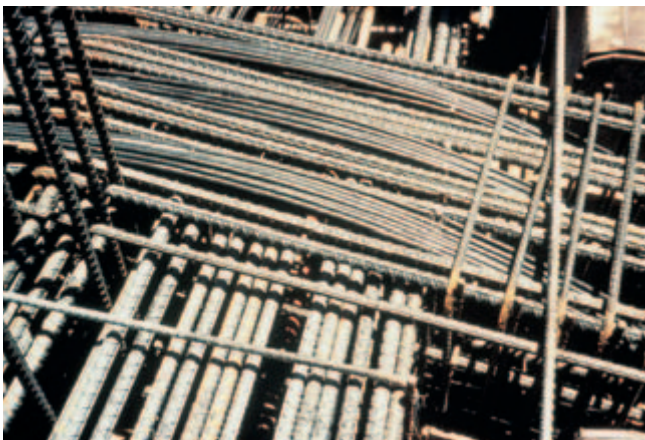
Fig. 6-9. Flowable concrete with a high slump (top) is easily placed (middle), even in areas of heavy reinforcing steel congestion (bottom). (IMG12324, IMG12325, IMG12326)
