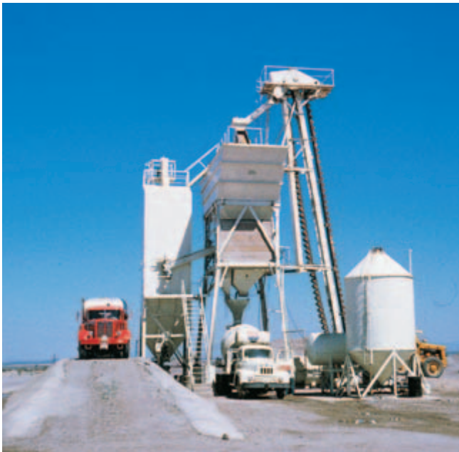
Fig. 10-6. Truck-mixed concrete is mixed completely in a truck mixer. (IMG12247)
