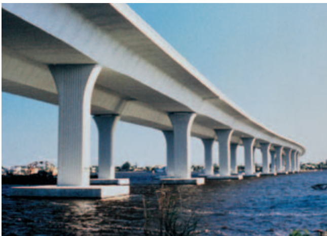
Fig. 1-34. Concrete bridges in seawater exposure must be specially designed for durability. (IMG12495)
