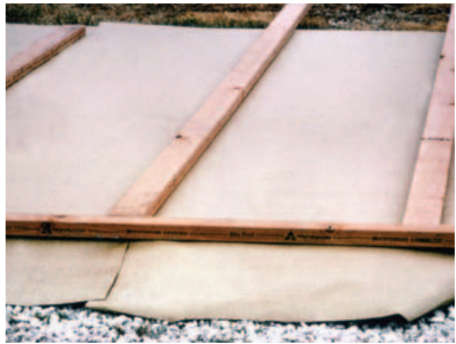
Fig.12-6. Impervious curing paper is an efficient means of curing horizontal surfaces. (IMG15128)
