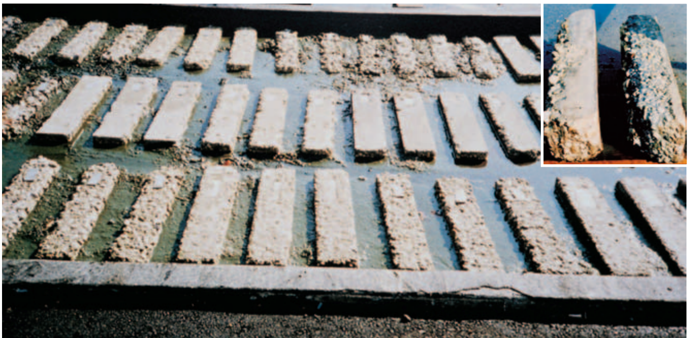
Fig. 1-32. Concrete beams after seven years of exposure to sulfate-rich wet soil in a Sacramento, California, test plot. The beams in better condition have low water-cementitious materials ratios, and most have sulfate resistant cement. The inset shows two of the beams tipped on their side to expose decreasing levels of deterioration with depth and moisture level. (IMG12296, IMG12496)
