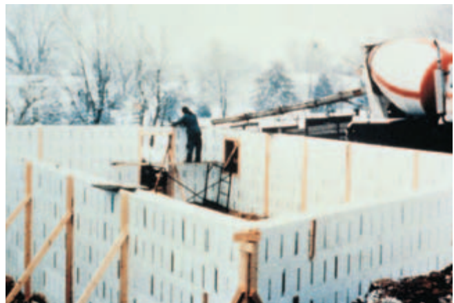
Fig. 14-20. Insulating concrete forms (ICF) permit concreting in cold weather. (IMG5003)
