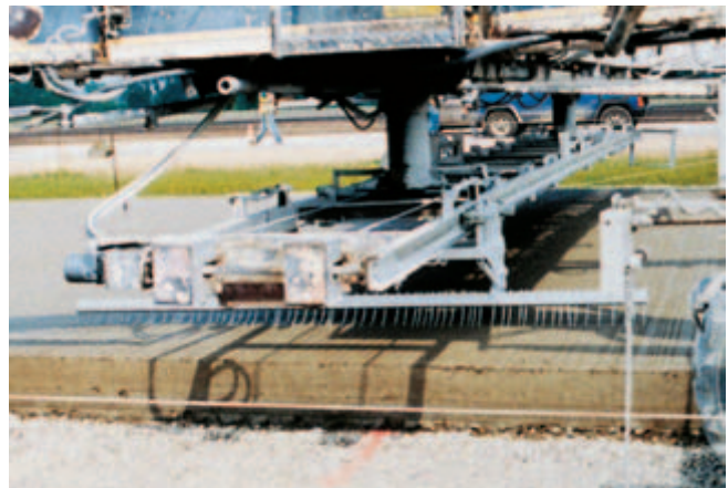
Fig. 11-20. Brooming provides a slip-resistant surface mainly used on exterior concrete. (IMG12377)
