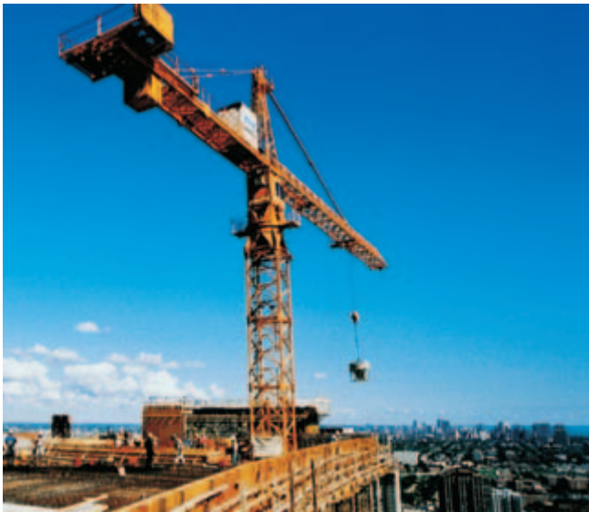
Fig. 10-12. The tower crane and bucket can easily handle concrete for tall-building construction. (IMG12396)
