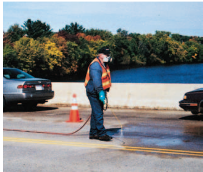
Fig 12-12. Penetrating sealers help protect reinforcing steel in bridge decks from corrosion due to chloride infiltration without reducing surface friction. (IMG12358)
