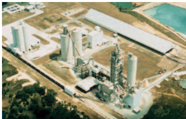
Fig. 2-5. Aerial view of a cement plant. (IMG12442)
