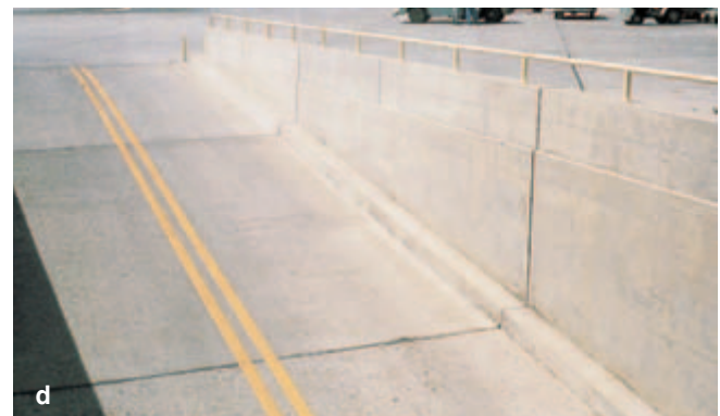
Fig. 15-10. (a) Illustration showing no crack development in concrete that is free to shrink (slab on rollers); however, in reality a slab on ground is restrained by the subbase (or other elements) creating tensile stresses and cracks. (b) Typical shrinkage cracks in a slab on ground. (c) A properly functioning contraction joint controls the location of shrinkage cracking. (d) Contraction joints in the slabs and walls shown will minimize the formation of cracks. (IMG12279, IMG12281, IMG12282)
