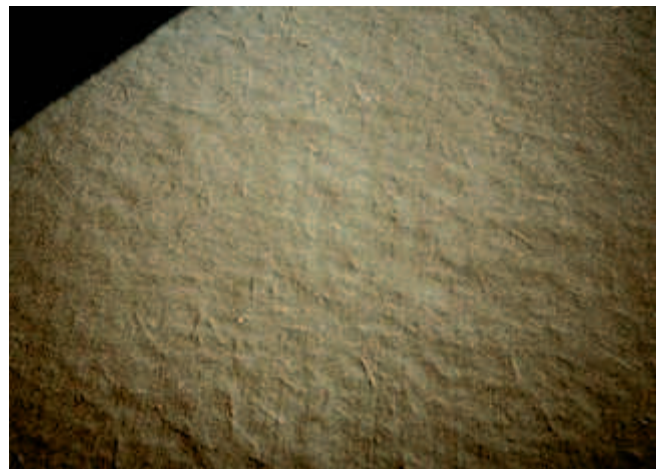
Fig. 7-3. Bridge deck with steel fibers. (IMG12410)
