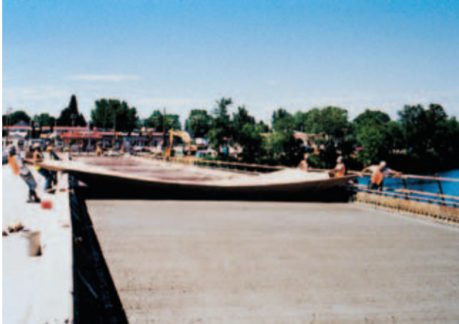
Fig. 11-22. An excellent method of wet curing is to completely cover the surface with wet burlap and keep it continuously wet during the curing period. (IMG12374)
