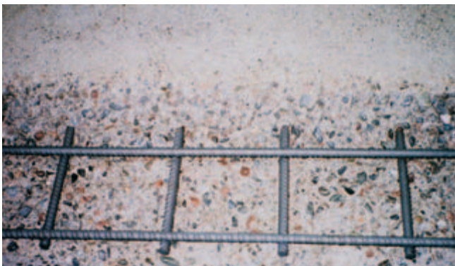
Fig. 11-32. Concrete prepared for patch installation. (IMG12372)
