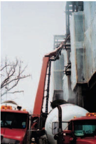
Fig. 14-1. When suitable preparations to build enclosures and insulate equipment have been made, cold weather is no obstacle to concrete construction. (IMG12272, IMG12271)
