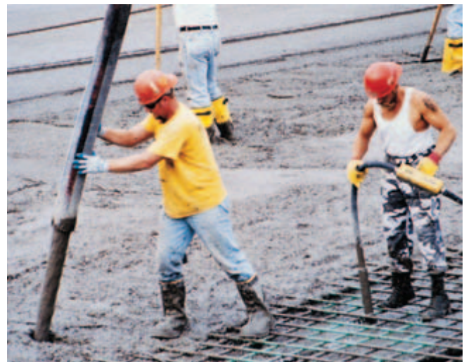
Fig. 10-15. (top) A truck-mounted pump and boom can conveniently move concrete vertically or horizontally to the desired location. (bottom) View of concrete discharging from flexible hose connected to rigid pipeline leading from the pump. Rigid pipe is used in pump booms and in pipelines to move concrete over relatively long distances. Up to 8 m (25 ft) of flexible hose may be attached to the end of a rigid line to increase placement mobility. (IMG12394, IMG12393)
