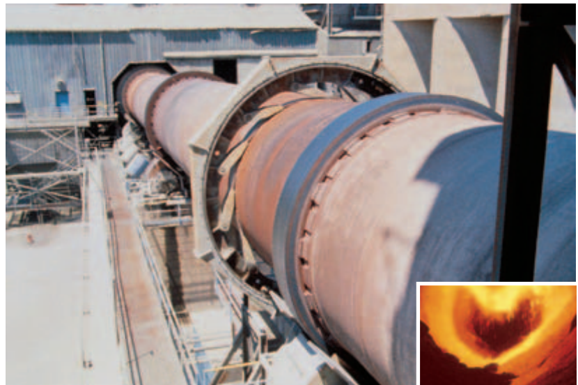
Fig. 2-8. Rotary kiln (furnace) for manufacturing portland cement clinker. Inset view inside the kiln. (IMG12307, IMG12435)
