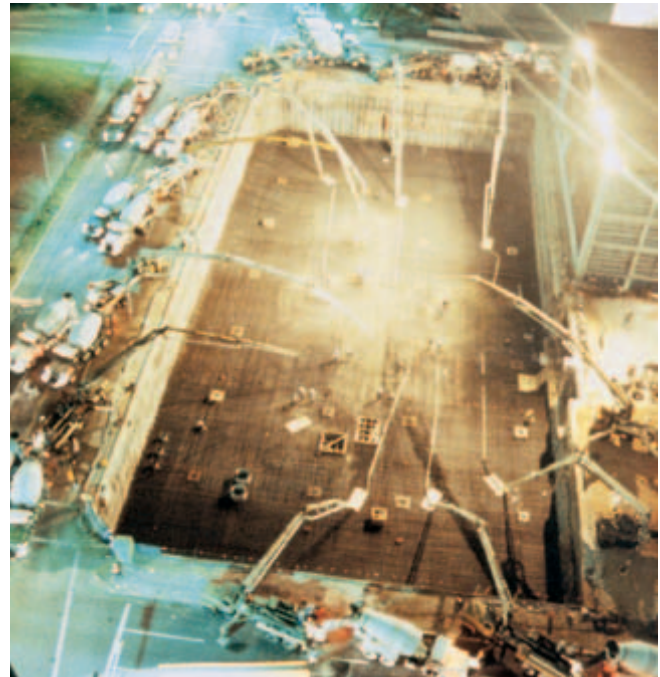
Fig.18-7. Large foundation placements as shown require mass-concrete precautions. (IMG12289)
