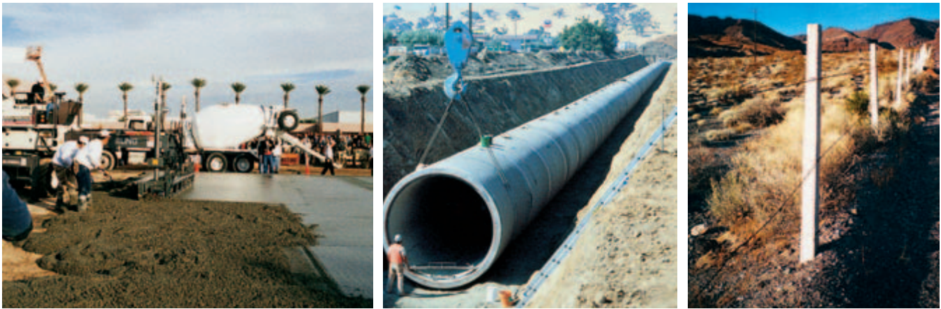
Fig. 2-14. Moderate sulfate resistant cements and high sulfate resistant cements improve the sulfate resistance of concrete elements, such as (left to right) slabs on ground, pipe, and concrete posts exposed to high-sulfate soils. (IMG12484, IMG12483, IMG12482)
