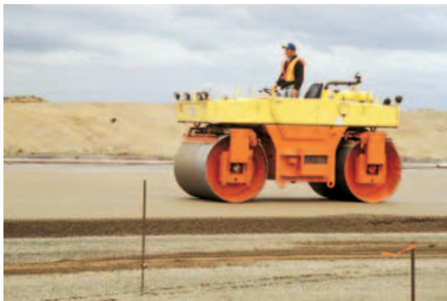
Fig. 18-11. Vibratory rollers are used to compact roller-compacted concrete. (IMG12338)
