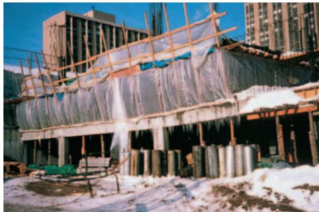
Fig. 14-1. When suitable preparations to build enclosures and insulate equipment have been made, cold weather is no obstacle to concrete construction. (IMG12272, IMG12271)
