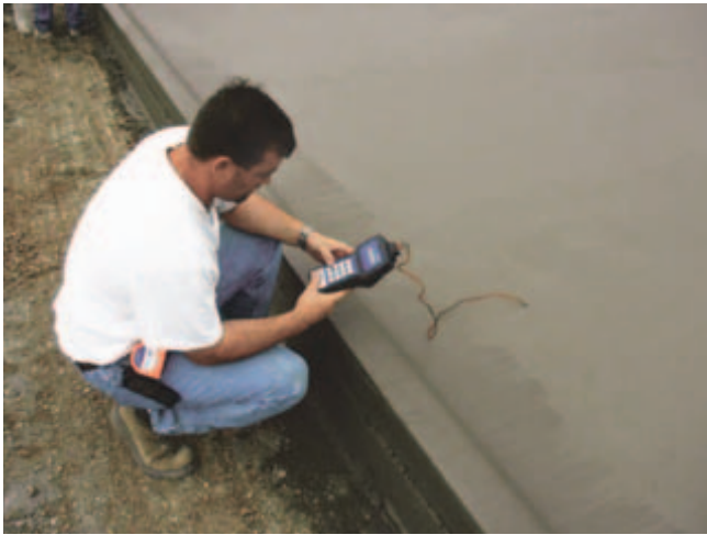
Fig. 14-26. Downloading data from a maturity sensor embedded in a pavement. (IMG19163)
