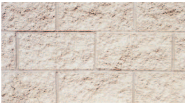
Fig. 2-20. Masonry cement and mortar cement are used to make mortar to bond masonry units together. (IMG12471)
