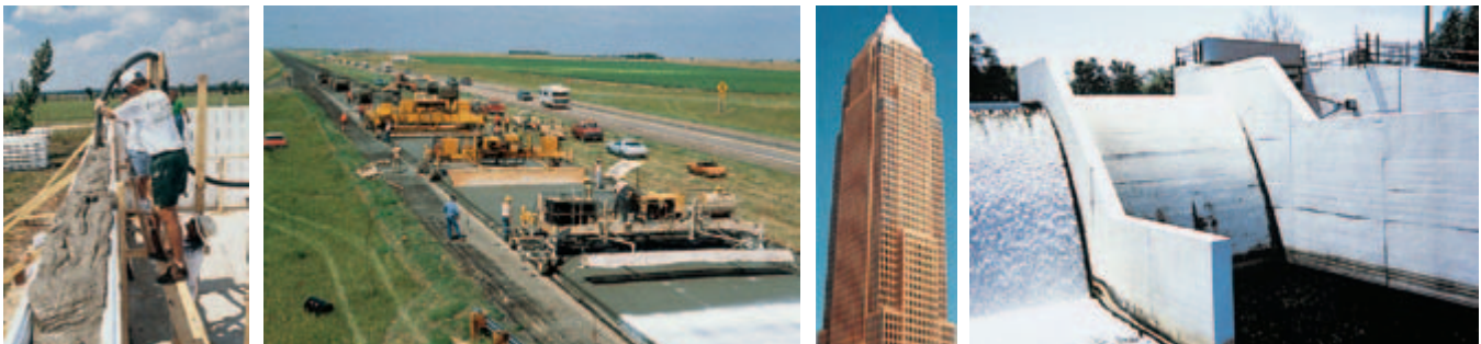
Fig. 3-4. Fly ash, slag, and calcined clay or calcined shale are used in general purpose construction, such as (left to right) walls for residential buildings, pavements, high-rise towers, and dams. (IMG12431, IMG12310, IMG12430, IMG12429)
