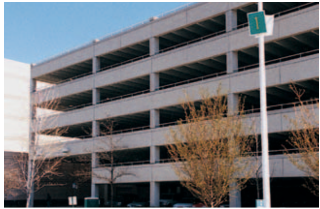
Fig. 3-9. Although they can be used in general construction, silica fume and metakaolin are often used in applications such as (left) bridges and (right) parking garages to minimize chloride penetration into concrete. (IMG12427, IMG12426)
