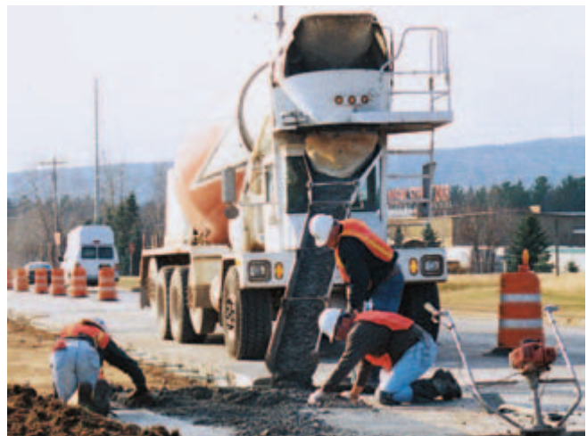
Fig. 10-11. In comparison to conventional rear-discharge trucks, front-discharge truck mixers provide the driver with more mobility and control for direct discharge into place. (IMG12397)
