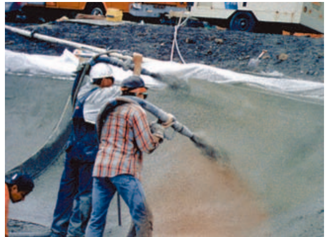
Fig. 18-13. Shotcrete. (IMG12341)
