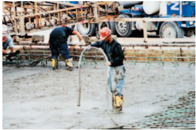
Fig. 11-11. Internal vibrators are commonly used to consolidate concrete in walls, columns, beams, and slabs. (IMG12387)
