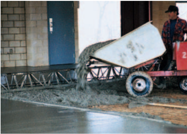
Fig. 11-8. Concrete should be placed as near as possible to its final position. (IMG12364)
