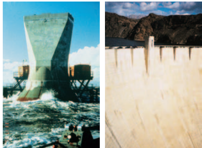
Fig. 2-16. Moderate heat and low heat cements minimize heat generation in massive elements or structures such as (left) very thick bridge supports, and (right) dams. Hoover dam, shown here, used a Type IV cement to control temperature rise. (IMG12479, IMG12478)
