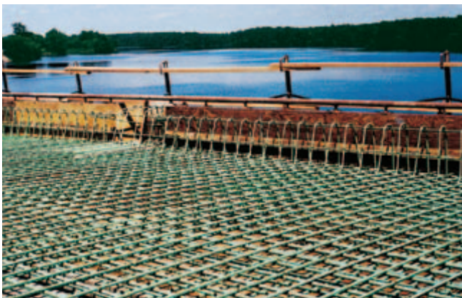
Fig. 1-30. Epoxy-coated reinforcing steel used in a bridge deck. (IMG12498)
