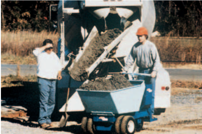
Fig. 10-8. Versatile power buggy can move all types of concrete over short distances. (IMG12249)
