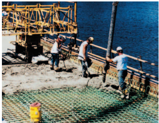
Fig. 6-6. Low water to cement ratio concrete with low chloride permeability—easily made with high-range water reducers—is ideal for bridge decks. (IMG12413)
