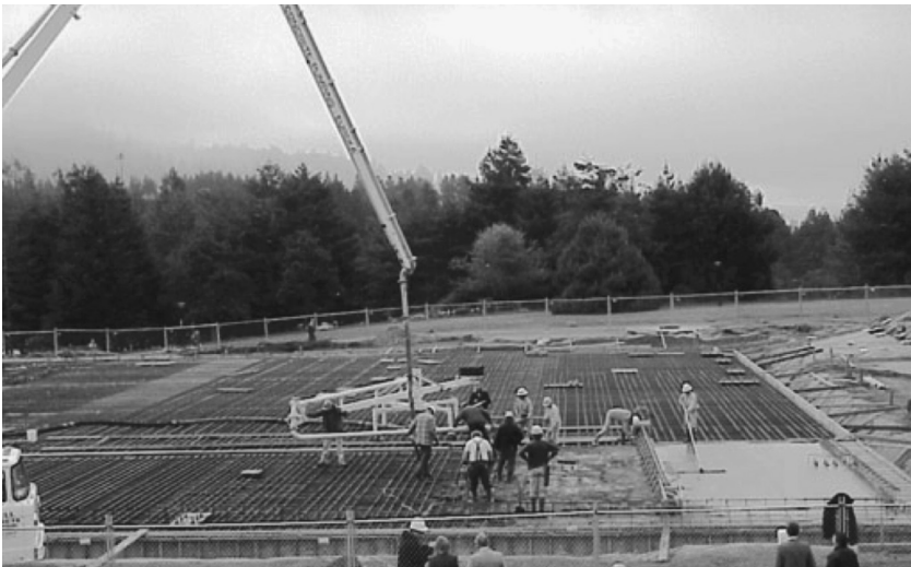
FIGURE 5.24 Pouring raft foundation by using pump.
