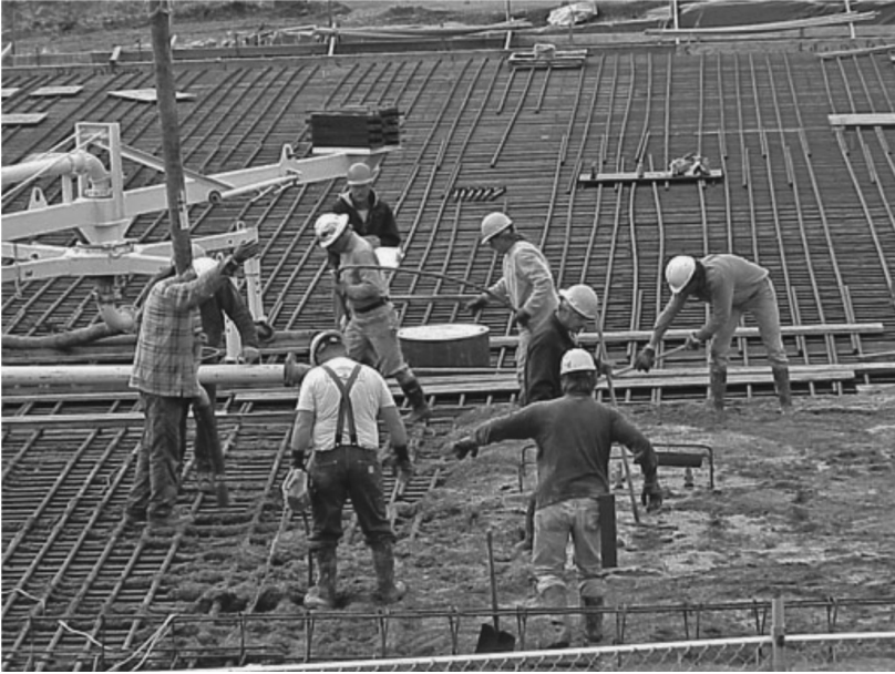
FIGURE 5.25 Pump concrete in pouring a slab.
