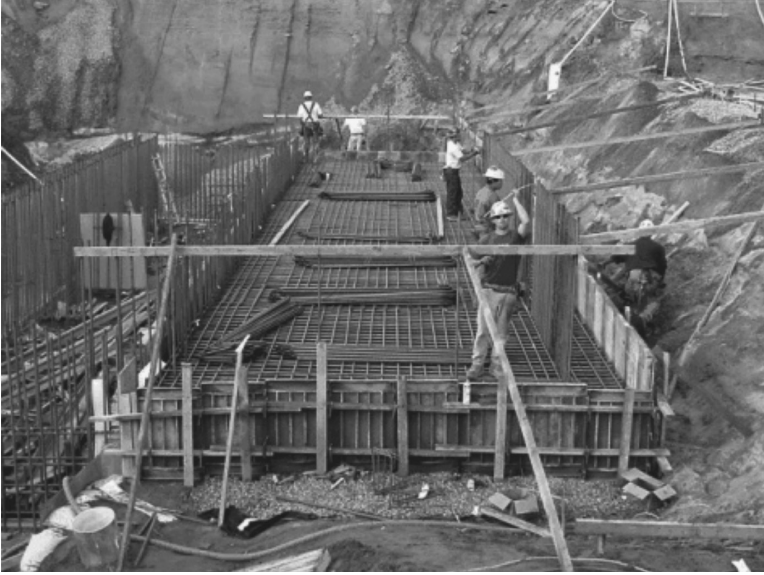
FIGURE 5.14 Steel bars between foundation and wall.
