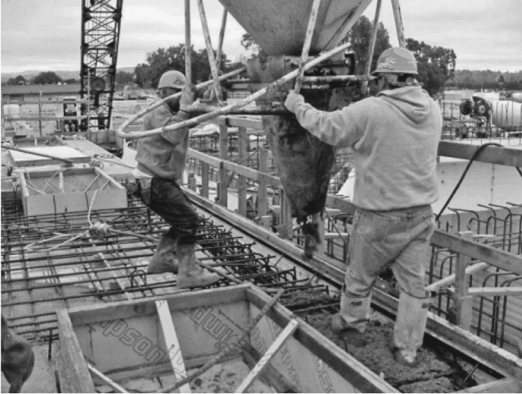
FIGURE 5.27 Pouring beam by using caisson.
