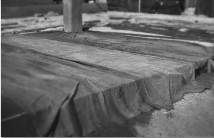
FIGURE 5.35 Curing by using textile.
