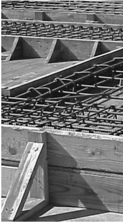
FIGURE 5.4 Strengthening wood form for ground slab.
