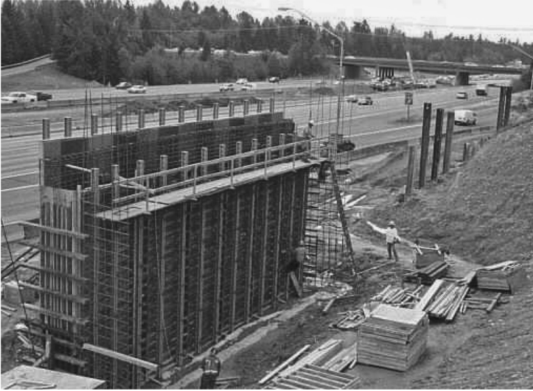
FIGURE 5.1 Formwork for reinforced concrete wall.
