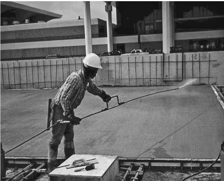
FIGURE 5.49 Spraying chemical compound on the surface.
