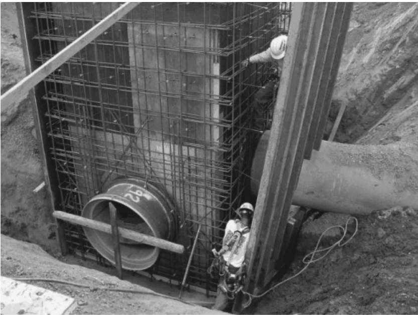
FIGURE 5.13 Wall steel bars with pipe sleeve.
