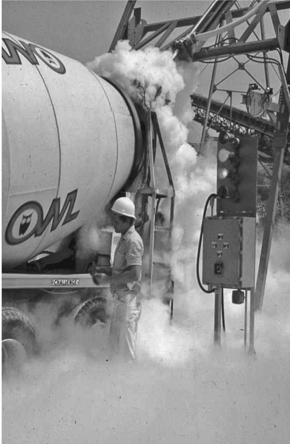
FIGURE 5.42 Using nitrogen for cooling.
