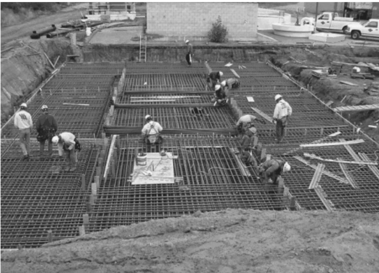
FIGURE 5.15 Distributing steel reinforcement in concrete raft.
