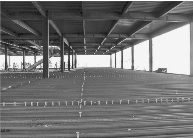
FIGURE 7.58 Stud bolts in roof slab.
