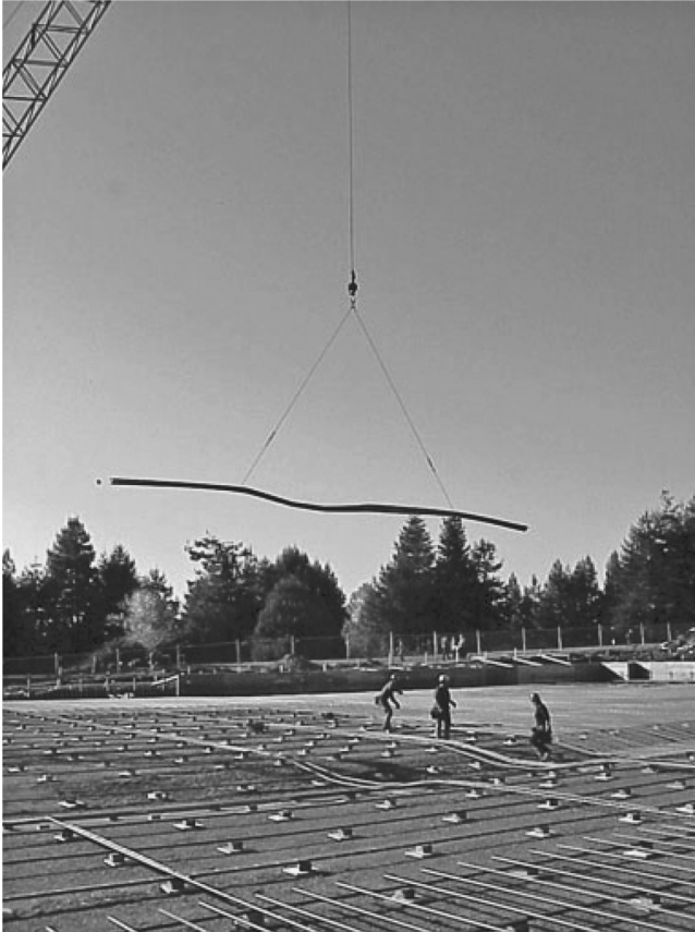
FIGURE 5.11 Distributing steel bars for ground slab.
