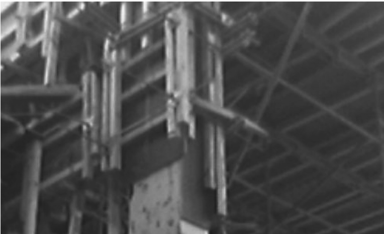
FIGURE 5.7 Steel supports with marine plywood.
