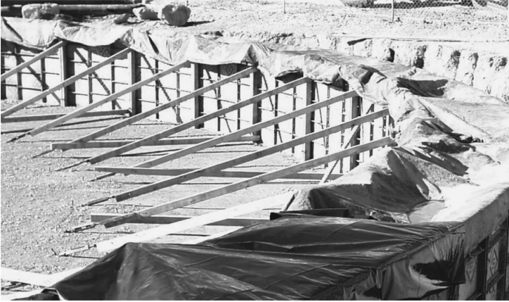
FIGURE 5.37 Plastic sheet to protect from evaporation.
