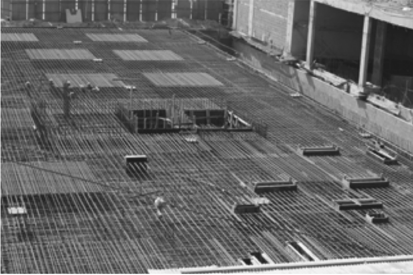
FIGURE 5.12 Steel bars for raft foundation.
