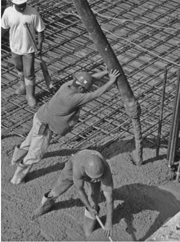
FIGURE 5.28 Preparing concrete surface.
