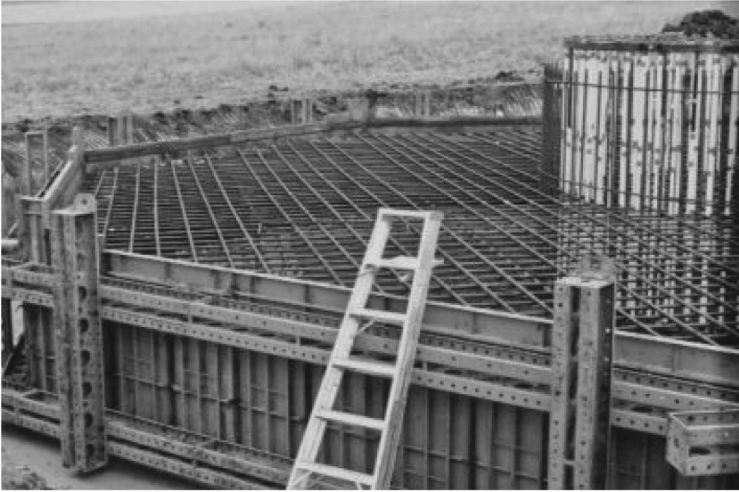
FIGURE 5.5 Steel form for raft foundation.
