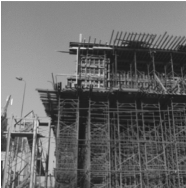
FIGURE 5.2 Bridges and slab form support.
