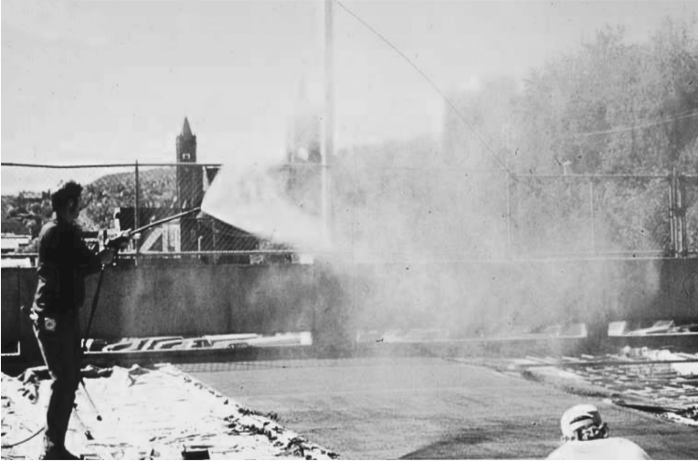
FIGURE 5.48 Curing concrete with silica fume.
