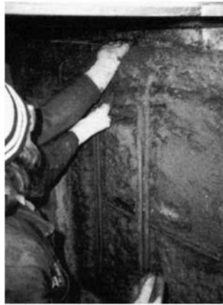
Fig. 8. Hand-applied repair being carried out without any form of shuttering
