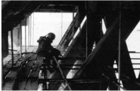
Fig. 3. The nozzleman spraying Gunite onto an inclined concrete element
