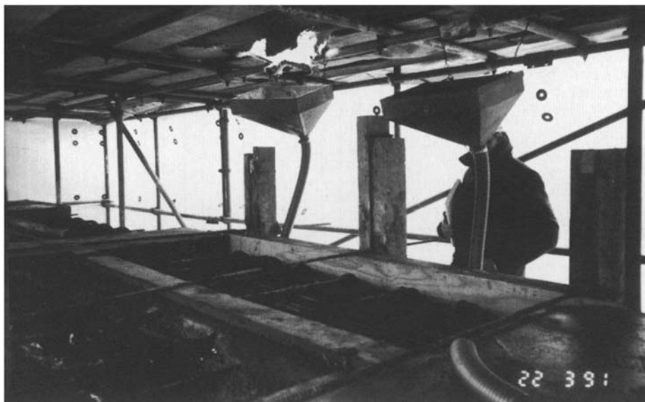
Figure 7—Placement by funnel and tube
