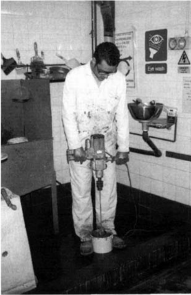
Fig. 5a. and 5b. Slow speed drill and paddle for mixing repair materials
