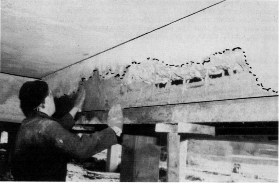
Fig. 7. Filling and compacting of a beam repair using the hand-packing technique
