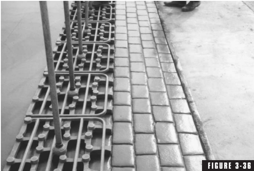
Pattern stamped concrete. (Photo courtesy PCA).
