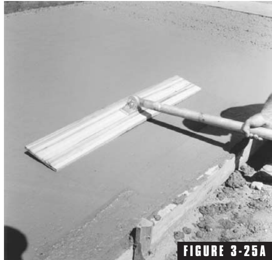
FIGURE 3-25A Bull float (Photo Courtesy PCA).
