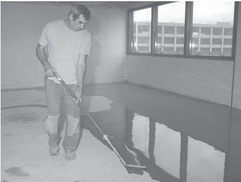
Figure 2.22 Application of floor-levelling compound.
