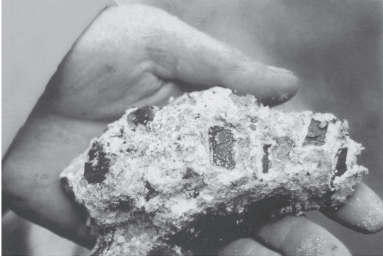
Figure 5.13 A severe example of the thaumasite type of sulphate attack in a hand specimen of concrete.
