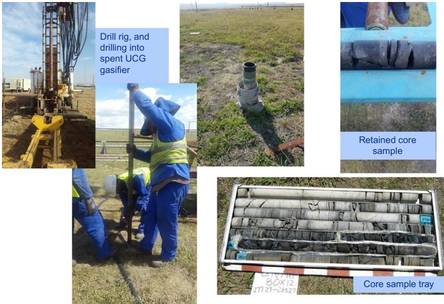
Fig. 14.23 Verification drilling and sampling.
