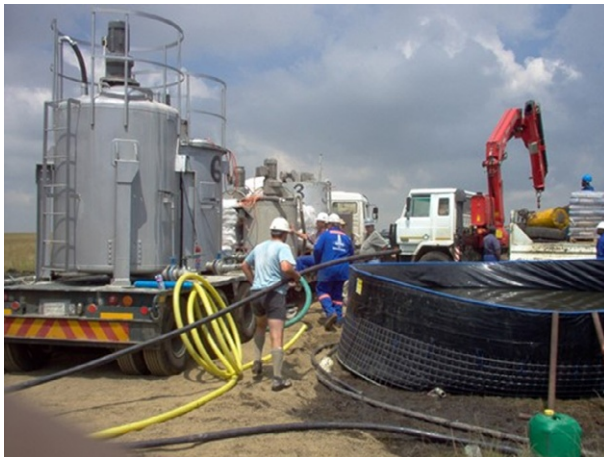
Fig. 14.12 Well casing cementation unit.
