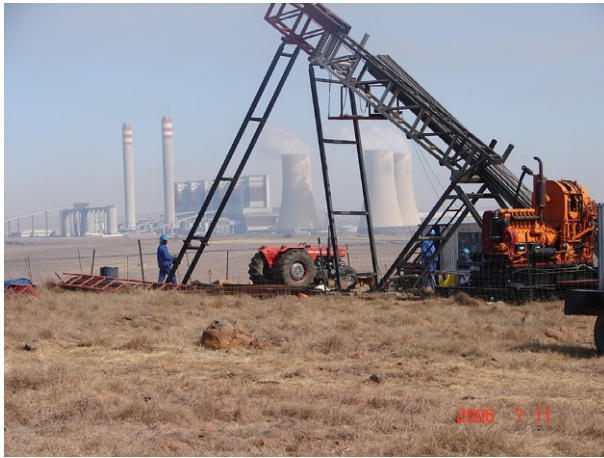
Fig. 14.11 Directional drilling rig with Majuba Power Station in the background.
