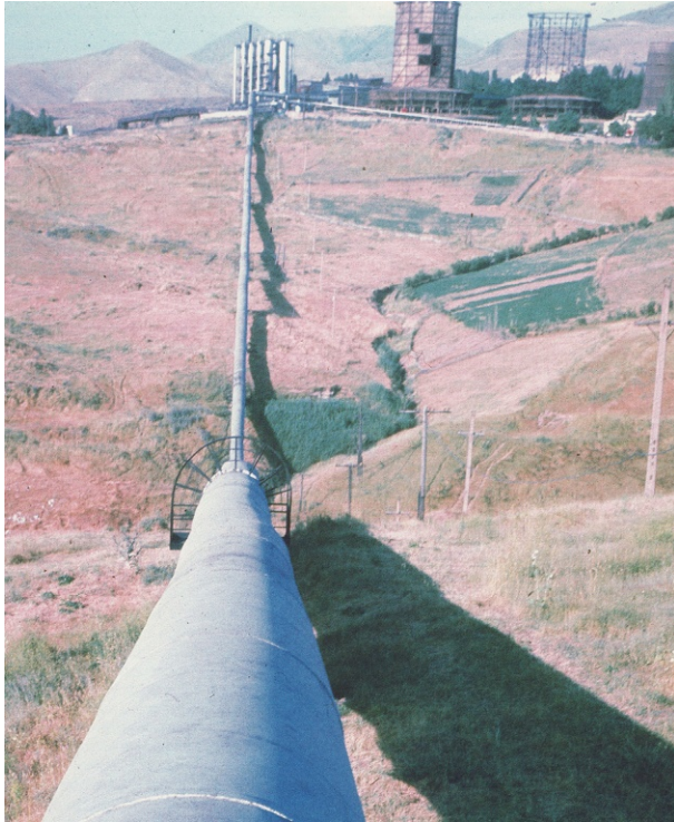
Picture 3.3 Main trunk gas pipeline to power station.
