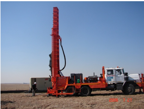
Fig. 14.10 Vertical drilling rig.
