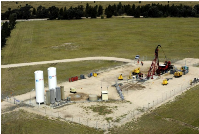
Fig. 6.8 Linc Energy gasifier 5 construction.
