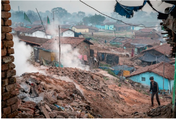
Fig. 17.3 In Jharia, several houses have collapsed due to the fires (Schiller, 2015) (photo, Johnny Haglund). Toxic gases adversely affect the health of local population.
