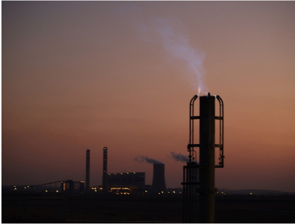
Fig. 14.20 15,000 Nm 3 /h gas flare stack with Majuba Power Station in background.
