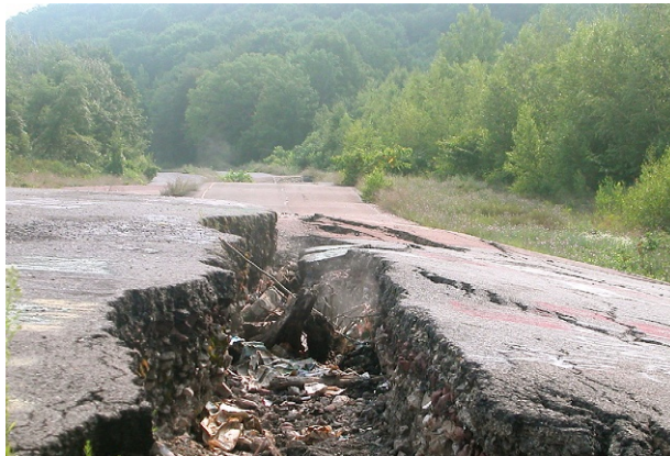
Fig. 17.4 Smoke emanating from a fissure in the road on the abandoned section of highway 61 near Centralia, PA. An underground mine fire has been burning there since 1962 (Matić, 2015). Taken from https://www.flickr.com/photos/citnaj/981132198 . Image under Creative Commons license.
