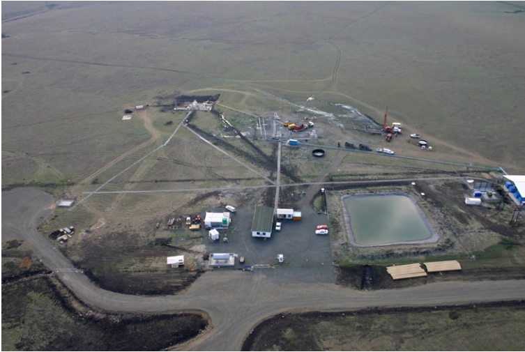
Fig. 14.9 Aerial view of Eskom Majuba UCG pilot site, October 2006.
