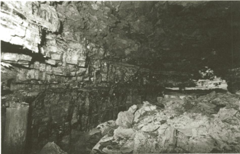
Fig. 7.4.3. Caved roof span without self-supporting abilities regardless on external support (timber).
