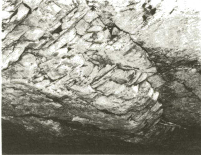
Fig. 7.4.8. Shear displacement and shear failure propagated upwards.
