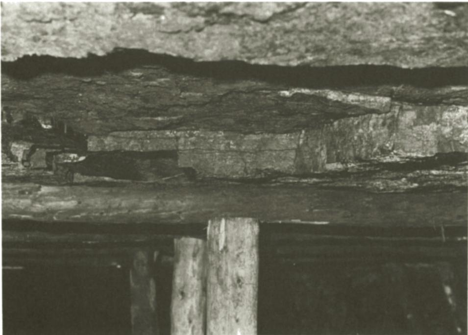
Fig. 4.1.8. Dilation (separation) and shearing of roof layers.
