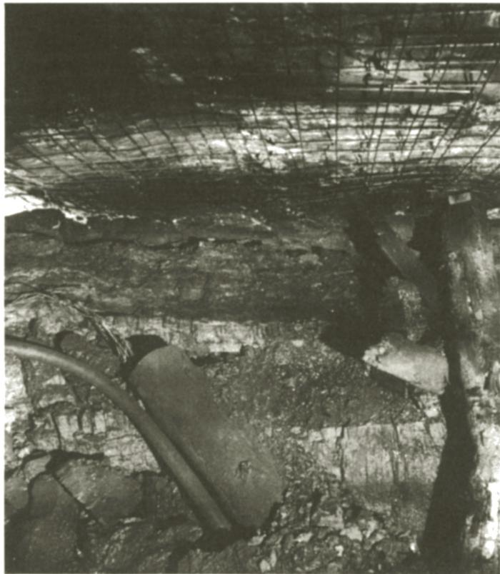
Fig. 5.2.8. Stable roof conditions after displacement and limited sagging.
