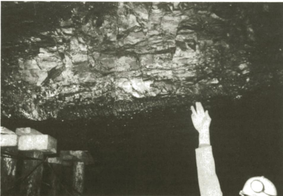
Fig. 4.1.10. Mine roof reinforcement by leaving coal layers (Western Collieries, Australia).
