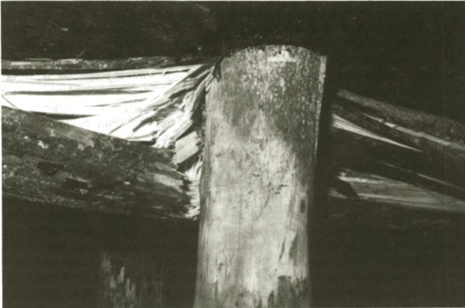
Fig. 4.2.1. The break of timber caps due to vertical displacement and horizontal slips of roof strata.
