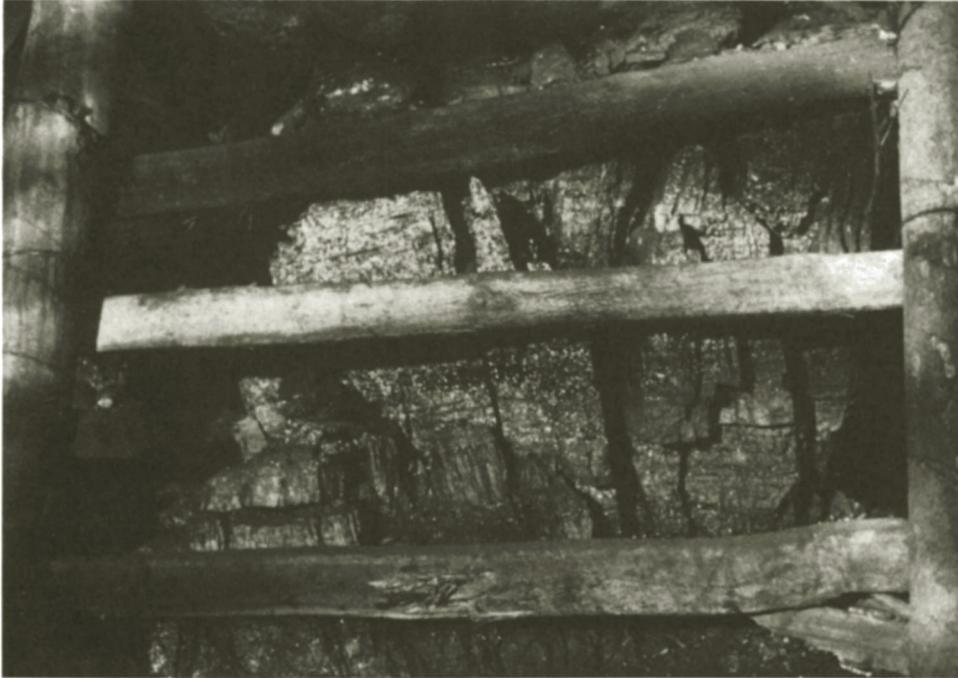
Fig. 6.2.8. Pillar within plastic state of deformations with fracture development (McIntyre Porcupine Mine, Canada).
