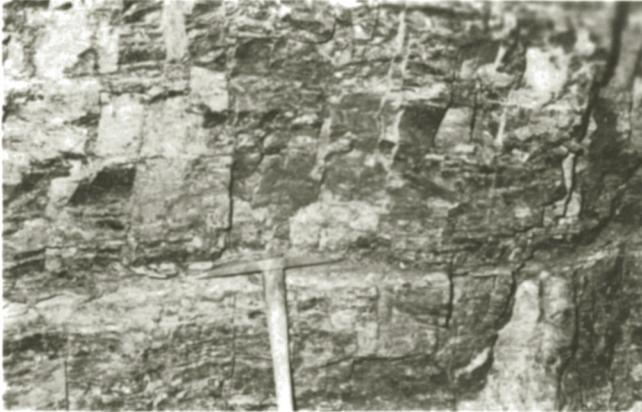
Fig. 6.2.4. Rib wall perpendicular to cleat in weathered coal.
