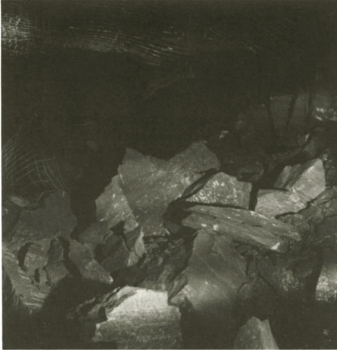
Fig. 4.2.8. Incomplete roof caving of the massive sandstone (fragmentation in large blocks).
