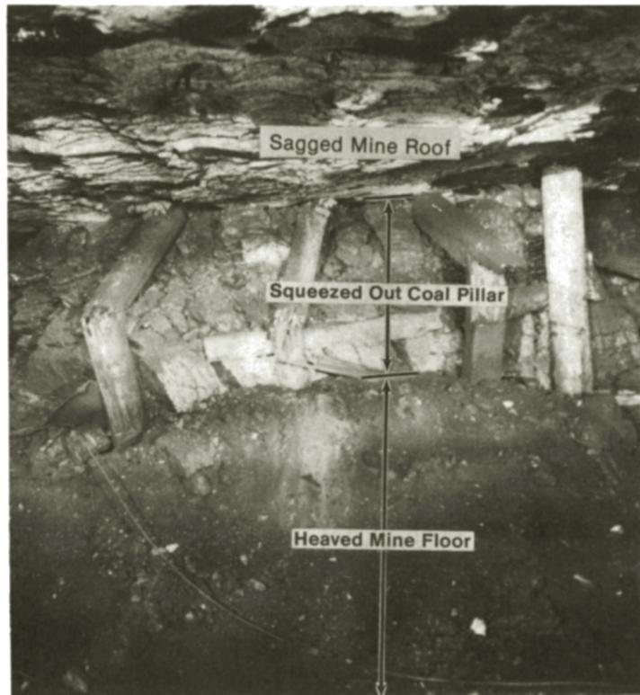
Fig. 6.4.1. Differential closure deformations due to existence of sandstone roof and coal-shale floor stratum.
