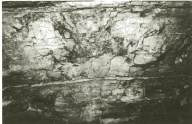
Fig. 6.2.3. Rib wall along cleat in weathered coal.
