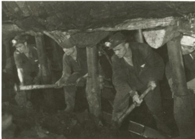
11.1.13. The supports of the roadways is by yielding arches lagged with timber halves.
