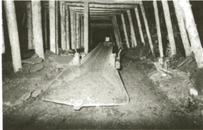
Fig. 7.1.9. Timber support of the chamber at Star-Key Mine (Western Canada).
