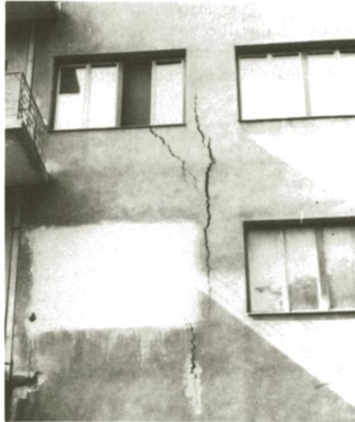
Fig. 12.4.5. Heavily damaged building due to surface subsidence (Tuzla, Yugoslavia).
