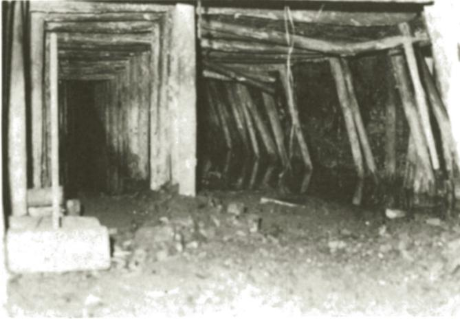
Fig. 7.4.2. Roof span reinforced by external support (timber).
