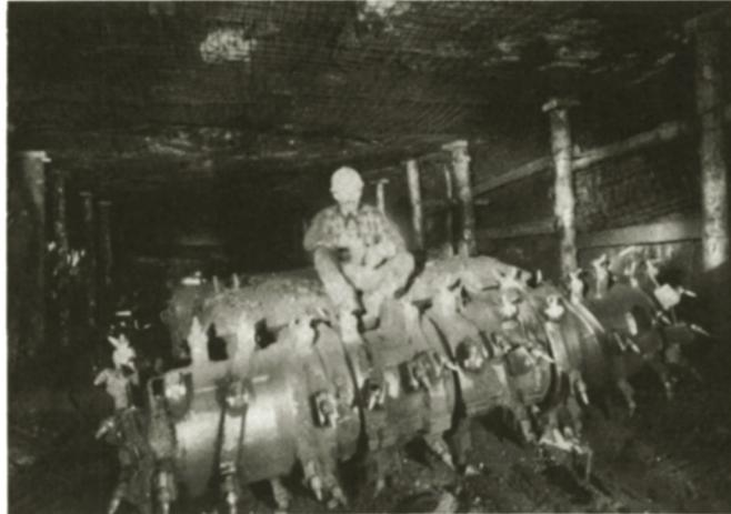
Fig. 7.1.4. Continuous miner at Cliff Terrace Mine of McIntyre Mine (Western Canada).
