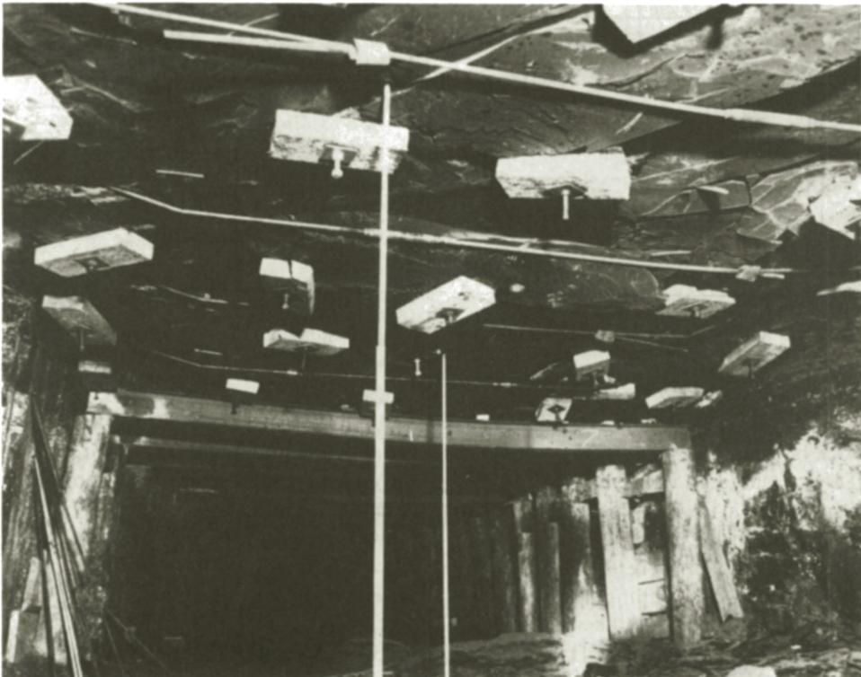
Fig. 4.1.7. Techniques of roof reinforcement, including I-beam frame support.
