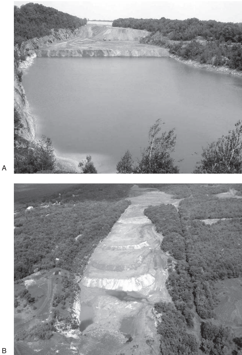
FIGURE 2.8 Big Gorilla pit showing the dry-to-wet placement of approximately three million tons of FBC ash into standing mine water. (A) Big Gorilla in the midst of the placement project. (B) Aerial shot of the filled Big Gorilla pit.
