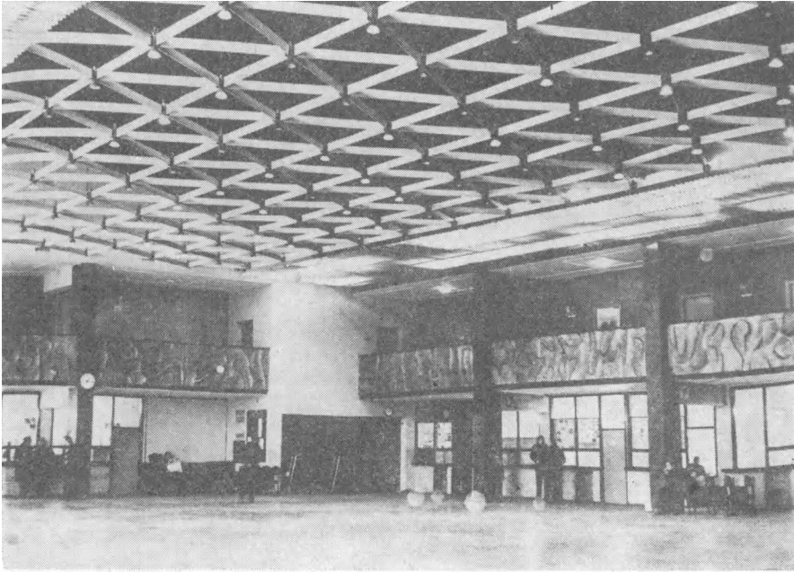
Fig. 6.4 Assembly hall of "Moszczenica" mine.
