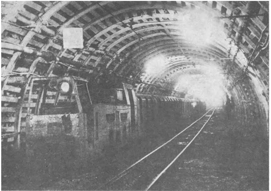
Fig. 5.12 Standardized underground railway station.
