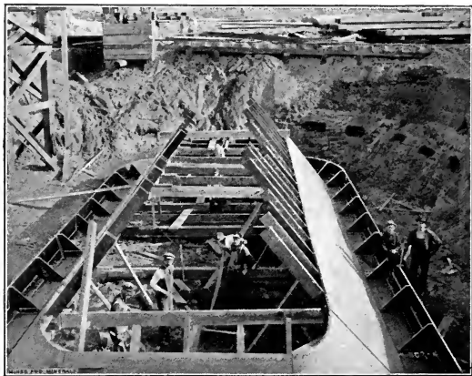
FIG. 22. — Shoe and Form for Bottom of D., L. & W. Caisson
