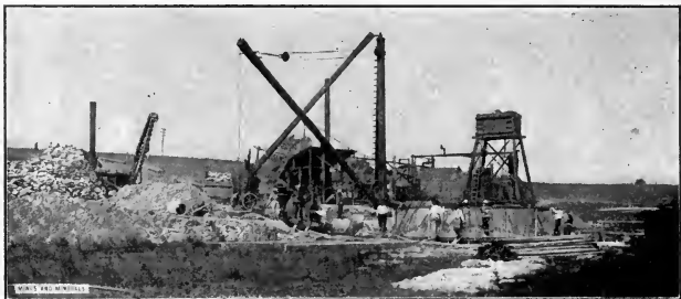
FIG. 17. — Derrick and Head Works Rondout Caisson
