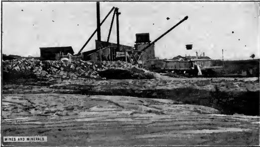
FIG. 18. — Dump, Rondout Caisson, Showing Flowing Nature of Material
