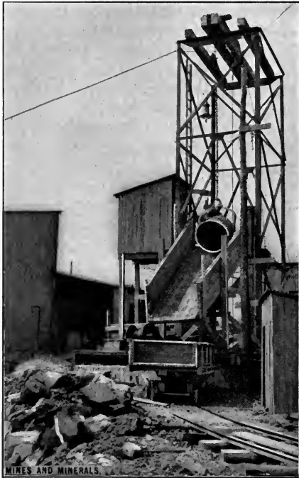
FIG. 5. — Sinking Head-frame showing Dumping Arrangement
