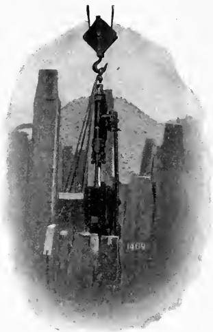
FIG. 12. — Sheet-pile Driver
