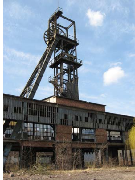
Figure 3. Coal mine “Sosnowiec” closed in 1997, Upper Silesia (Southern Poland) (Photographer: Iga Lewin).
