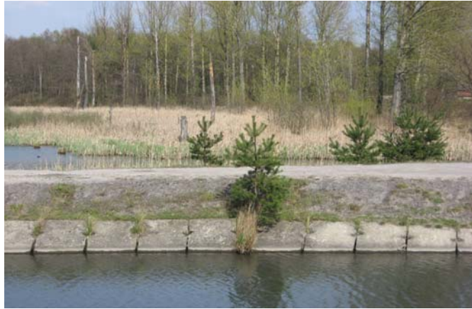
Figure 6. Mining subsidence reservoirs: reclamation- waterbanks concrete-lined and stabilized with waste rock and slag, Czułów, Upper Silesia (Photographer: Iga Lewin).
