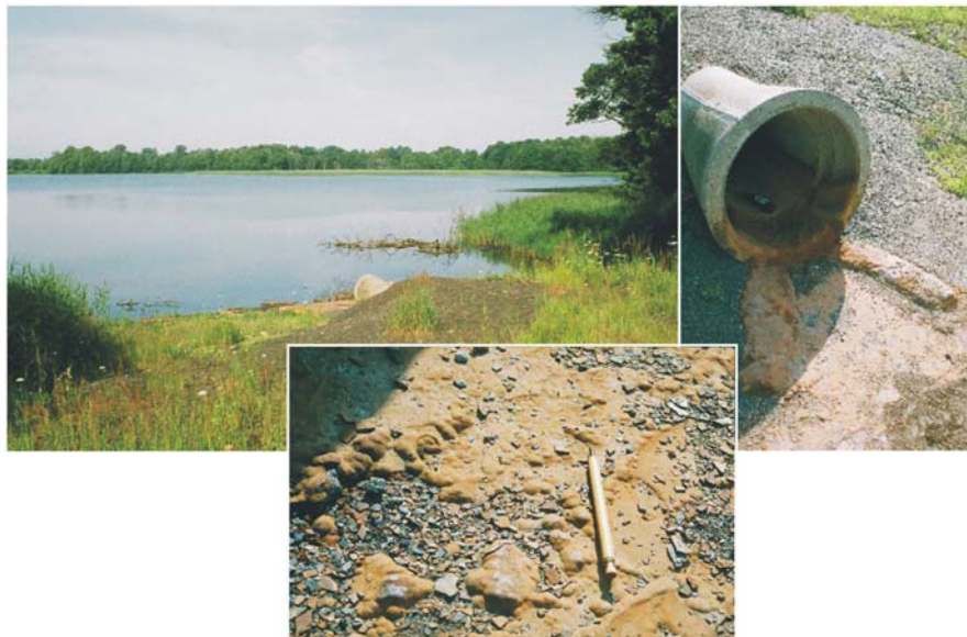
Figure 2. Scales consisting of radiobarite at the discharge point into the former Rontok tailing pond in the USCB in 2005.
