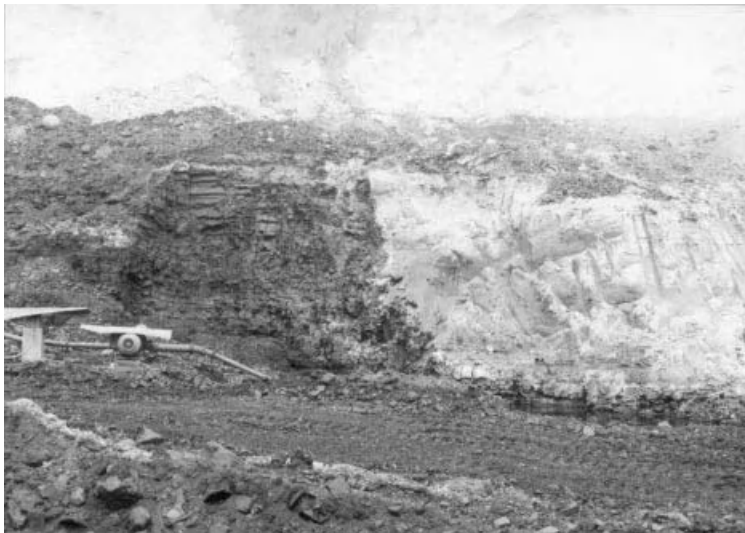
Figure 2.37 Normal fault downthrowing overburden (light colour) against a coal seam. In an opencast mine in central India: height of face is 10 m. (Photograph by courtesy of Dargo Associates Ltd.)
