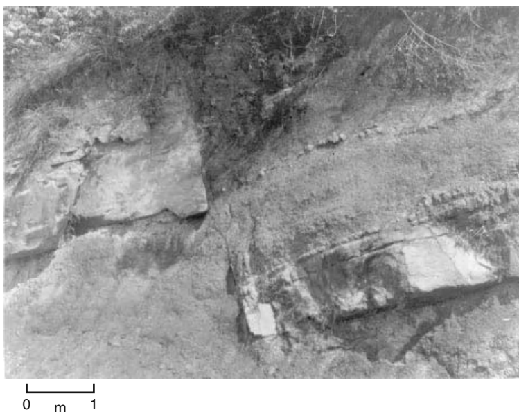
Figure 2.35 Normal fault with downthrow of 2 m to the right. Paleogene–Neogene coal-bearing sediments, Sumatra, Indonesia. (Photograph by LPT.)
