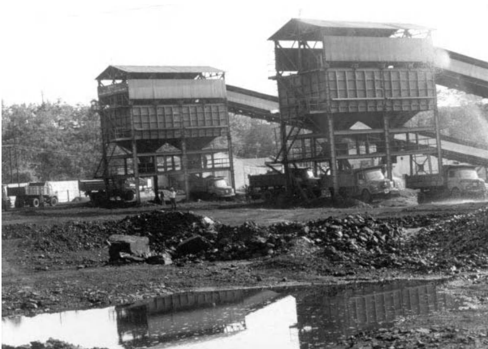
Figure 13.6 Automatic loading of trucks from overhead bins, Orissa State, India. (Photograph by courtesy of Dargo Associates Ltd.)
