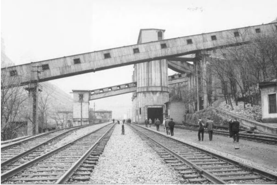
Figure 13.2 Coal silos for loading coal directly to trains, People's Republic of China. (Photograph by courtesy of Dargo Associates Ltd.)
