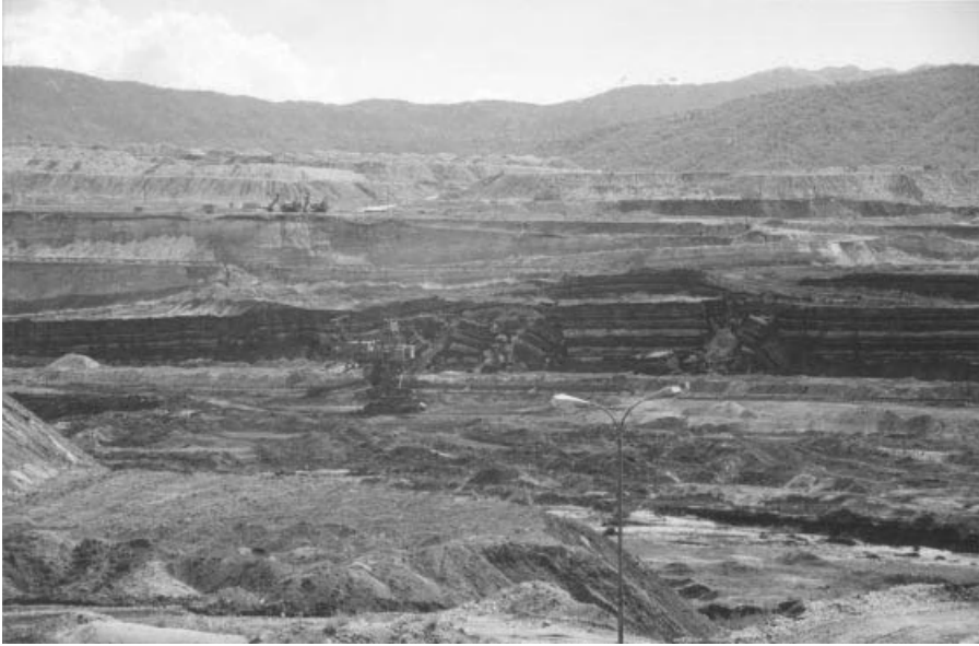
Figure 12.4 Opencast mine in Bosnia-Herzegovina showing large scale overburden removal. Note small scale failures of the high wall caused by surface water action during periods of mining inactivity. (Photograph by courtesy of Dargo Associates Ltd.)
