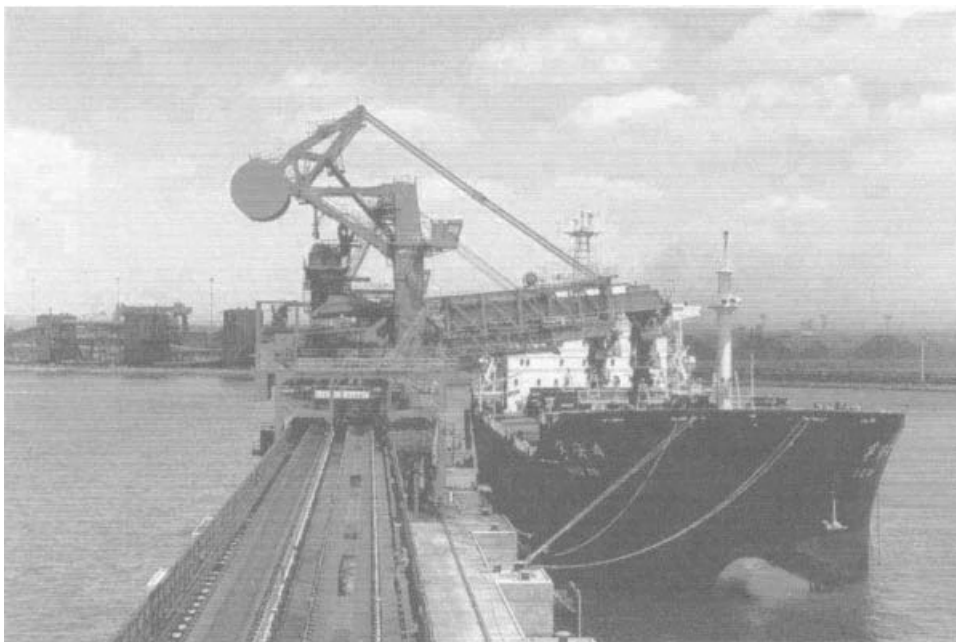
Figure 13.13 Coal loading directly into the ship from the stockyard conveyor system, port of Qinhuangdao, People's Republic of China. (From Thomas and Frankland, 1999.)
