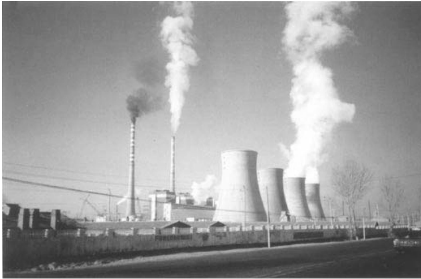
Figure 12.13 Modern coal-fired power station, Inner Mongolia, People's Republic of China. (Photograph courtesy of Dargo Associates Ltd.)
