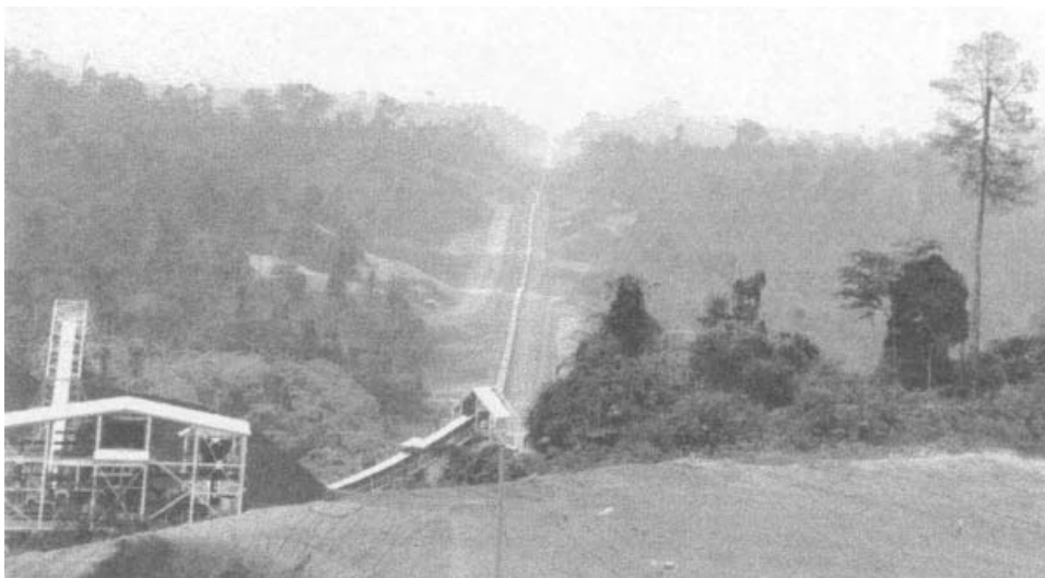
Figure 13.4 Overland conveyor, 14 km in length, from Kaltim Prima Coal mine to the port of Tanjung Bara, East Kalimantan, Indonesia. (Photograph by courtesy of Dargo Associates Ltd.)
