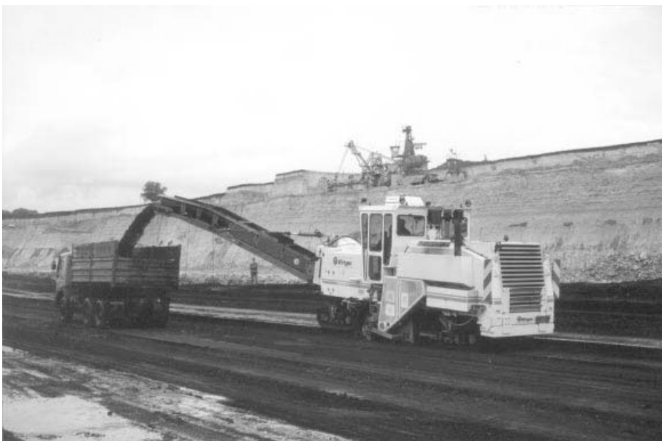
Figure 10.22 Wirtgen surface strip miner in operation in Gacko mine, Bosnia-Herzegovina. (Photograph by courtesy of Dargo Associates Ltd.)
