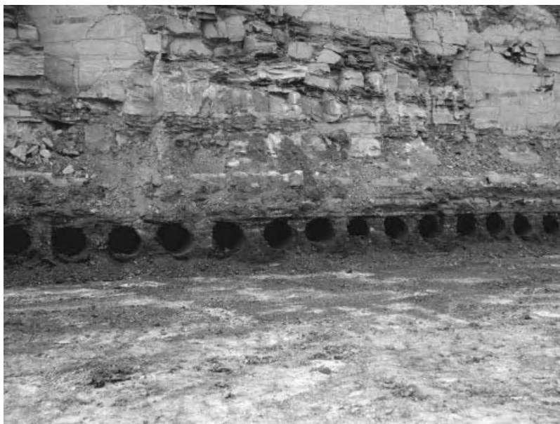
Figure 10.24 Auger mining in Bottom Busty seam, Shotton opencast mine, Northumberland, United Kingdom. Auger holes have 0.45 m diameter. (Photograph by courtesy of M. C. Coultas.)
