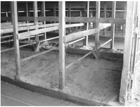
Fig. 6.10. An example of cubicle renovation. All woodwork has been removed from the front of the cubicle and the lower dividing rail has been replaced by a tensioned strap allowing cows to share space and lunge both sideways and forwards. Cows are positioned by a brisket board and a new neck rail (of tensioned rope) set far forward in the stall. The old bed has been replaced by deep sand. While the cubicles remain short, cow comfort has been dramatically improved and the functional life of the building extended at relatively low cost.
