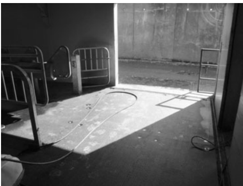
Fig. 6.11. Rubber matting fitted in the parlour and on right-angled turns at the parlour exit.
