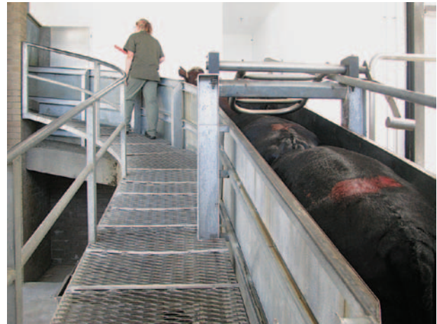
Figure 2.1: Ramp with closed sides leading to the slaughter point. Source: CSIRO Food and Nutritional Sciences.
