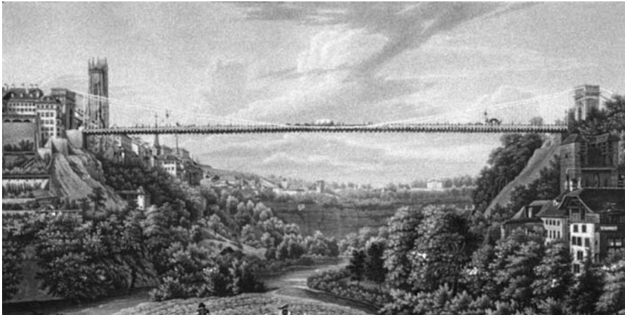
Fig. 3.3 Pont de Fribourg (CH). Engineer Joseph Chaley (Photo IBK, ETH – Zurich).
