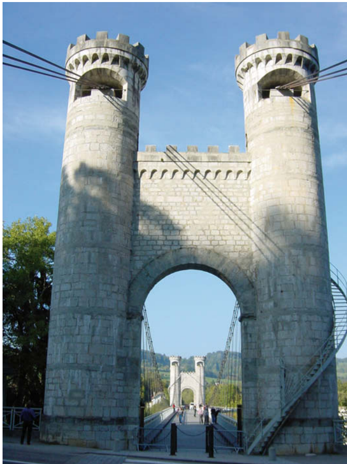
Fig. 3.4 Pont de la Caille (F). Engineer E. Belin (Photo ICOM).
