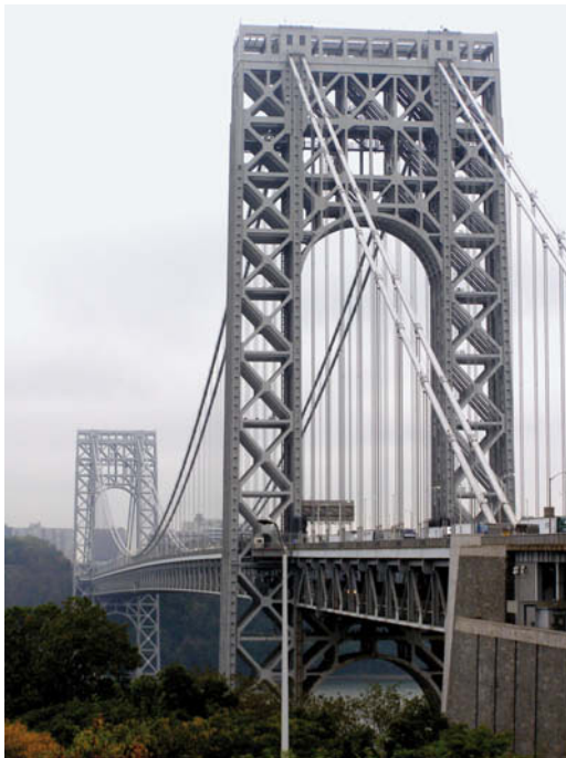
Fig. 3.9 George Washington Bridge (USA). Engineer Othmar H. Ammann (Photo Bojidar Yanev).
