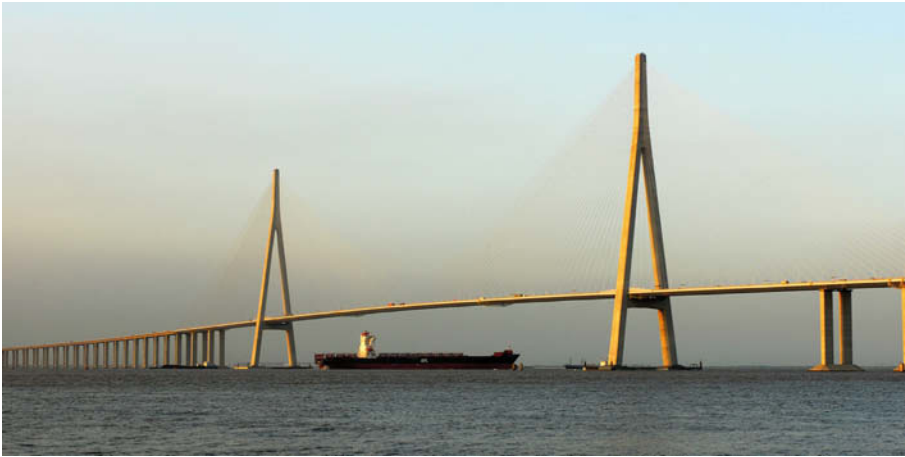
Fig. 3.21 Sutong Bridge (PRC). Engineer Jiangsu Provincial Communications Planning and Design Institute (Photo Yaojun Ge).
