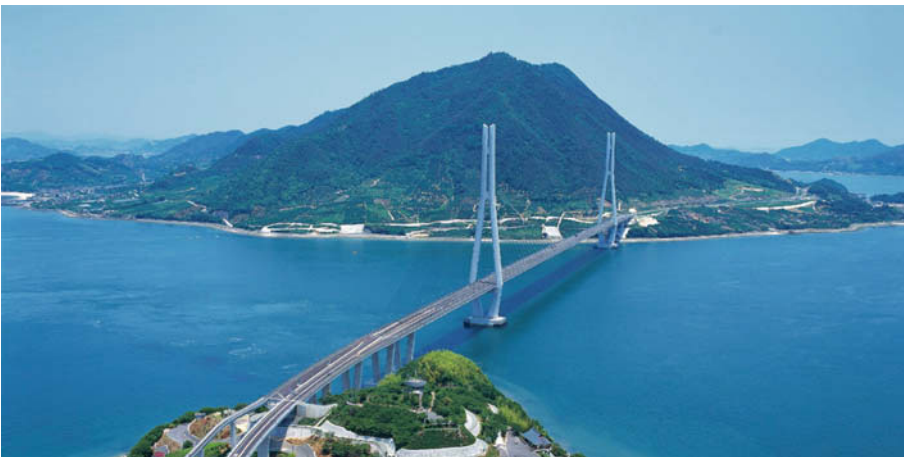
Fig. 3.16 Tataro Bridge (J). Engineer Honshu-Shikoku Bridge Authority (Photo Honshu-Shikoku Bridge Expressway Company).
