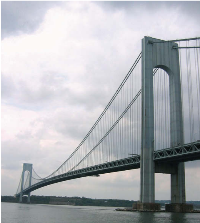
Fig. 3.11 Verrazano-Narrows Bridge (USA). Engineer Othmar H. Ammann (Photo Bojidar Yanev).
