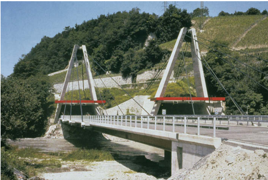
Fig. 3.18 Bridge over the Rhone at St Maurice (CH). Engineer René Walther (Photo ICOM).
