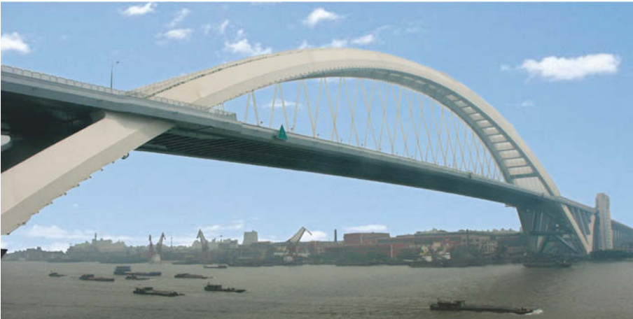
Fig. 3.15 Lupu Bridge (PRC). Engineer Shanghai Municipal Engineering Design Institute (Photo Yaojun Ge).
