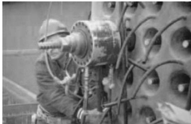
Fig. 15.5 Post-tensioning bars.
