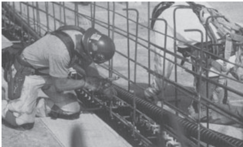
Fig. 15.4 Pre-tensioning of tendons.
