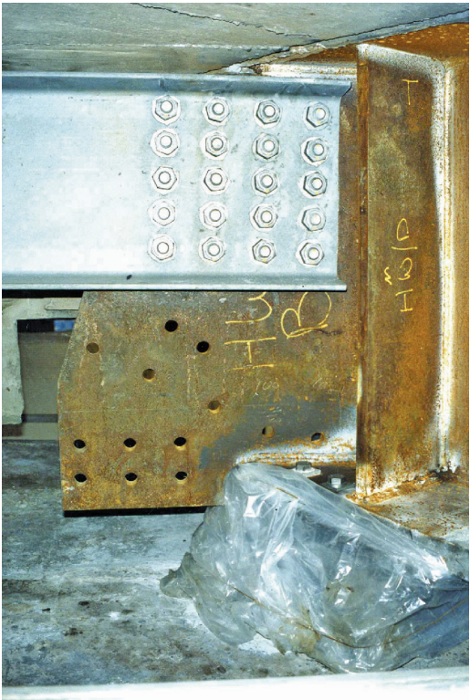
Figure 15.9 – Trimmer beam
