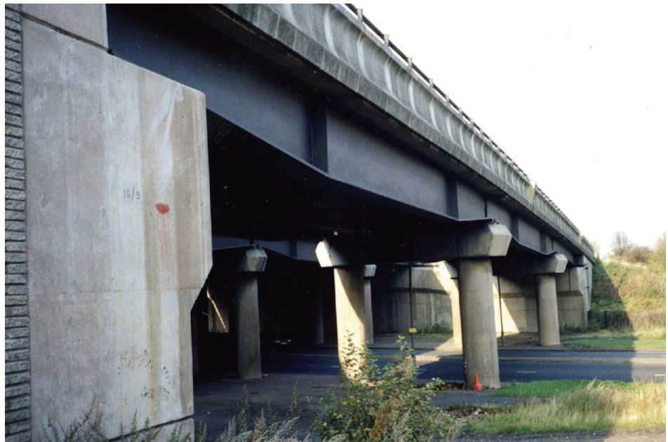
Figure 15.4 – Viaduct supported on skewed crossbeams
