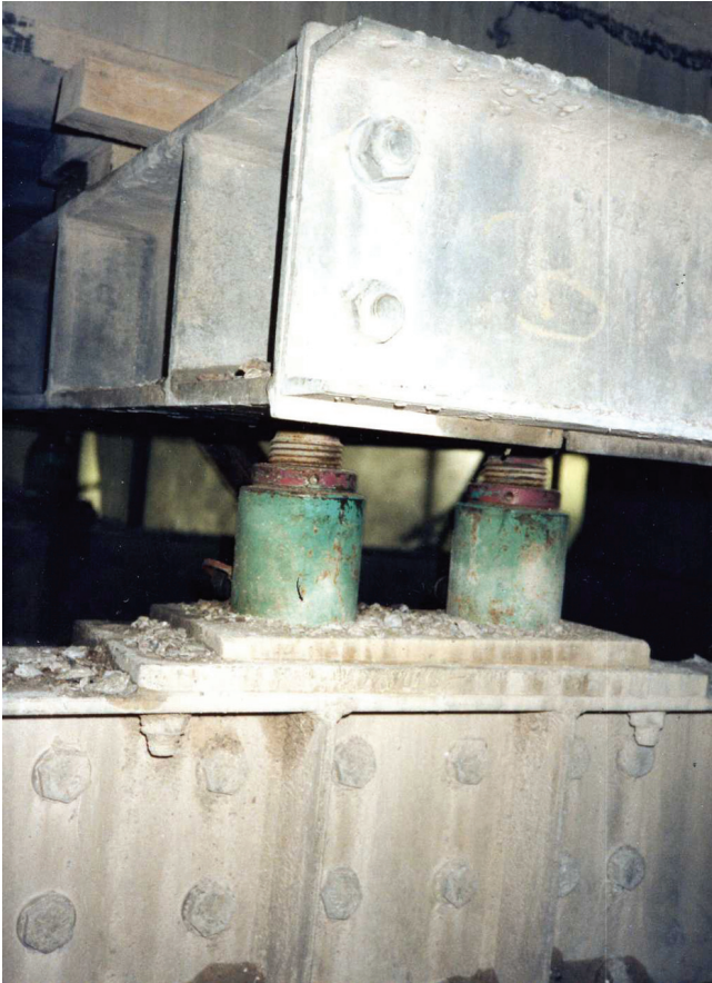
Figure 4.8 – Jacking beam jacks
