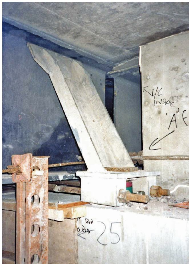
Figure 6.1 – A-frame for repair below bearing
