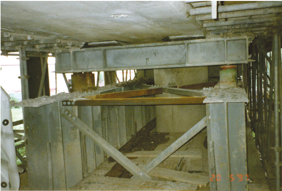
Figure 4.7 – Temporary jacking beam
