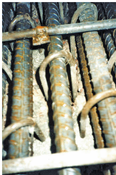
Figure 4.1 – New length of torsion bar butt welded into position
