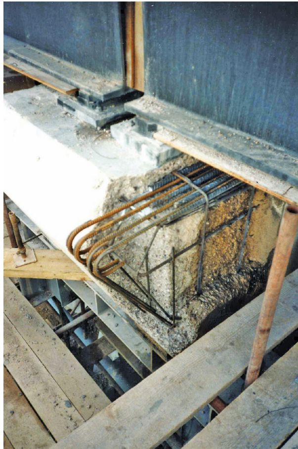
Figure 6.5 – Concrete nib reinforcement
