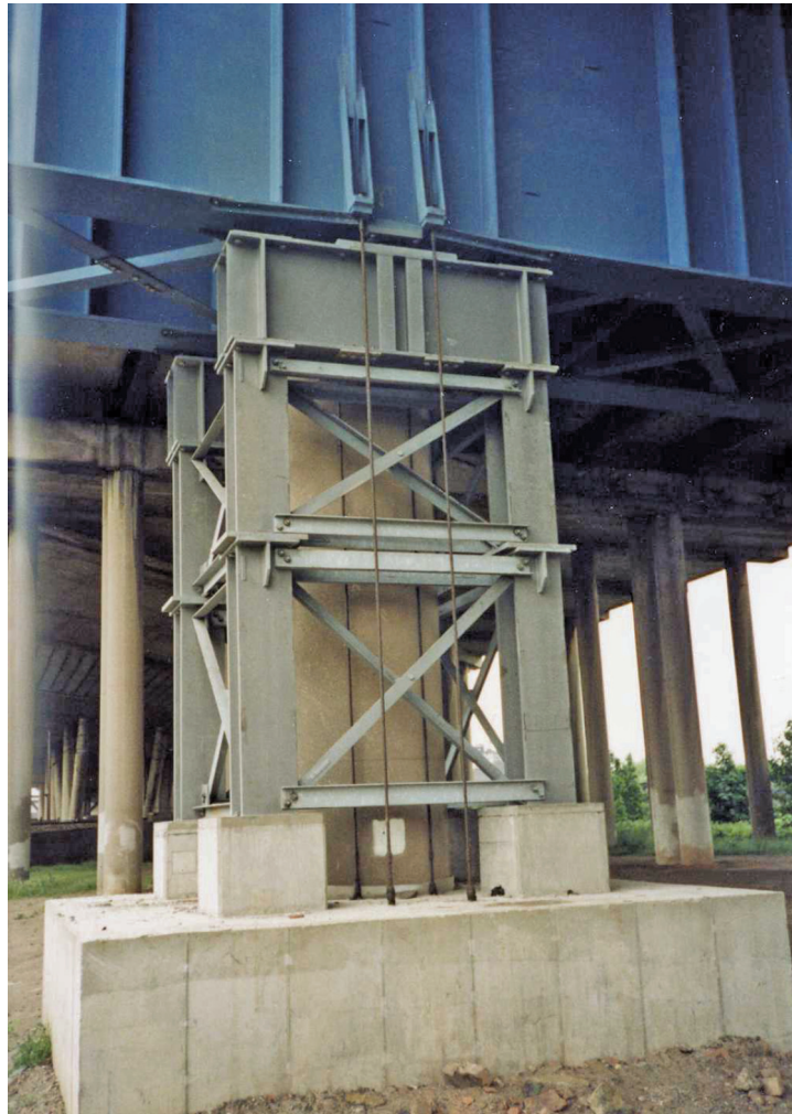
Figure 1.11 – Plate girder tied down to counterweight
