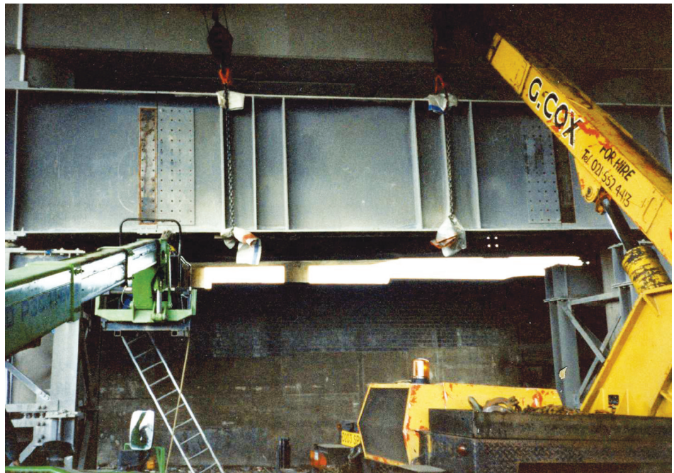
Figure 4.5 – Temporary plate girder being erected
