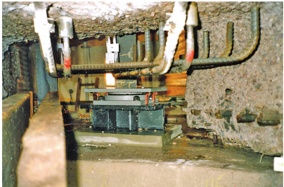
Figure 15.2 – Reinforcement for bearing downstand
