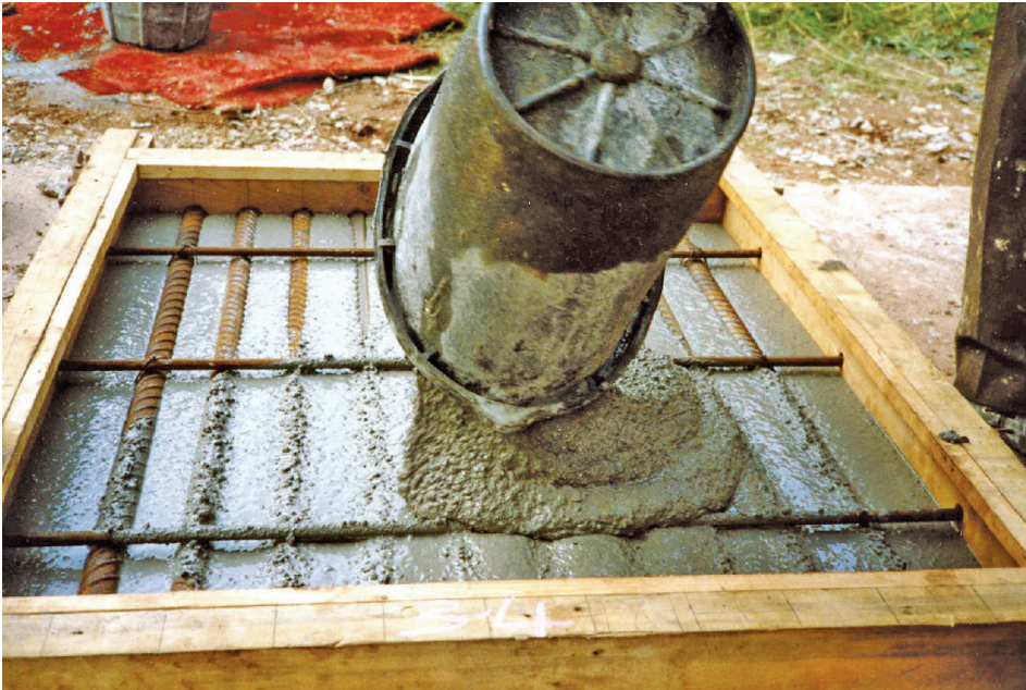
Figure 4.13 – Flowing concrete trial for crossbeam top
