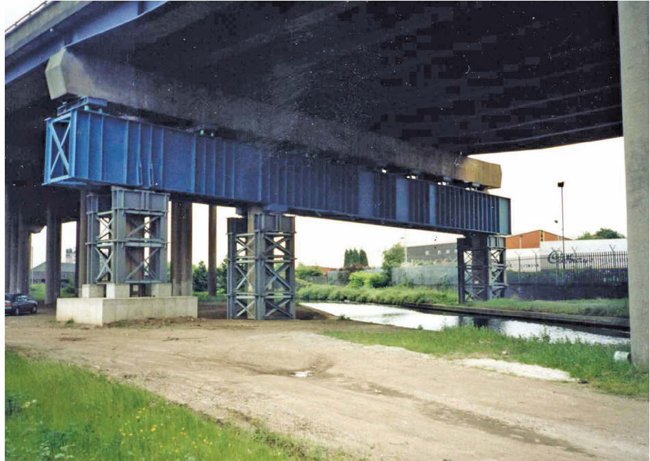
Figure 1.10 – Plate girder erected across canal
