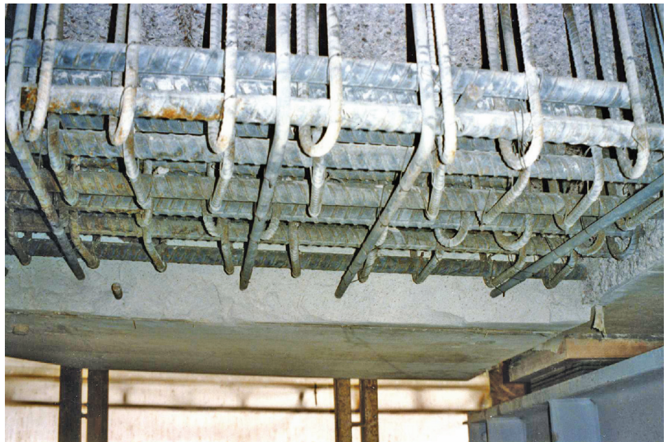
Figure 4.9 – Soffit break out
