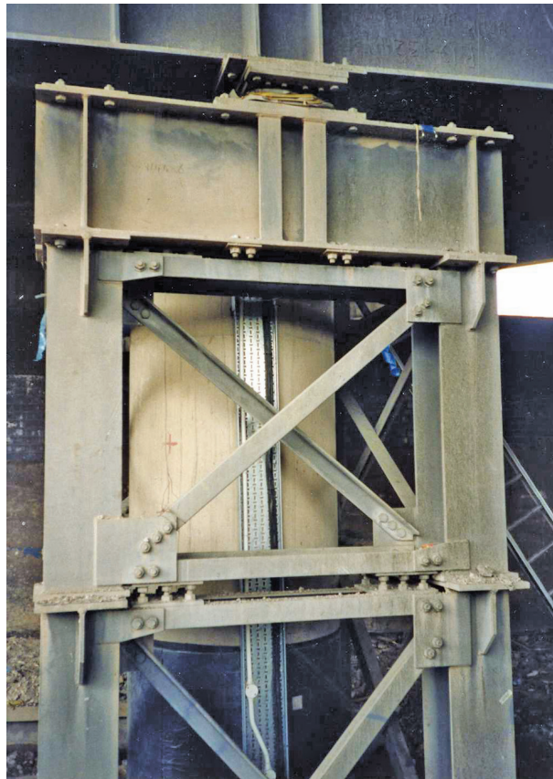
Figure 4.6 – Temporary steel trestle
