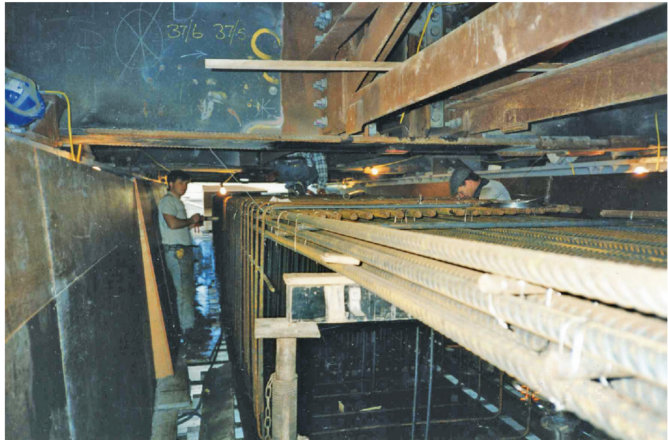
Figure 2.15 – Steel fixing for replacement crossbeam
