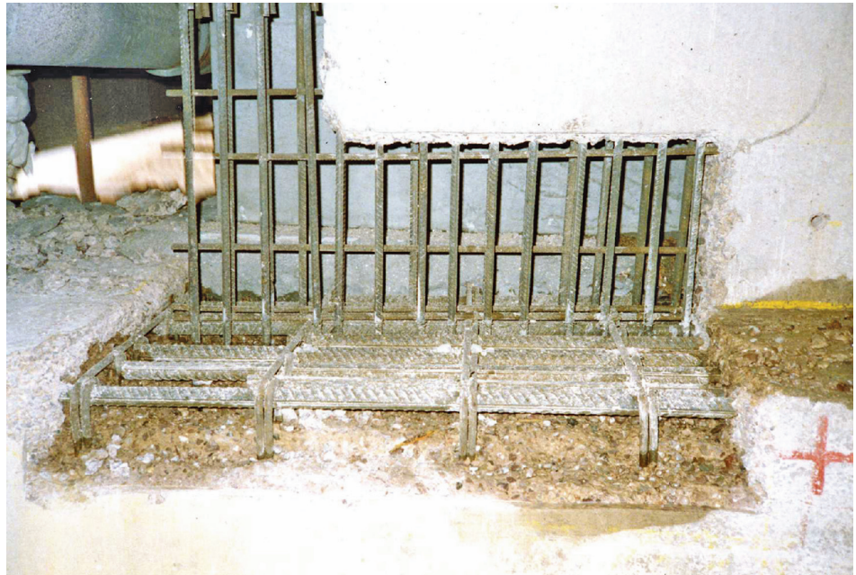
Figure 3.3 – Concrete removed from panel wall by waterjetting
