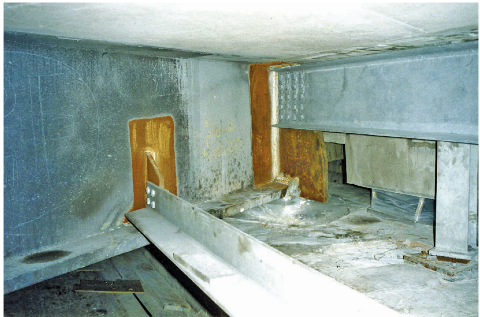
Figure 15.8 – Bracing to bottom flange. (Also trimmer beam)
