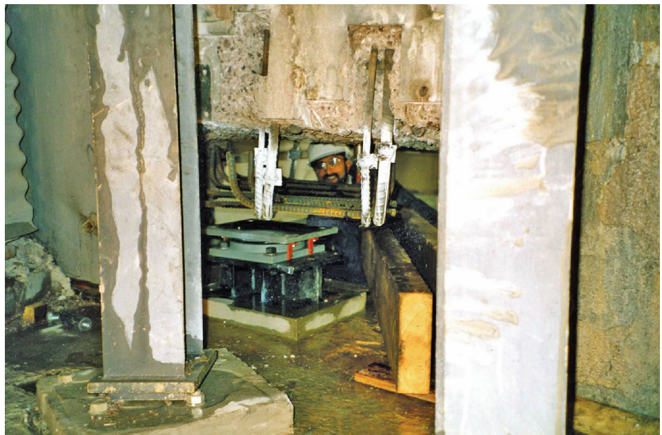
Figure 15.3 – Reinforcement for bearing downstand
