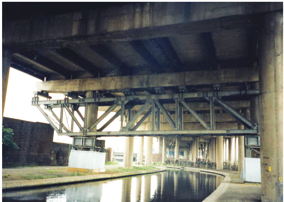
Figure 4.3 – Temporary truss support
