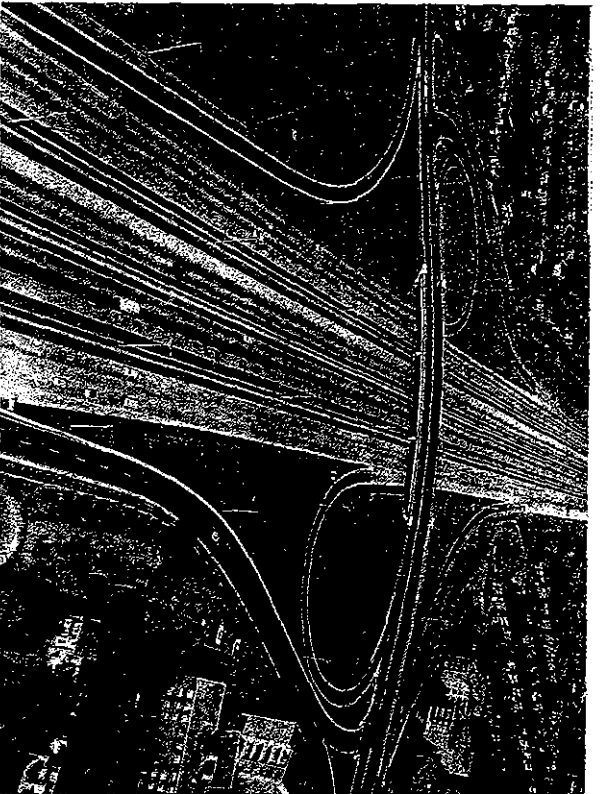
Fig. 31.2 Intersection of Highway 401 and Avenue Road, Toronto
