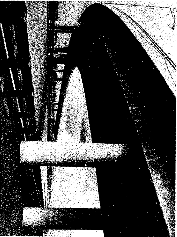
Fig. 31.7 A bridge at junction of Highways 400 and 401, Toronto
