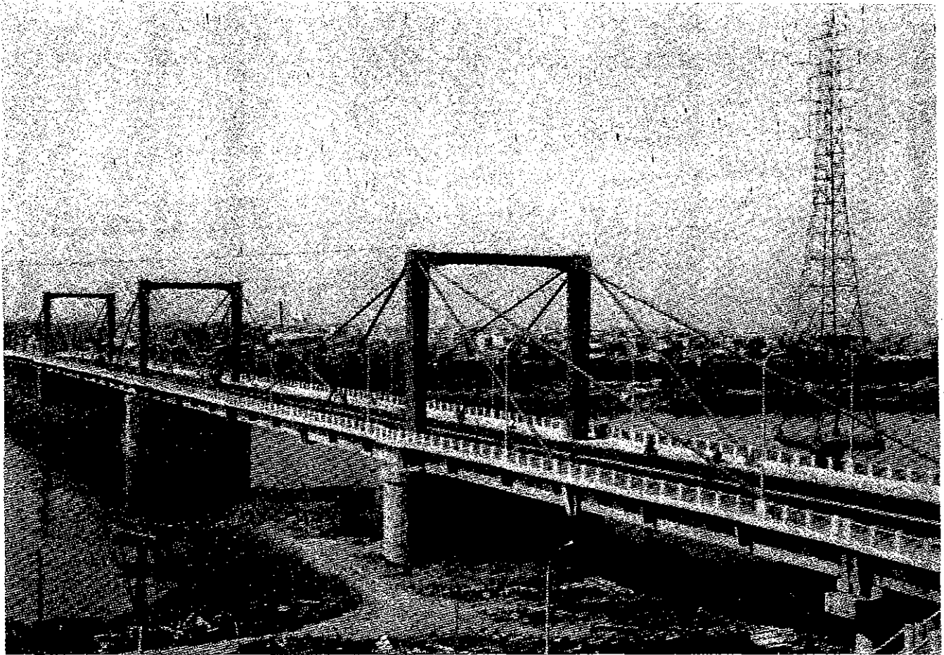
KWANG FU BRIDGE
