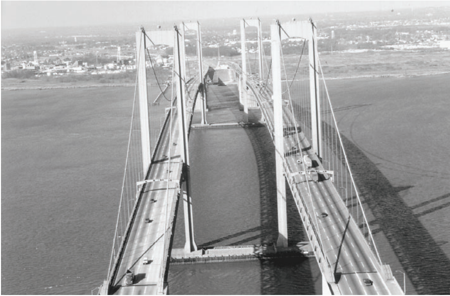
FIGURE 3.5 Delaware Memorial Bridges. (Courtesy of D. Sailors.)
