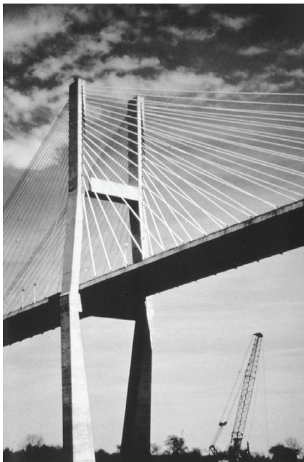
FIGURE 3.8 Talmadge Bridge, Georgia. (Courtesy of T. Y. Lin International.)
