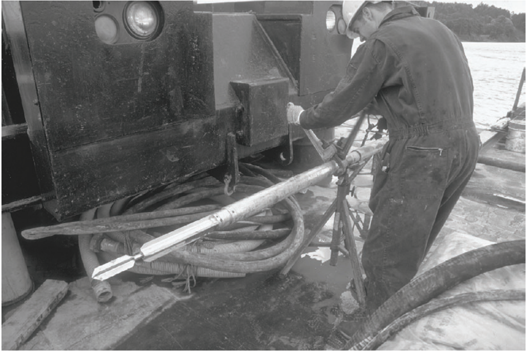
FIGURE 5.5 In situ vane shear device.
