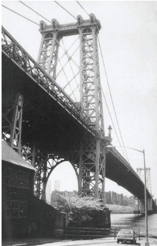
FIGURE 3.4 Williamsburg Bridge, New York. (Courtesy of Charles Seim.)
