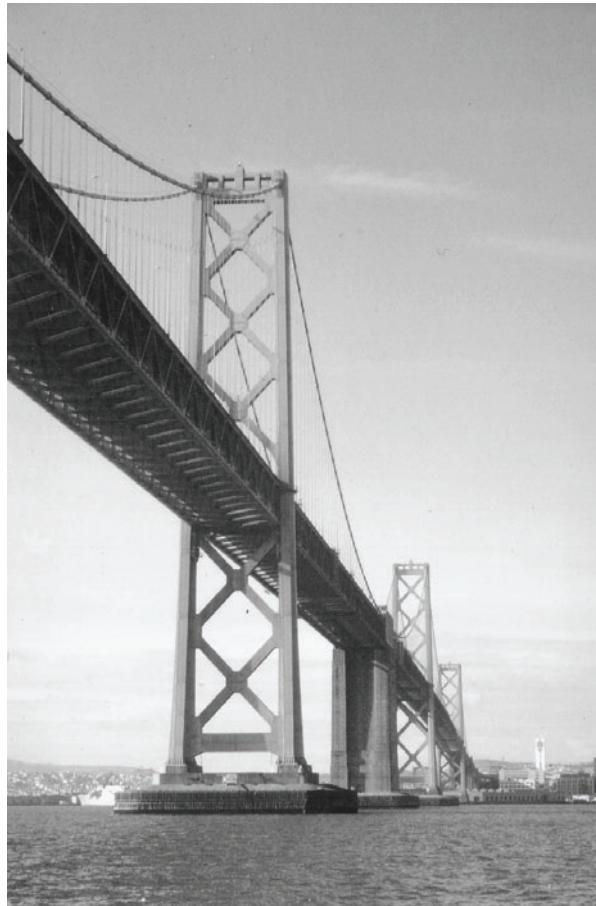
FIGURE 3.2 San Francisco–Oakland Bay Bridge. (Courtesy of Charles Seim.)
