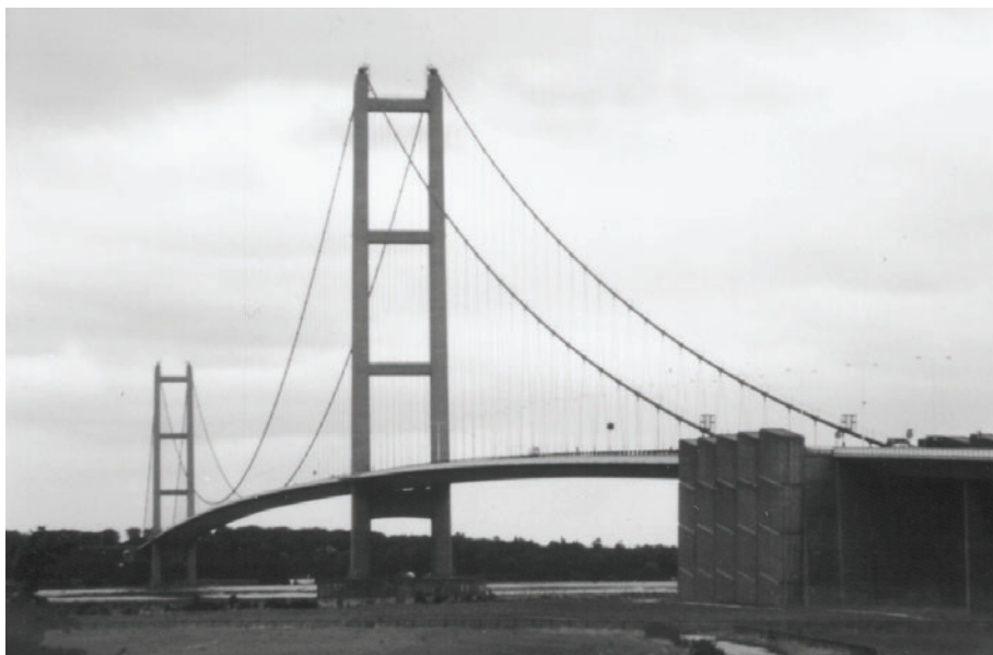
FIGURE 3.12 Humber Bridge, England. (Courtesy of Charles Seim.)
