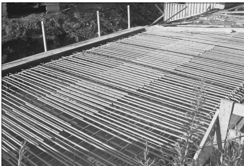
Figure 3.23 Reinforcing steel for a concrete deck slab about to be poured.
