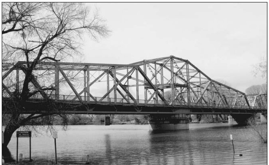
Figure 1.14 American River Bridge near Sacramento, California.
