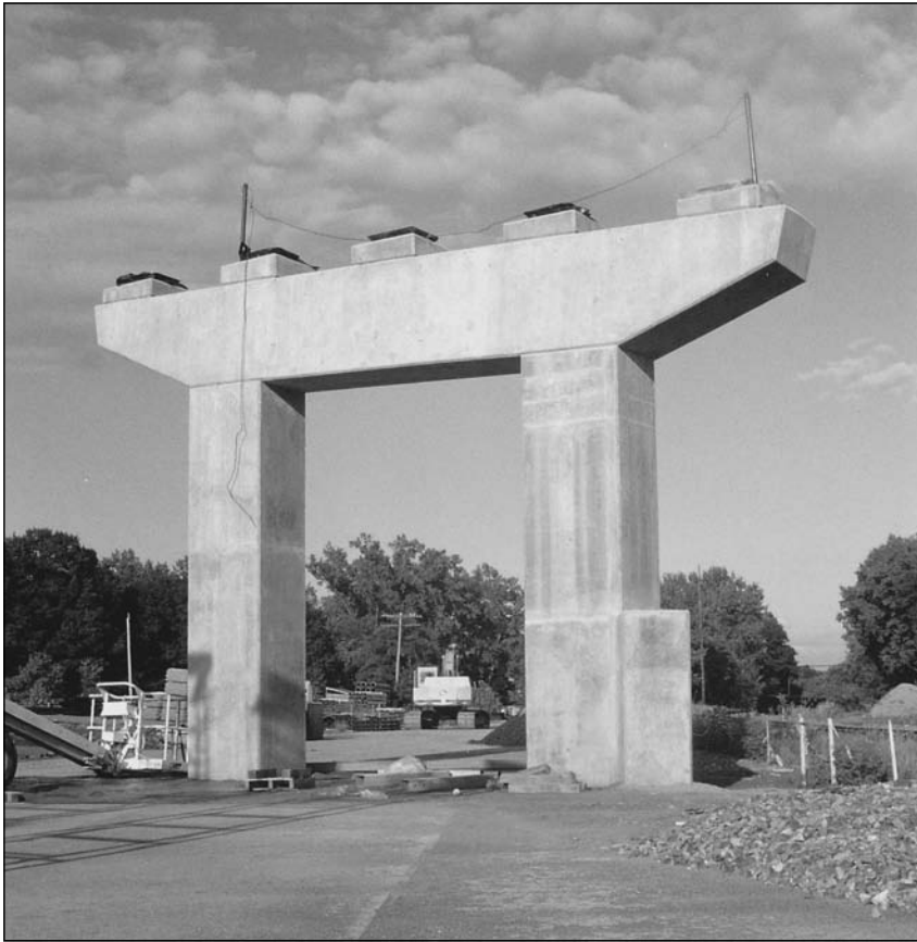
Figure 4.8 A two column, concrete hammerhead pier under construction.
