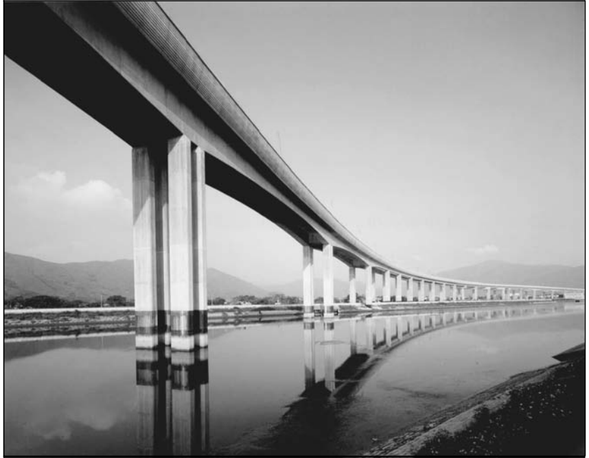
Figure 1.11 KCRC West Rail Viaducts, Hong Kong.
