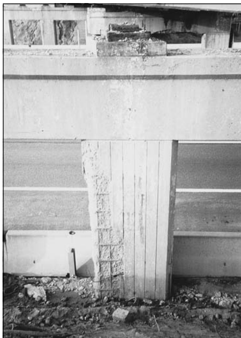
Figure 2.6 Exposed reinforcing signals repair.
