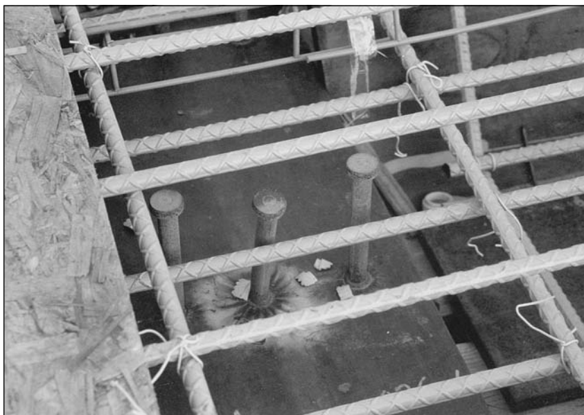
Figure 3.30 A shear stud installed at the top flange of a plate girder. Shear connectors are the key ingredient to preventing slippage and creating composite action.
