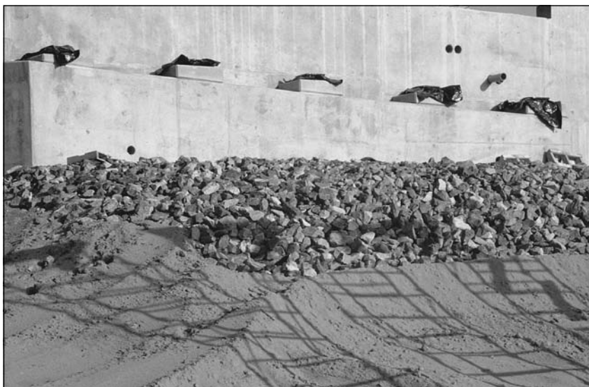
Figure 1.9 Broken rocks, varying in size, can be used as slope protection.
