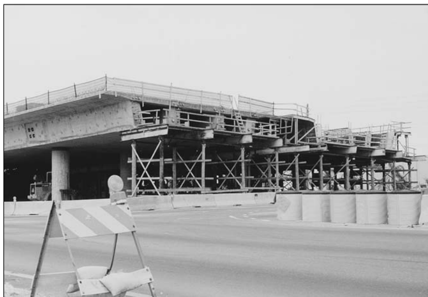
Figure 3.56 A prestressed concrete box structure under construction.
