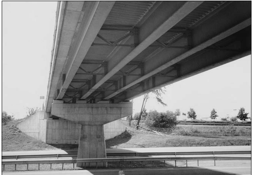
Figure 1.5 A hammerhead pier supports a slab-on-stringer superstructure.
