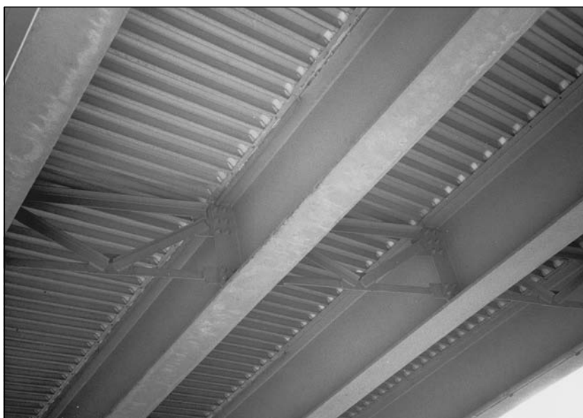
Figure 2.8 Stay-in-place forms can hide deterioration beneath them.
