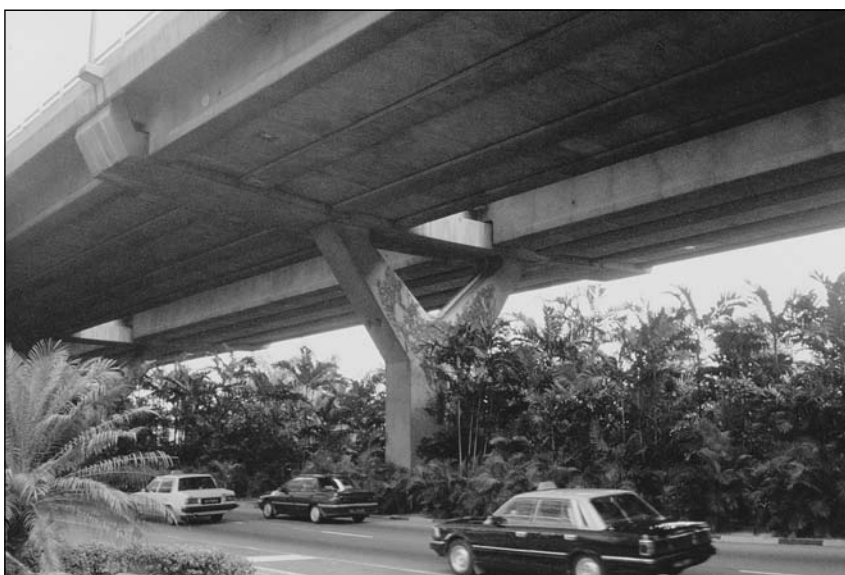
Figure 3.50 A prestressed concrete bridge carries dual roadways over a busy underpass in Singapore.
