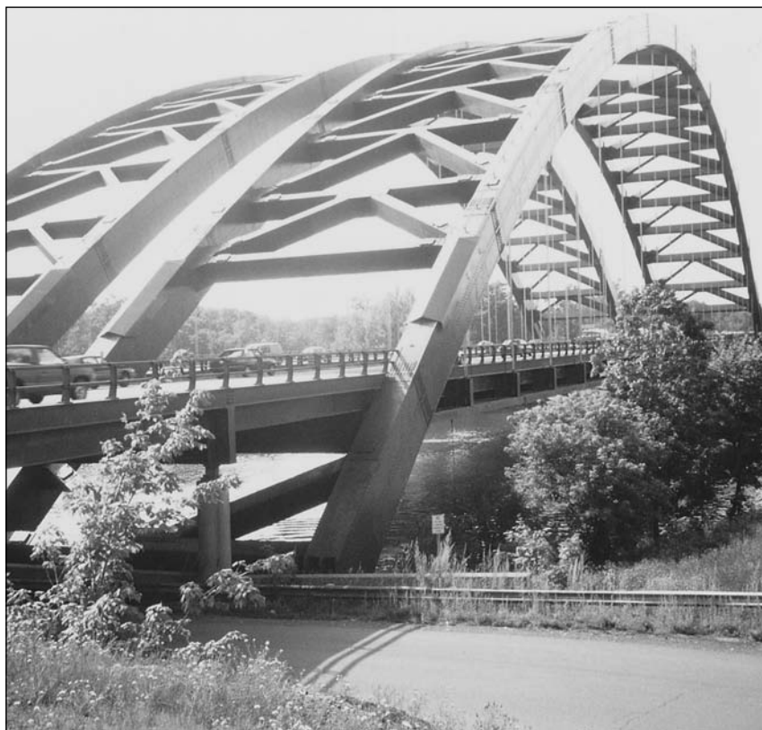
Figure 1.13 Twin steel through arches cross the Mohawk River in upstate New York.
