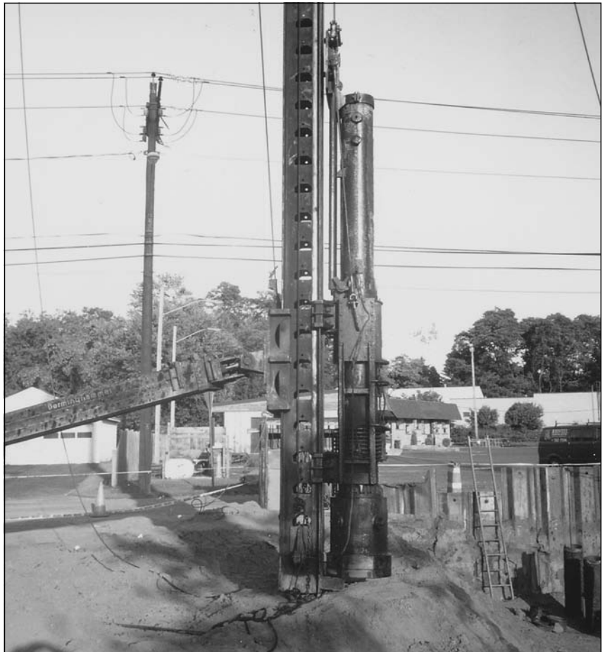
Figure 1.7 Driving piles for a new abutment in a bridge replacement project.
