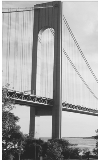
Figure 1.1 The type of bridge we won't be talking about in this text.
