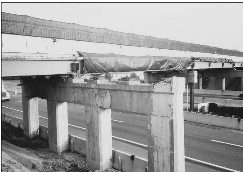
Figure 1.10 A bridge undergoing staged construction for a rehabilitation.
