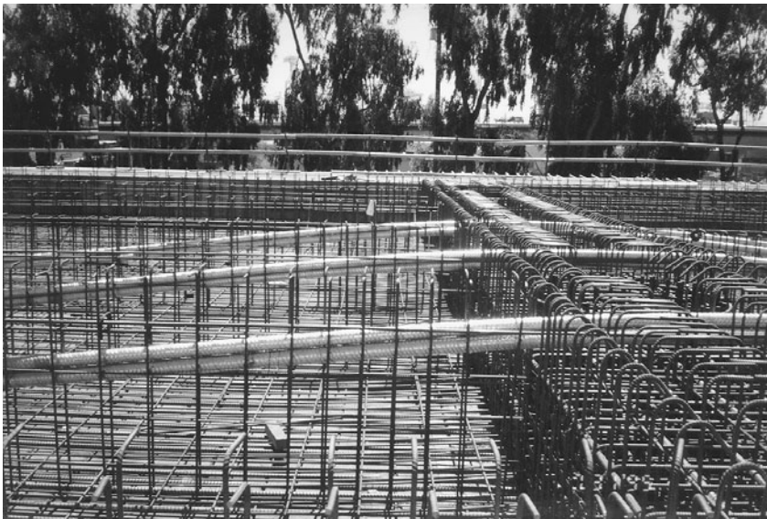
FIGURE 4.6 Bridge soffit and girder reinforcements with prestressing duct profile.
