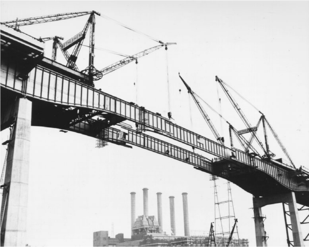
FIGURE 1.29 Erecting closing girder sections of Passaic River Bridge, New Jersey Turnpike, 1951. Huge double-boom travelers, each weighing 270 tons, erect closing plate girders of the 375 ft (114 m) main span. Closing girders are 14 ft (4.3 m) deep and 115 ft (35 m) long and weigh 146 tons each. Sidewise entry was required (as shown) because of long projecting splice material. Longitudinal motion was provided at one pier, where girders were jacked to effect closure. Closing girders were laterally stable without floor steel fill-in, such that derrick falls could be released immediately. (Courtesy of Bethlehem Steel Corporation.)
