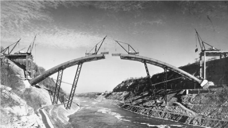
FIGURE 1.4 Lewiston-Queenston arch bridge, near Niagara Falls, New York, 1962. The longest fixed-arch span in the U.S. at 1000 ft (305 m); rise is 159 ft (48 m). Box arch-rib sections are typically about 3 \times 13\text{-}1/2 ft ( 0.9 \times 4.1 m) in cross-section and about 44\text{-}1/2 ft (13.6 m) long. Job was estimated using erection tiebacks (same as shown in Figure 1.3 ), but subsequent studies showed the long, sloping falsework bents to be more economical (even if less secure looking). Much permanent steelwork was used in falsework bents. Derricks on approaches load steelwork onto material cars that travel up arch ribs. The 115-ton-capacity travelers are shown erecting the last full-length arch-rib sections, leaving only the short, closing crown sections to be erected. Canada is at left, the U.S. at right. (Courtesy of Bethlehem Steel Corporation.)
