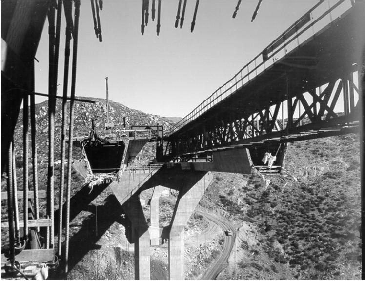
FIGURE 2.4 Pine Valley Creek Bridge — girder construction.
