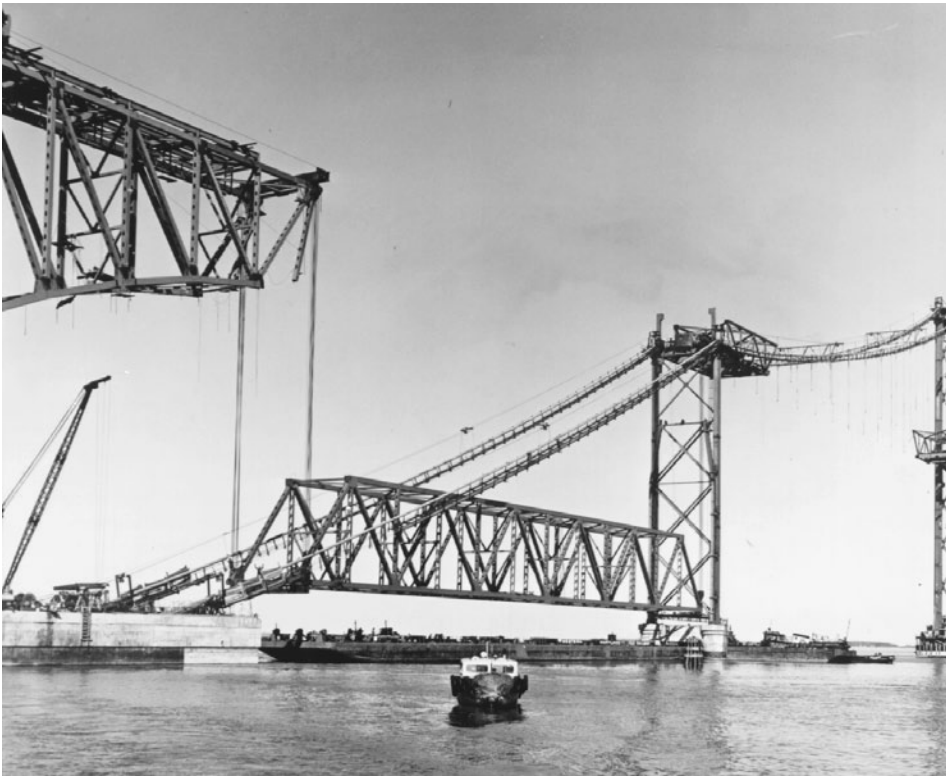
FIGURE 1.32 Erection of a truss span by hoisting, first Chesapeake Bay Bridge, Maryland, 1952. A 360 ft (110 m) truss span is floated into position on barges and picked clear using four sets of lifting falls. Suspension bridge deck is under construction at right. (Courtesy of Bethlehem Steel Corporation.)
