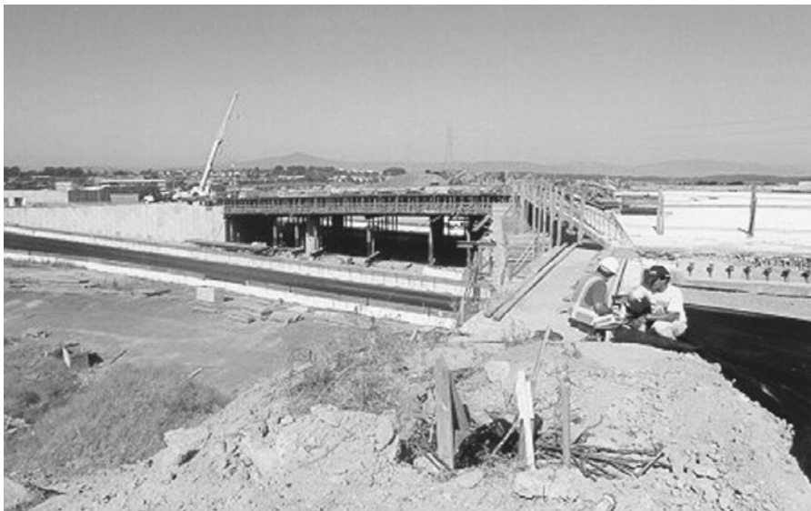
FIGURE 2.6 Falsework at I-80 HOV construction, Richmond, CA.
