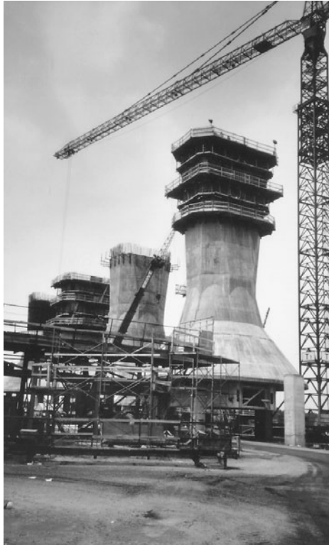
FIGURE 3.26 Prefabricated pier shaft and icebreaker, Prince Edward Island Bridge, Canada.
