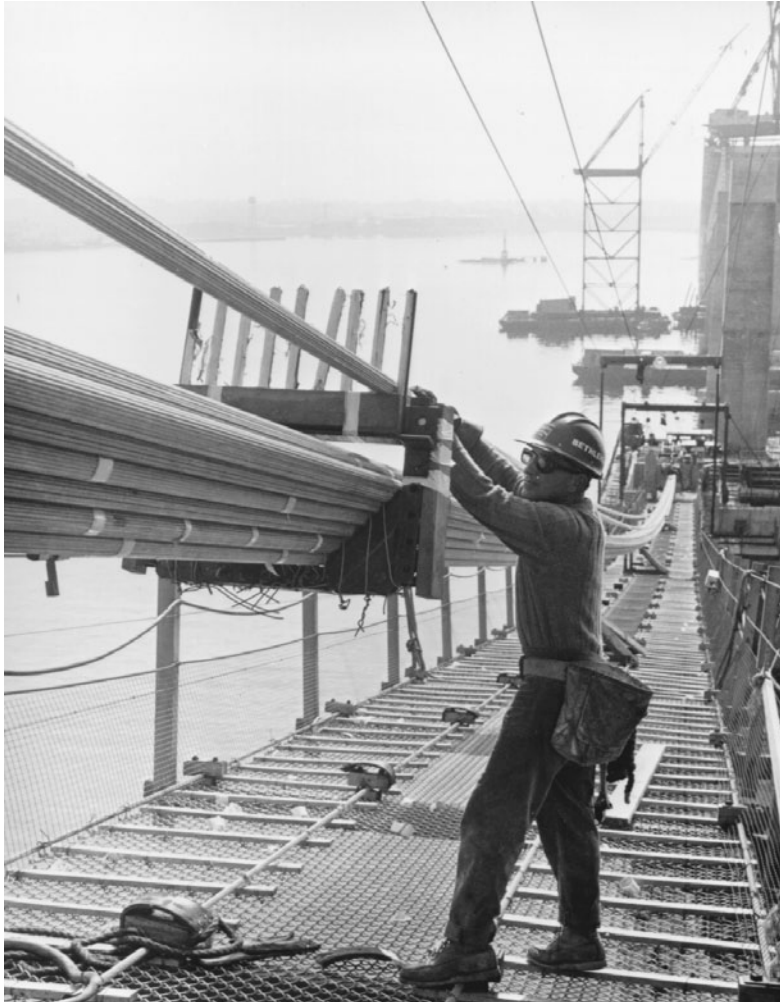
FIGURE 1.37B Cable formers maintain strand alignment in cables prior to cable compaction. Each finished cable is about 15-1/4 in. (387 mm) in diameter. (Courtesy of Bethlehem Steel Corporation.)
