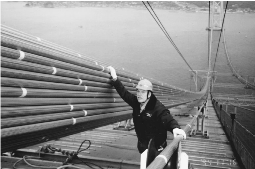
FIGURE 1.46 Parallel-wire-strand main cable, Akashi Kaikyo suspension bridge, Kobe, Japan, 1994. Main span is 6532 ft (1991 m), by far the world's longest. PWS at right is being towed across spans, supported on rollers. Completed cable is made up of 290 PWS, making a total of 36,830 wires, and has diameter of 44.2 in. (1122 mm) following compaction — largest bridge cables built to date. Each 127-wire PWS is about 2-3/8 in. (60 mm) in diameter. (Courtesy of Nippon Steel — Kobe Steel.)
