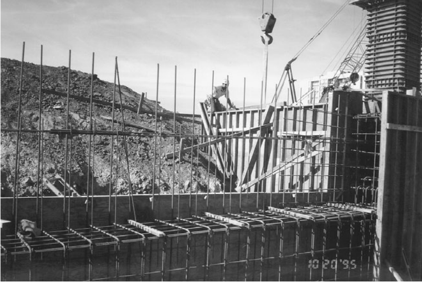
FIGURE 4.3 Wingwall and abutment construction.
