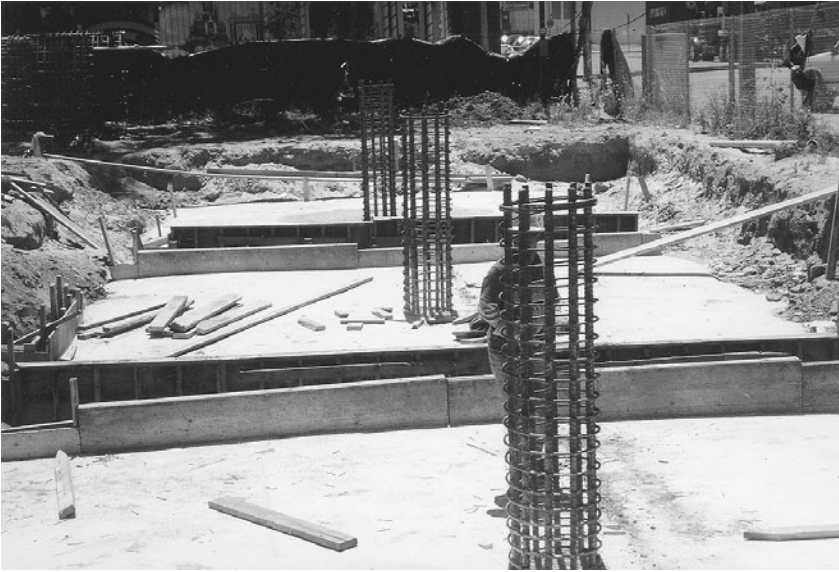
FIGURE 4.1 Foundation forms.
