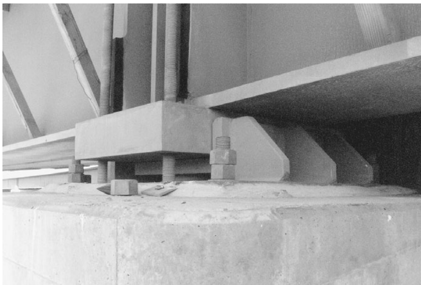
FIGURE 4.8 Bearing assembly of steel plate girder.
