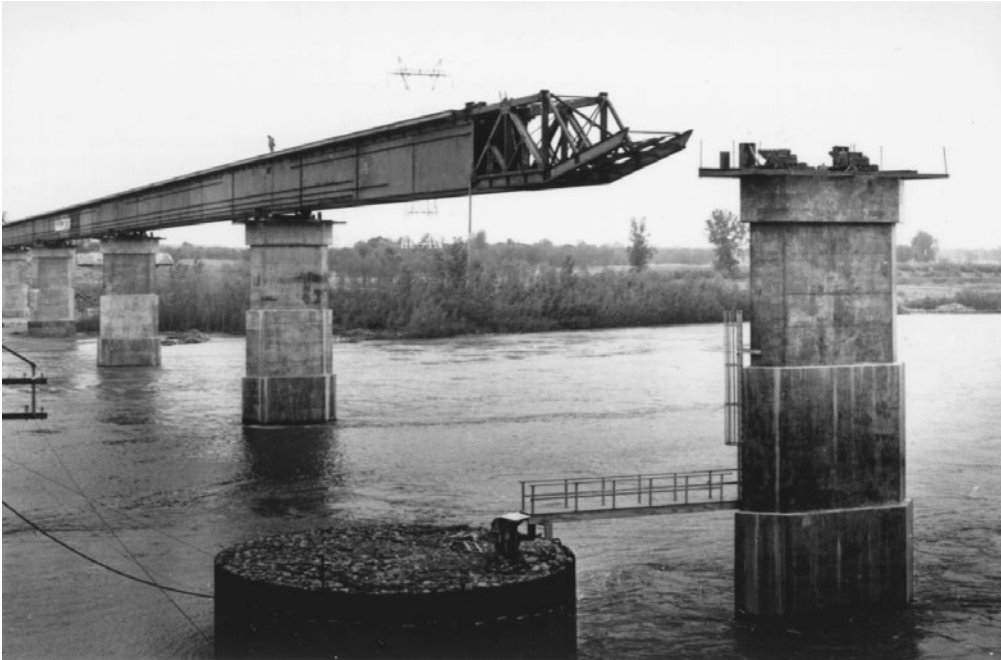
FIGURE 1.41A Leading end of north girder train moves across 250 ft (76 m) span 4, approaching pier 5. Main span, 330 ft (101 m), is to right of pier 5.
