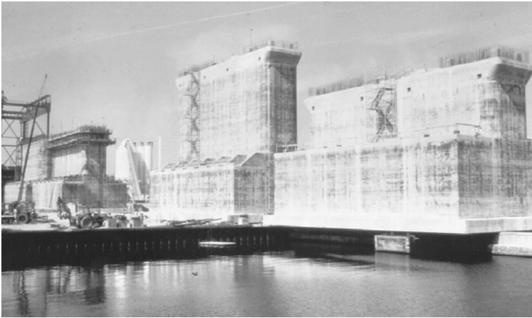
FIGURE 3.22 Prefabricated concrete box caissons are moved by jacks onto pier for load-out.
