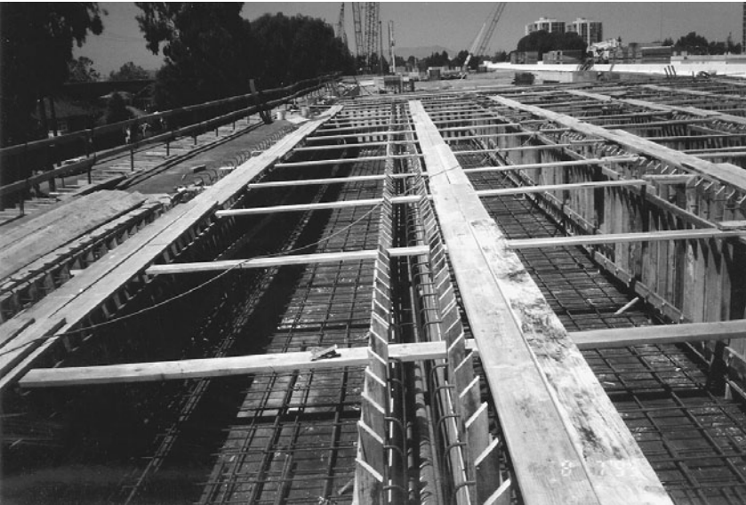
FIGURE 4.4 Bridge stem and soffit forms for concrete box girder.
