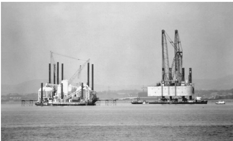
FIGURE 3.28 Installing precast concrete box caissons for Second Severn Crossing, Bristol, England. Extreme tidal range of 10 m and high tidal current imposed severe demands on installation procedures and equipment.
