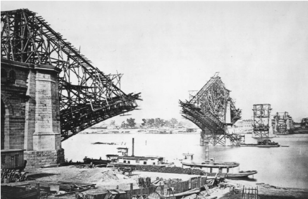
FIGURE 1.15 Eads Bridge across the Mississippi River, St. Louis, Mo., 1873. The first important metal arch bridge in the U.S., it is supported by four planes of hingeless trussed arches having chrome-steel tubular chords. Spans are 502-520-502 ft (153-158-153 m). During erection, arch trusses were tied back by cables passing over temporary towers built on the piers. Arch ribs were packed in ice to effect closure.
