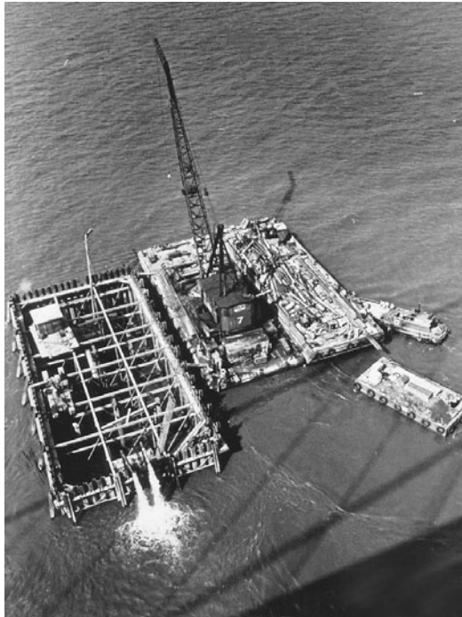
FIGURE 3.12 Dewatering the cofferdam for the main tower pier, Second Delaware Memorial Bridge.
