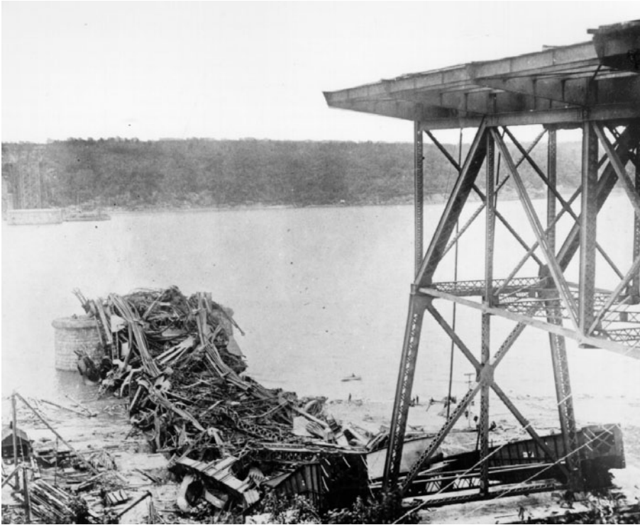
FIGURE 1.12 Wreckage of south anchor span of first Quebec railway cantilever bridge, 1907. View looking north from south shore a few days after the collapse on 29 August 1907, the worst disaster in the history of bridge construction. About 20,000 tons of steelwork fell into the St. Lawrence River, and 75 workmen lost their lives.
