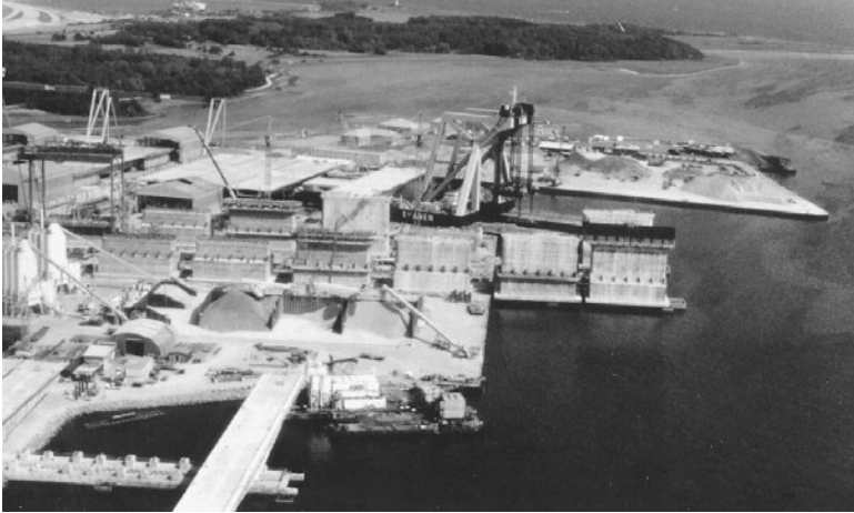
FIGURE 3.21 Prefabrication of box caisson piers for Great Belt Western Bridge, Denmark.
