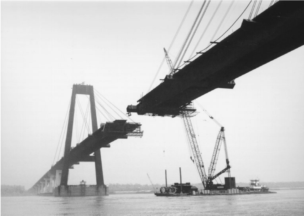
FIGURE 1.9 Cable-stayed orthotropic-steel-deck bridge over Mississippi River at Luling, La., 1982; view looking northeast. The main span is 1222 ft (372 m); the A-frame towers are 350 ft (107 m) high. A barge-mounted ringer derrick erected the main steelwork, using a 340 ft (104 m) boom with a 120 ft (37 m) jib to erect tower components weighing up to 183 tons, and using a shorter boom for deck components. Cable stays at the ends of projecting cross girders are permanent; others are temporary erection stays. Girder section 16-west of north portion of bridge, erected a few days previously, is projecting at left; companion girder section 16-east is on barge ready for erection (see Figure 1.10 ).
