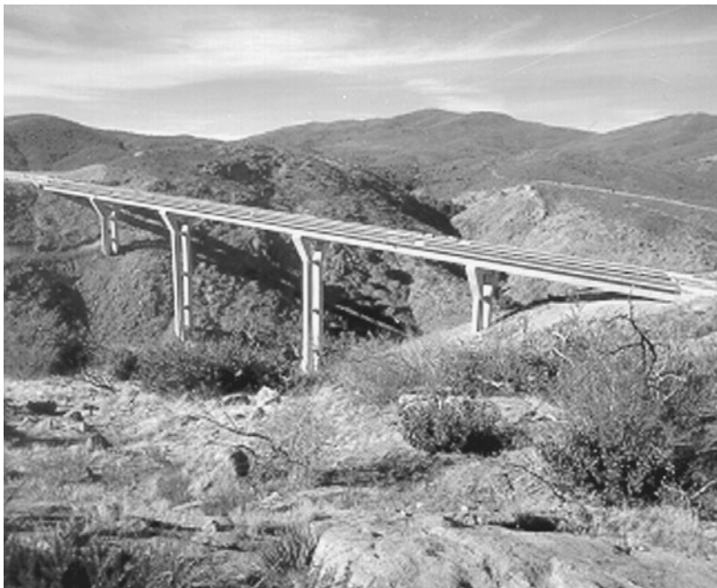
FIGURE 2.5 Pine Valley Creek Bridge — construction completion.
