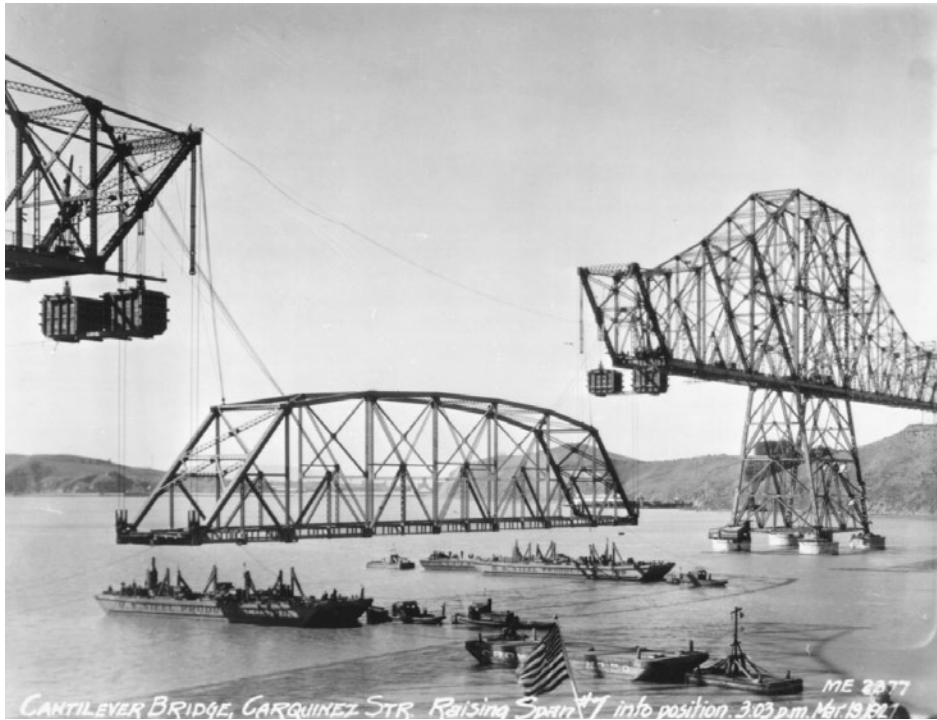
FIGURE 1.20 Raising of suspended span, Carquinez Strait Bridge, California, 1927. The 433 ft (132 m) suspended span, weighting 650 tons, was raised into position in 35 min., driven by four counterweight boxes having a total weight of 740 tons.
