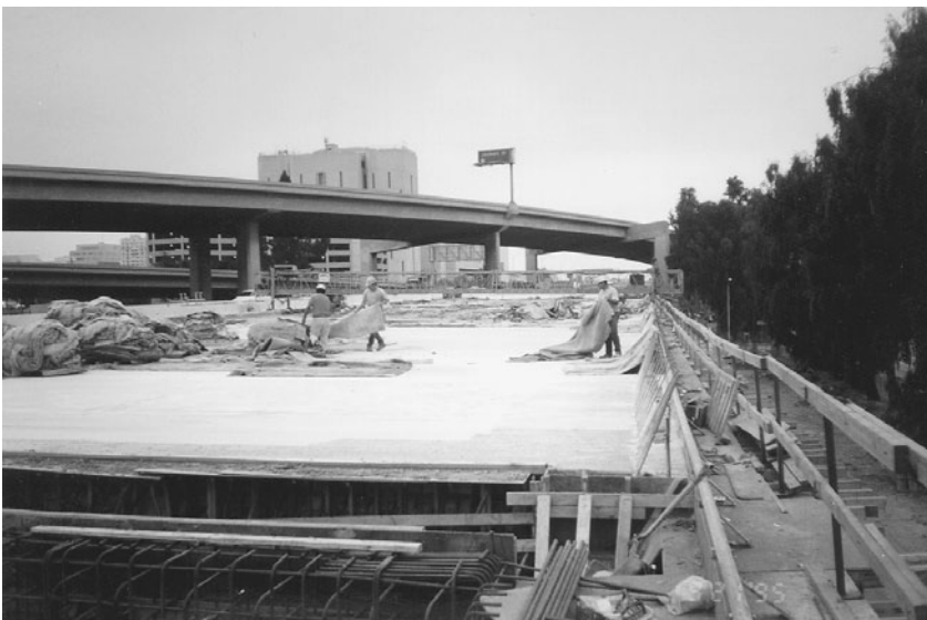
FIGURE 4.9 Bridge deck is being cured with moist rugs.
