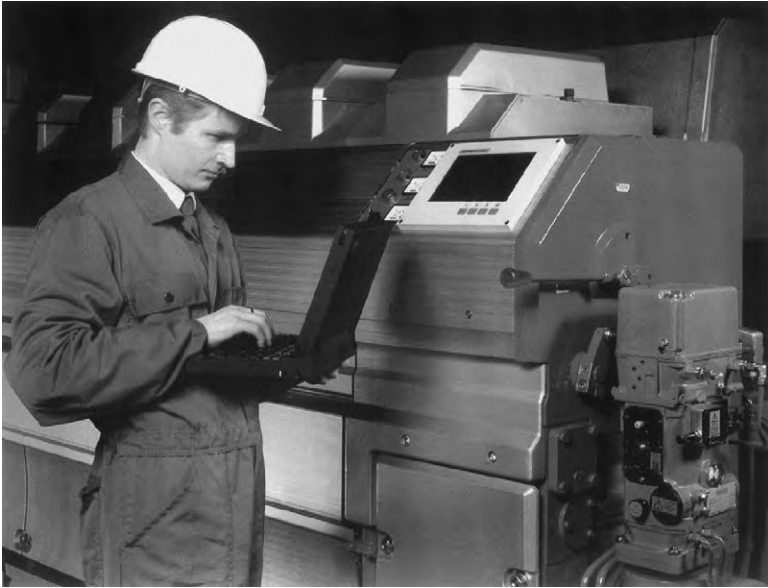
FIGURE 27.3 The engine computer is the ‘brain’ of the Wärtsilä Engine Control System (WECS), shown here on a Wärtsilä 32
