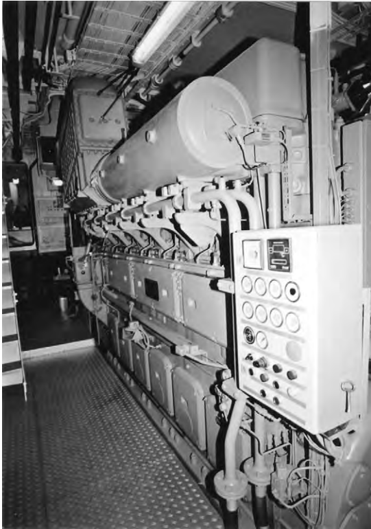
FIGURE 20.2 Deutz 645F engine installed in a Dutch trawler
