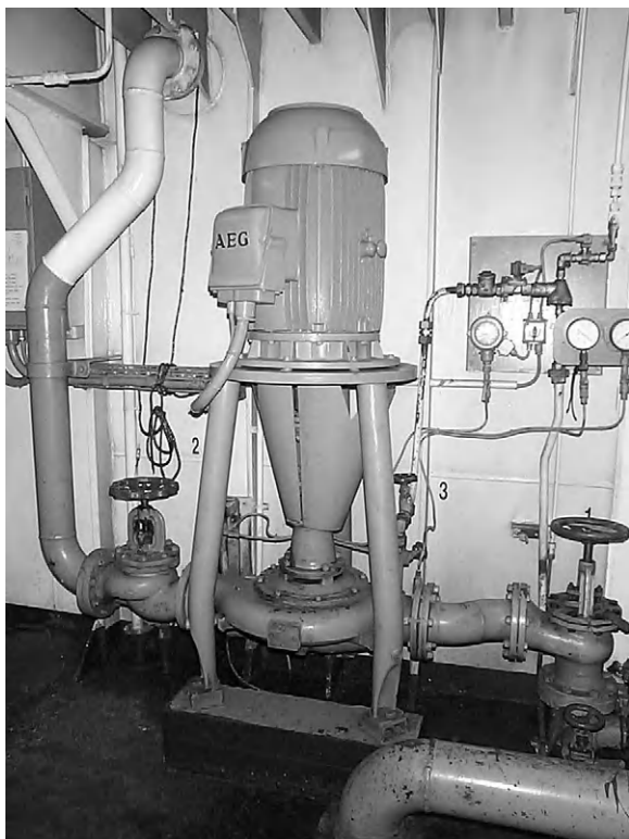
Figure 5.4 A vertical electric-driven centrifugal water pump
