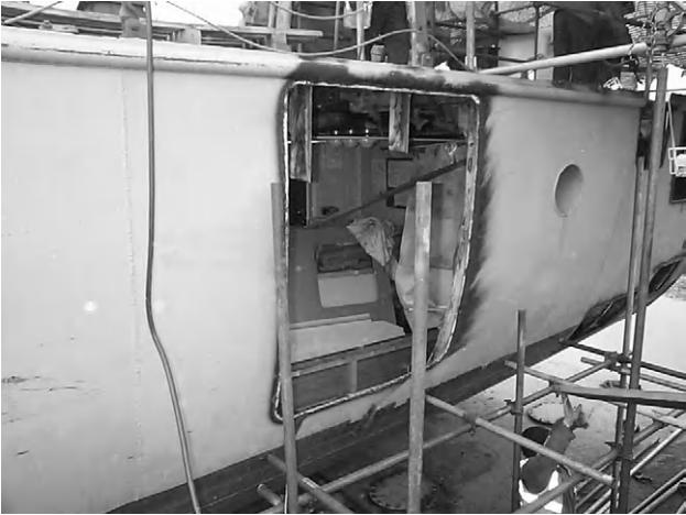
Figure 3.1 Repair of damage to shell plating
