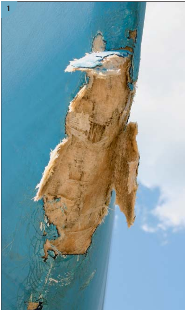
(1) The boat has been hauled after grounding on rocks, and here we're looking up at damage in the bow area. Impact damage has penetrated the outer laminate and into the core, which has been exposed in places.
