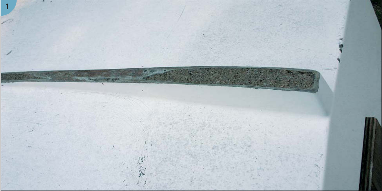
(1) This dinghy has been dragged repeatedly over a beach or other hard surface, wearing the skeg away. The core material in the skegs of many small boats is not glassed in place, so a breach in the exterior laminate may cause the
