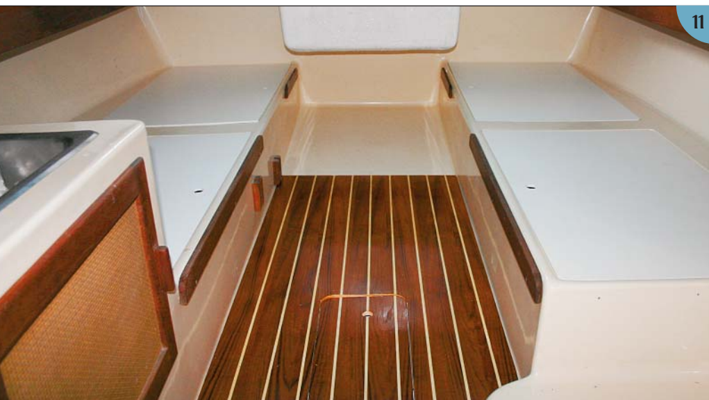
(11) The final job was to cut a teak-and-holly sole from plywood and place it on the new floor bearers. We screwed the sole to the old fiberglass liner around the edges. Measuring and cutting the sole took several hours. We coated it with Ultimate Sole, a high-gloss, varnish-style finish with low skid properties ( www.ultimatesole.com ). This product looks just like varnish but is much less slippery when wet. Compare this to photo 3 on page 21—it is the same boat.
