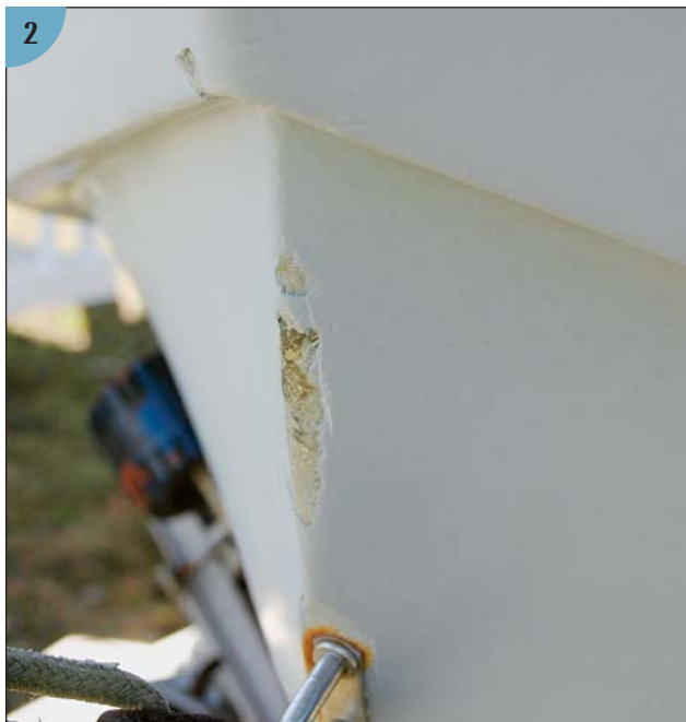
(2) Here we see chipping on the stem as well as the chine, possibly sustained in the same incident.
