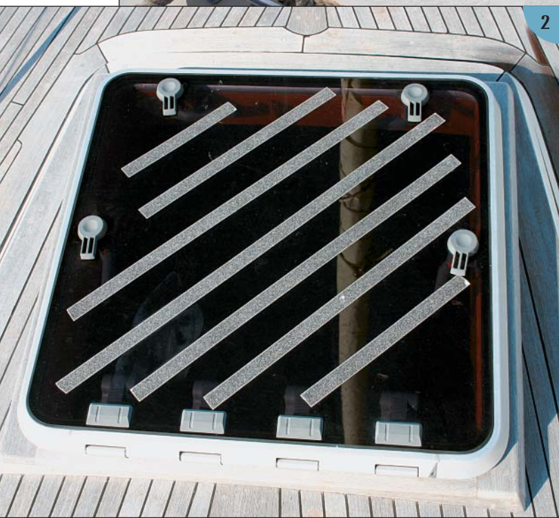
Nonskid tape can be used in many places to help prevent slips and falls. (1) On the foredeck of a launch it provides more secure footing for a crewmember tending lines. (2) On a foredeck hatch it transforms a slick surface to a “sticky” one.
