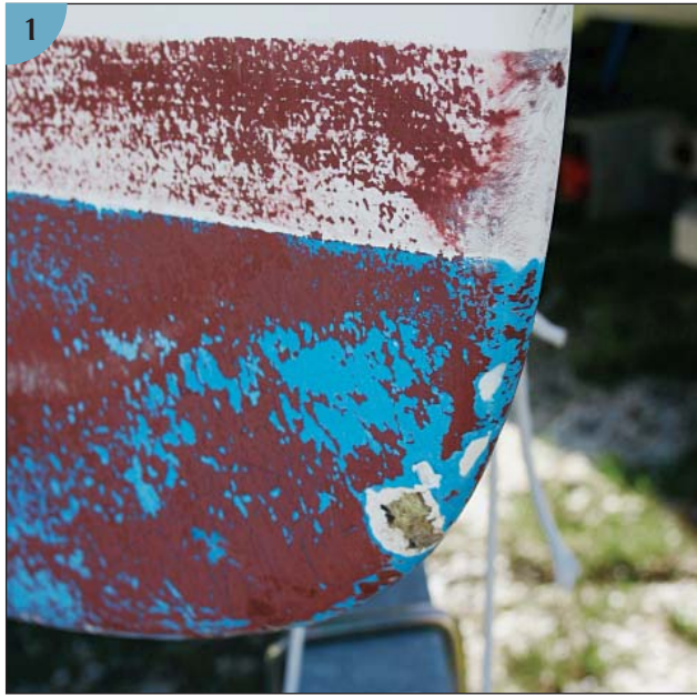
(1) Damage to a bow is not always obvious. This ding, probably caused by hitting a floating object, is below the waterline and should be repaired before the boat goes back into the water. If left like this, with the gelcoat missing, water can penetrate into the underlying laminate and/or the core. Impact damage along the chines of a powerboat may not be structurally significant, but it can be unsightly and can affect the boat's value when sold. Severe impact damage needs immediate repair.
