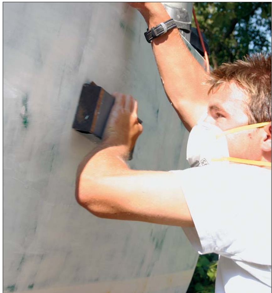
Doing a final sanding of primed topsides with a wood block and 400-grit sandpaper. The hull has already been machine sanded with 320-grit. Once this sanding is done, the topsides will be ready for the polyurethane topcoat.
